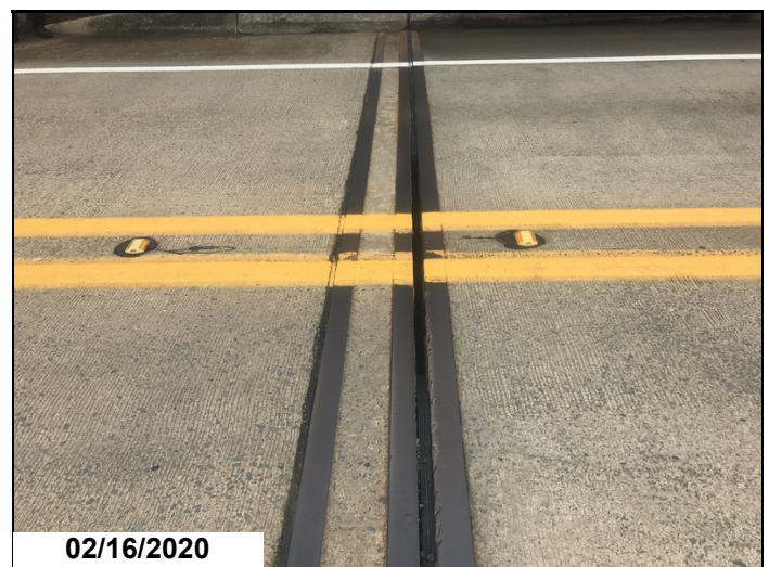
Bt. 1, 6' of joint seal missing.
