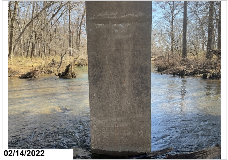
Cracks at bent 4 and 5
