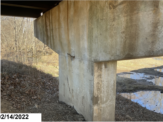
Spall with rebar at bent 6
