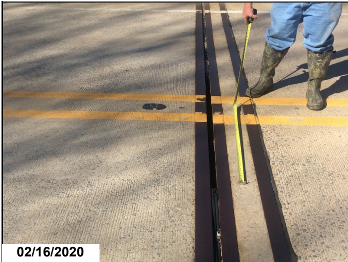
Bent 1 abutment has 5 foot of joint seal missing
