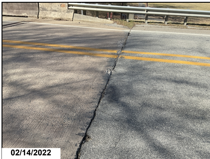
Spall at bent 1 approach slab
