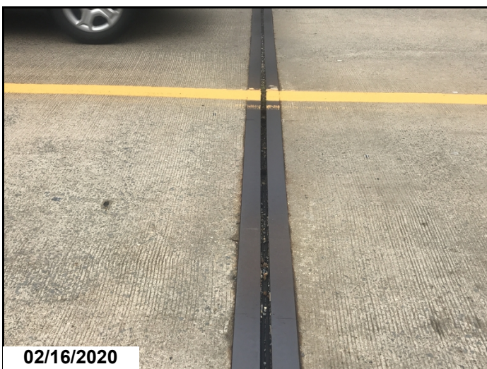
Bt. 3, 3' of joint seal missing & debris impacted.
