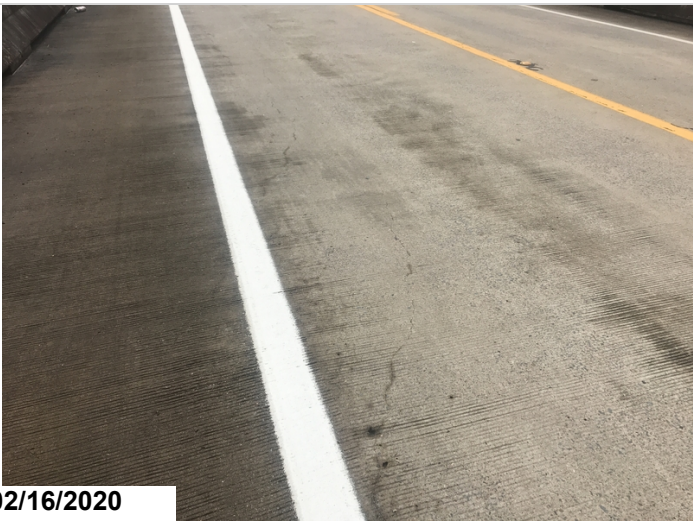
Span 2, cracks up to 0.020"
