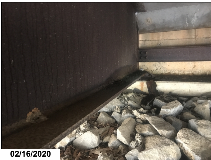
Bt. 7, Beam 4, active corrosion
