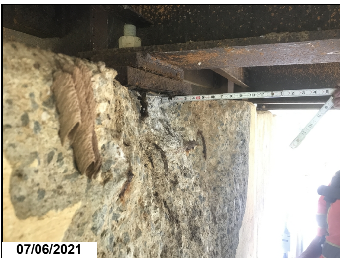
1 1/4 " loss of bearing area at the masonry plate at bent 4 backside
