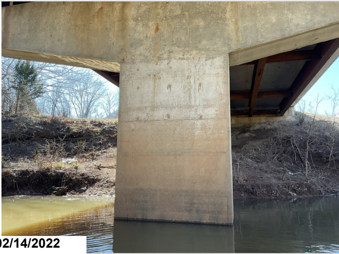
Bent 5 backside has large cracks and delamination
