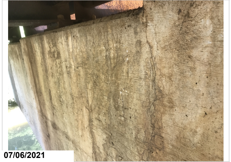
longitudinal and vertical cracks and cracks with rust staining
