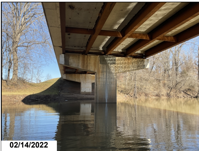
Bent 3 repair has been made to large spall under beam 3
