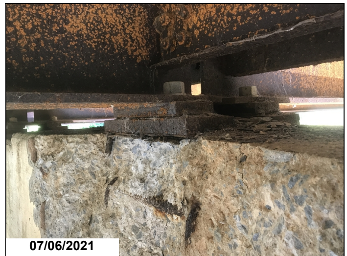
4' spall with rebar exposed at bent 4 backside
