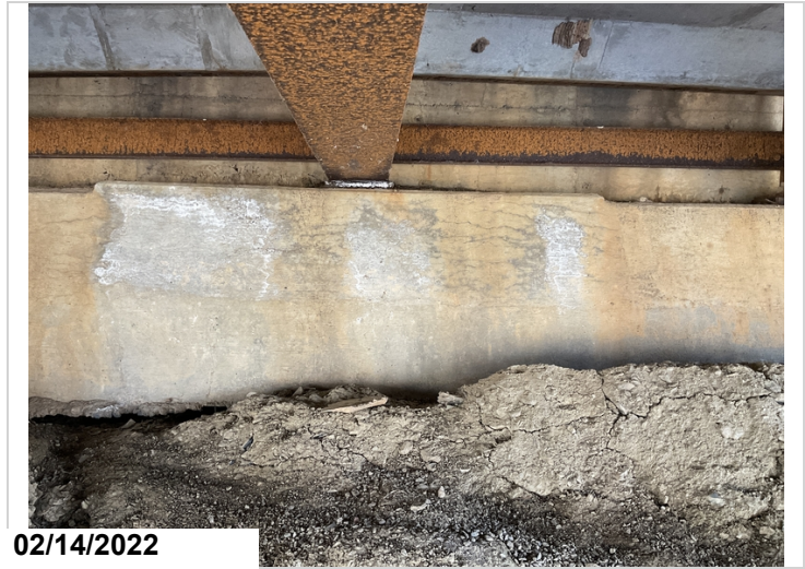
Map cracks in the abutment at bent 6
