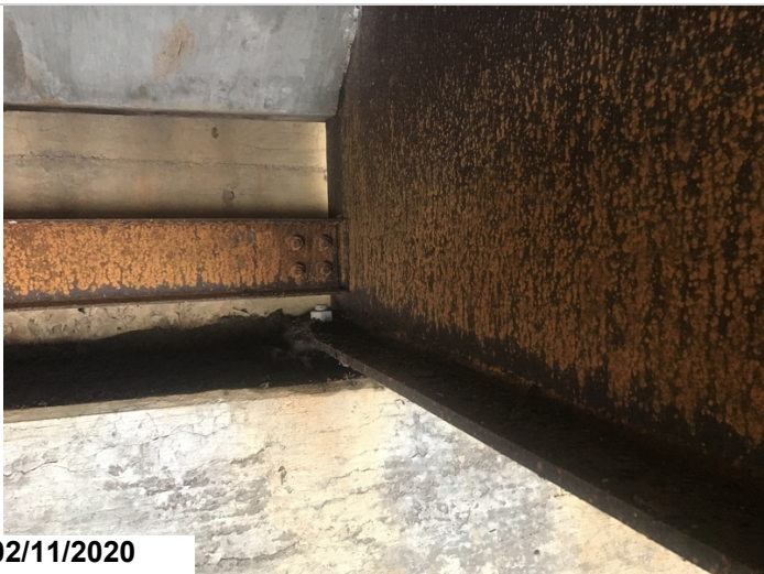
Bt. 6, Bm. 3, bottom flange & web around hothead haunch has corrosion.
