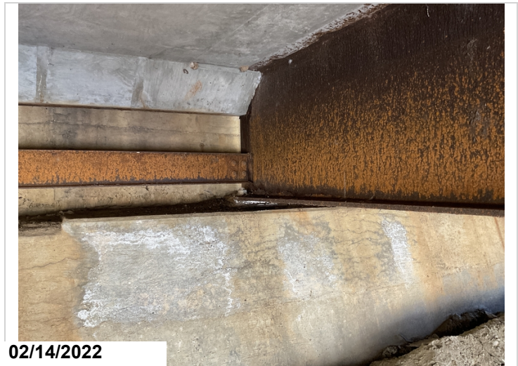
Bent 6 girder 3 bearing has corrosion and laminated rust
