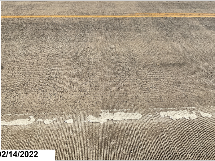
Deck cracks in span 5
