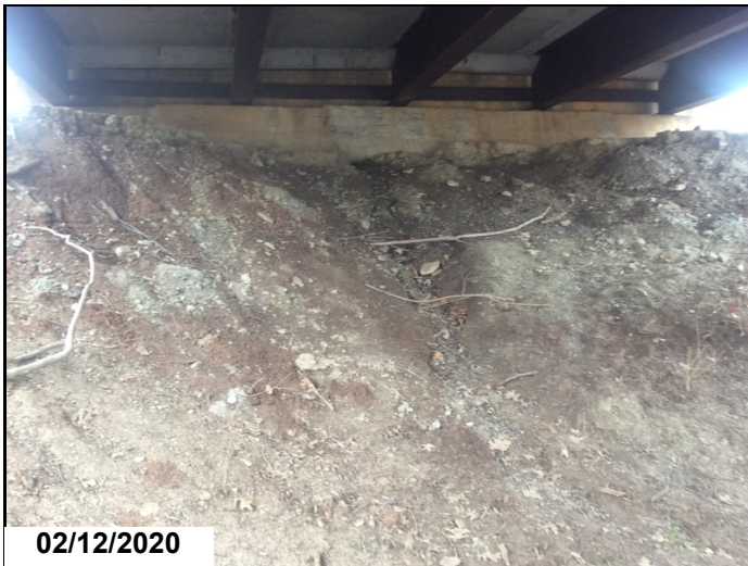
Embankment at Bent 6 (South end) has settled
