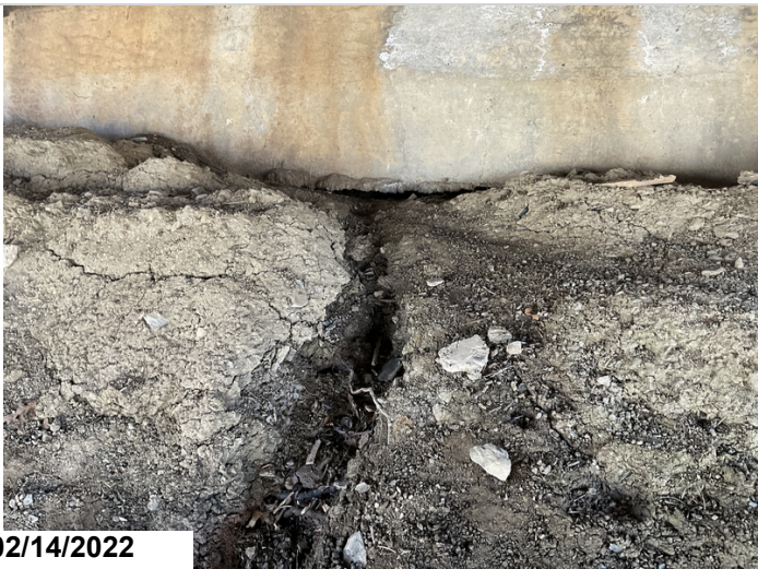
Erosion at bent 6 between girder 2 and 3
