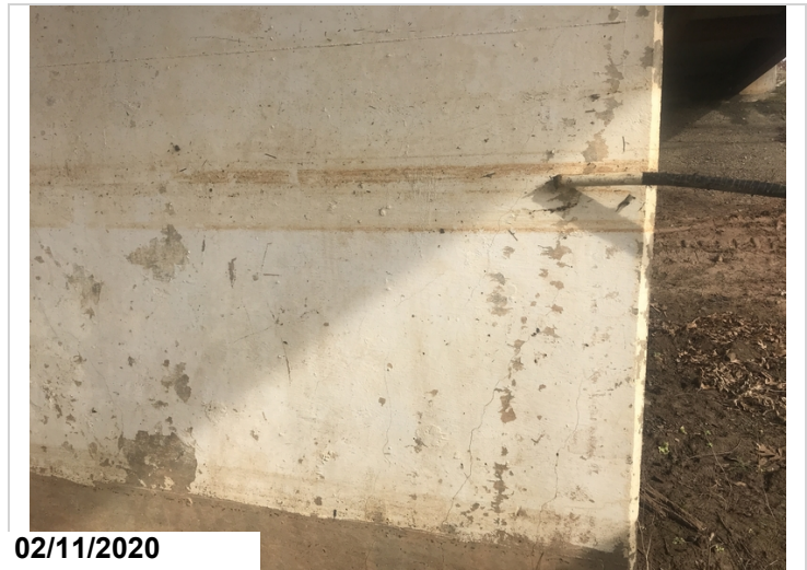
Bt. 2 column, cracks up to 0.015"
