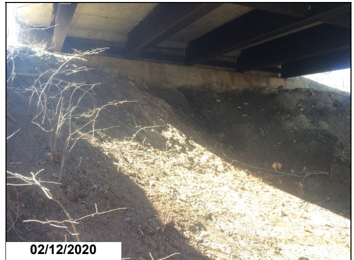
Looking at bent 6: runoff is eroding the embankment.
