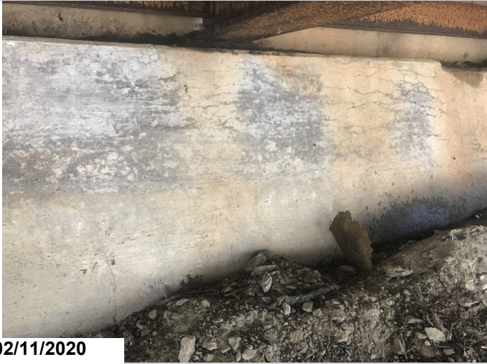
Bt. 6 abutment has horizontal cracking.
