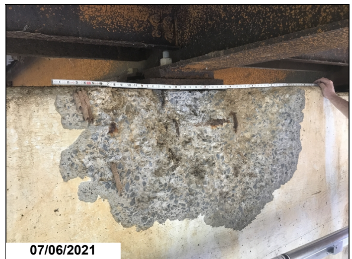
4' spall with rebar exposed at bent 4 backside
