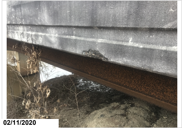
Span 5, right edge, spall.
