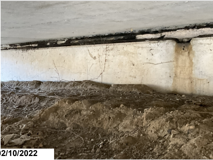
Horizontal crack at bent 1 abutment
