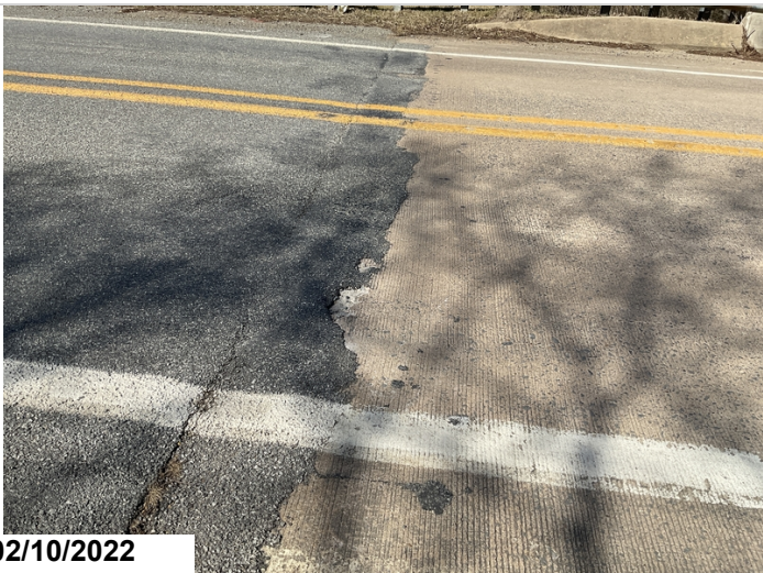
Small spall at east approach slab is half full of asphalt
