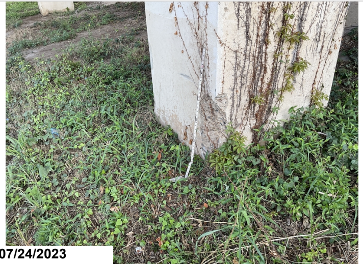
Bent 4, column 3: spall to the bottom of column. (1'4" x 11")
