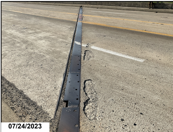
Span 2 , bent 2: multiple spalls adjacent to the joint. Approximately 20sf.
