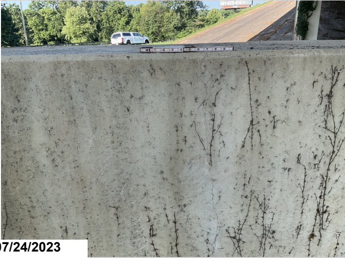
Bent 3: pier wall with couple full height vertical cracks up to 0.016"
