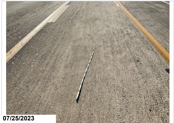
Span 4: multiple longitudinal cracks (0.025")
