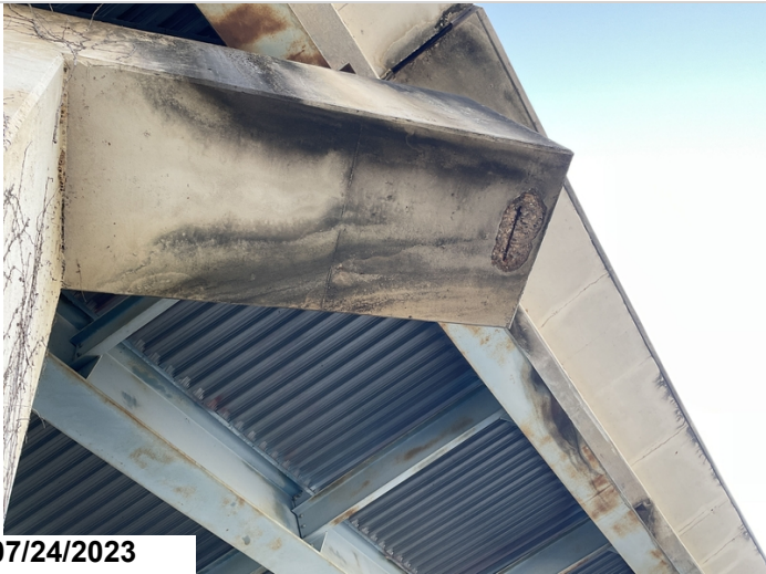
Bent 4: bottom of cap spalled with exposed rebar. (1'x8")
