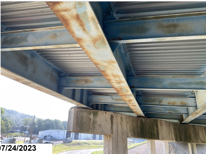
Span 1, girder 2: bottom flange with freckled rust. 2023
