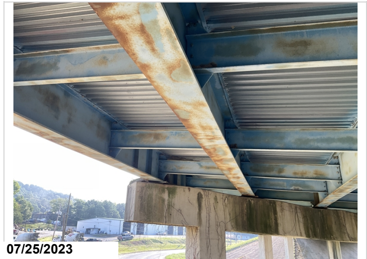
Span 1, girder 2: bottom flange with freckled rust. 2023
