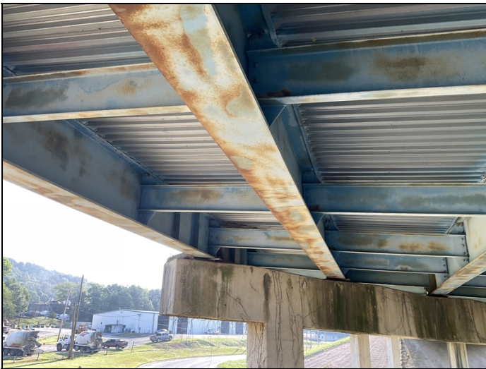
Span 1, girder 2: bottom flange with freckled rust. 2023
