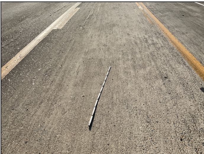
Span 4: multiple longitudinal cracks (0.025")
