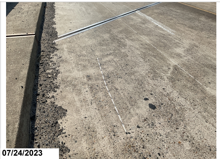
Span 3: large unsealed diagonal and transverse cracking. Average width is 0.030"
