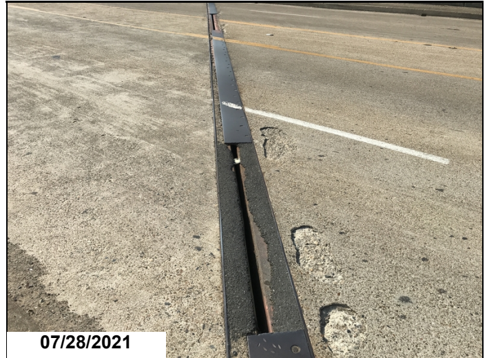
Bent 3 approx. 22 foot of joint armor missing.
