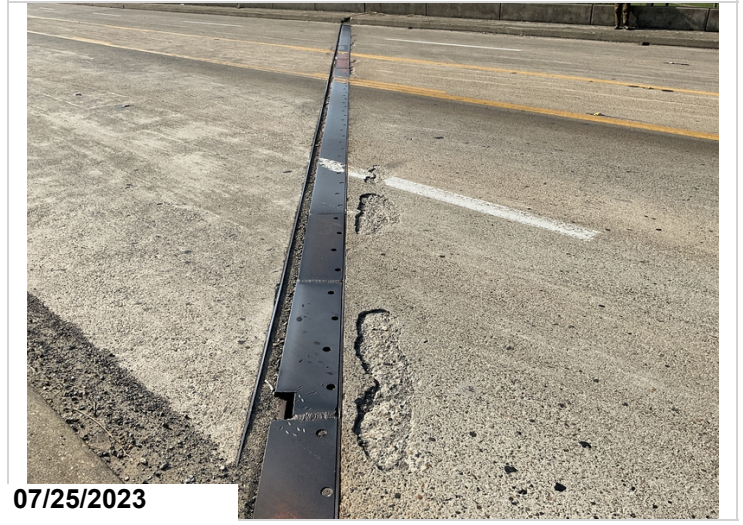
Span 2 , bent 2: multiple spalls adjacent to the joint. Approximately 20sf.
