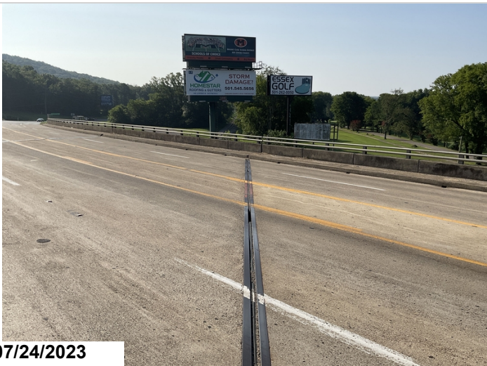
Bent 2: 5' of joint material missing or has lost bond allowing water to freely flow through.
