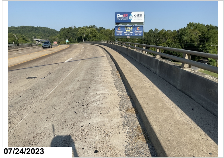
All spans with dirt and debris build up on the shoulders and sidewalk.
