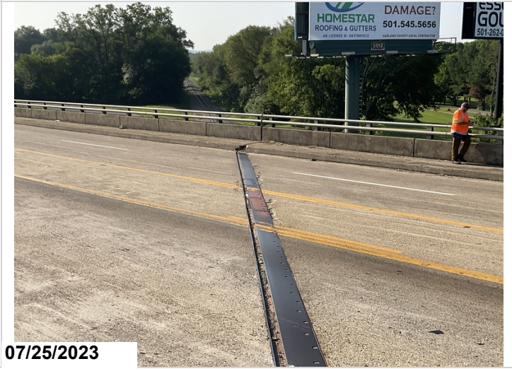
Bent 3: East bound lanes: the assembly joint is loose under traffic
