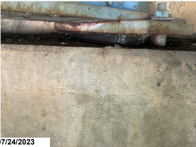
Bent 1, girder 6: active corrosion to all bearings is common throughout.
