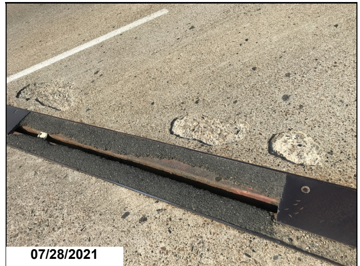
Deck span 2 at bent 3 has spalls.
