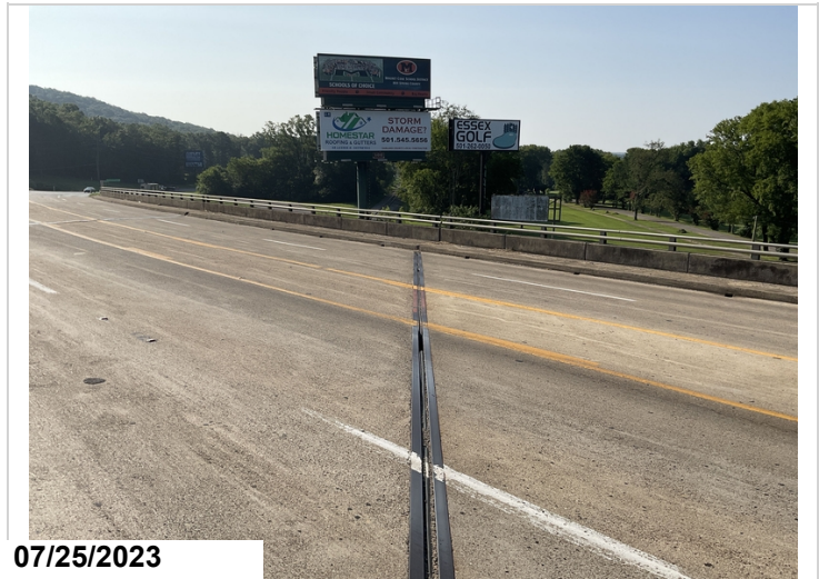
Bent 2: 5' of joint material missing or has lost bond allowing water to freely flow through.
