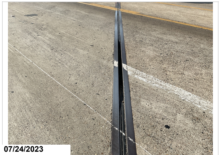
Bent 4: 5' of joint seal has lost it's bond and has dropped out.
