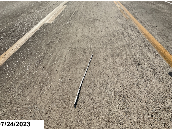
Span 4: multiple longitudinal cracks (0.025")
