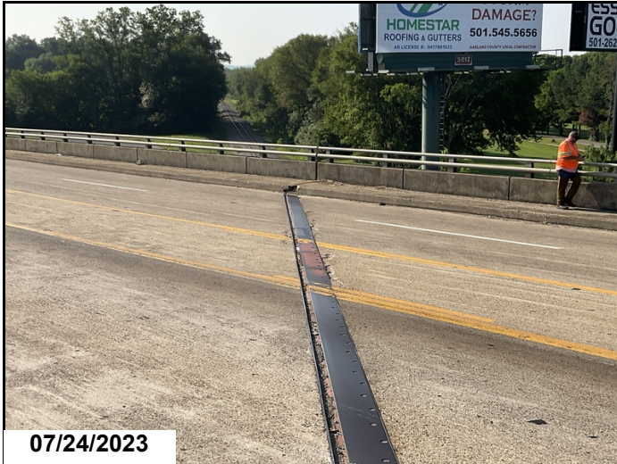
Bent 3: missing joint seal has been repaired.
