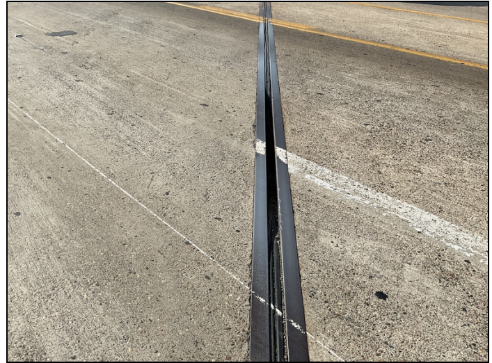
Bent 4: 5' of joint seal has lost it's bond and has dropped out.
