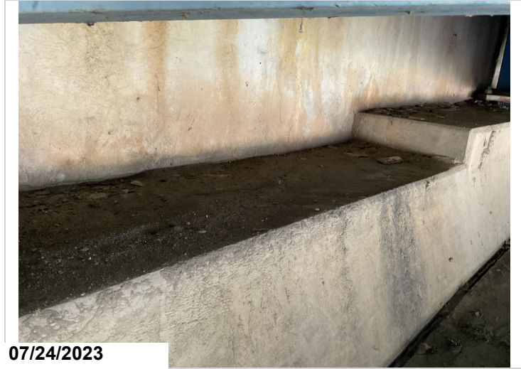
Bent 1: beam seat has dirt and debris
