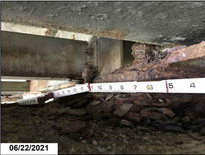
Ahead bent 21, span 22, beam 1: beam has severe section loss to the bottom flange at the bearing.
