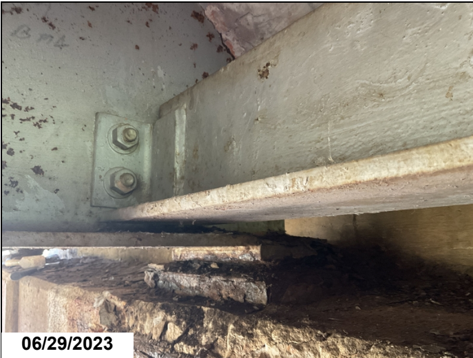
Abutment 1 span 1 beam 4, left bottom flange is down to a knives edge over bearing. 6" from beam end.
