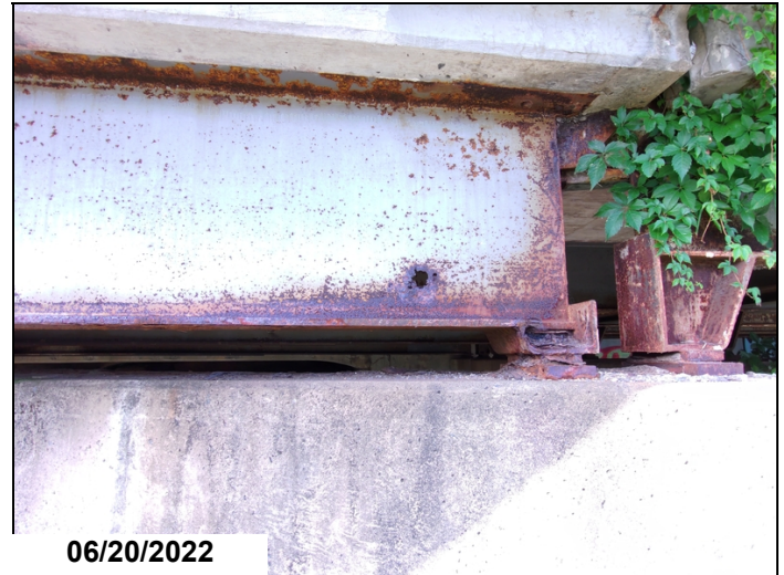
Bent 19, span 19, beam 5: large hole in web.2022
