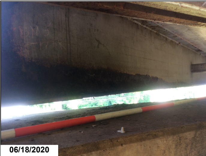
Bent 6 beam 3 holes in the upper and lower web
