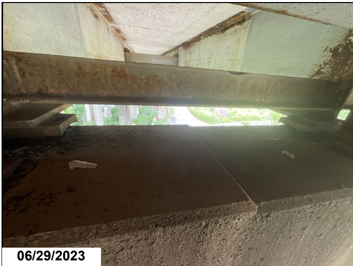
Span 10 at bent 9 anchor bolts missing
