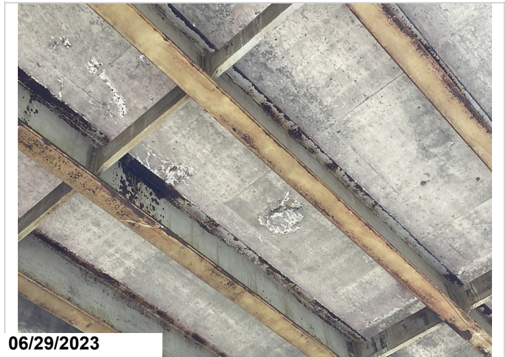
Span 10 exposed rebar on soffit
