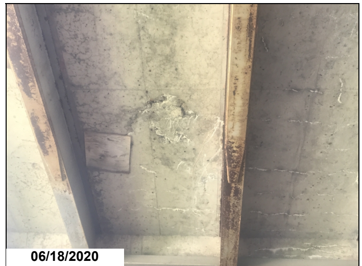
Span 3 soffit between beams 3 & 4 delam.
