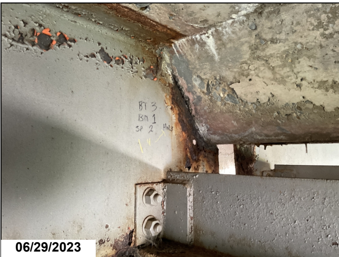
Bent 2, span 2, beam 1: 1" Hole in the web at the haunch.
