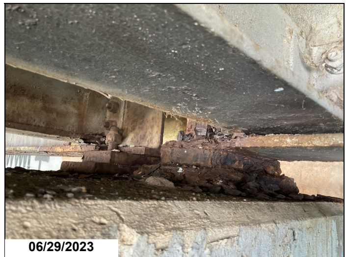
Ahead bent 21, span 22, beam 1: beam has severe section loss to the right bottom flange at the bearing.
