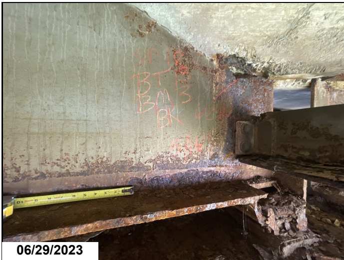
Span 18, bent 18, beam 3: 6"x2" hole in haunch area. 5/16" section loss in lower web.
