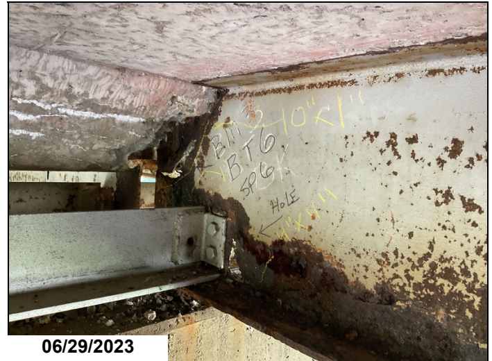
Bent 6, span 6, beam 3: 10"x1" holes in the web at the haunch where it nearly goes to the end of the girder and lower web just back from the diaphragm. 4"x4" hole in lower web in front of diaphragm. 1" hole behind diaphragm. 1/2" section loss to left side of bottom flange 1" in front of bearing.
