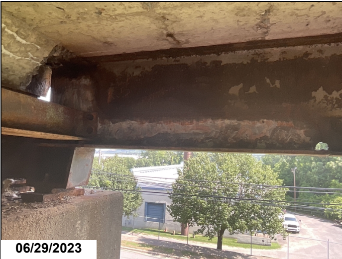
Bent 16 span 16 beam 5 t-splice repair 2023
