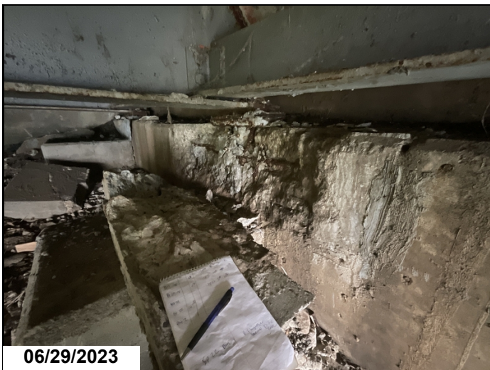
Abutment 2, spall 50% bearing loss area
