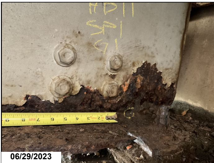
Abutment 1 span 1 beam 1, 8" of left side of bottom flange has 100%. 1/2" hole in lower web 6" from beam end. Right bottom flange has 75% section loss over bearing
