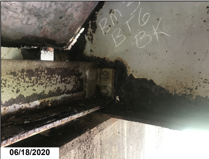
Bent 6 beam 3 holes in the upper and lower web
