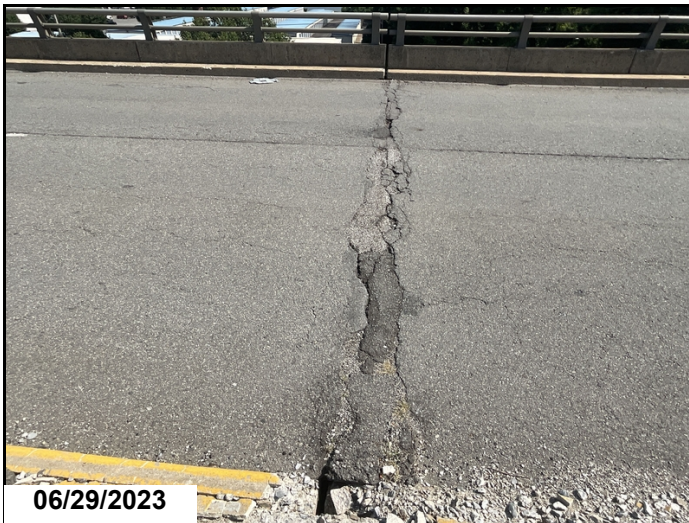
Most joints have spalls in asphalt overlay
