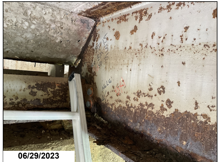
Span 15, bent 15, beam 3: 5"x1" hole in haunch and lower web.
