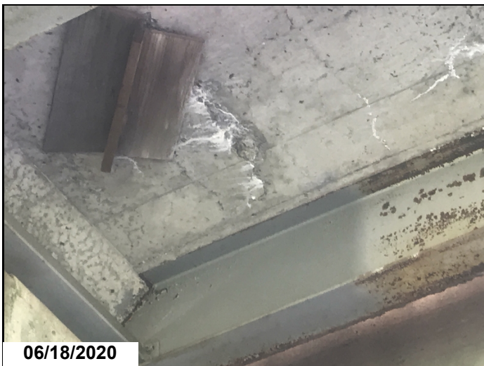
Span 6 soffit between beams 1 & 2 delam.
