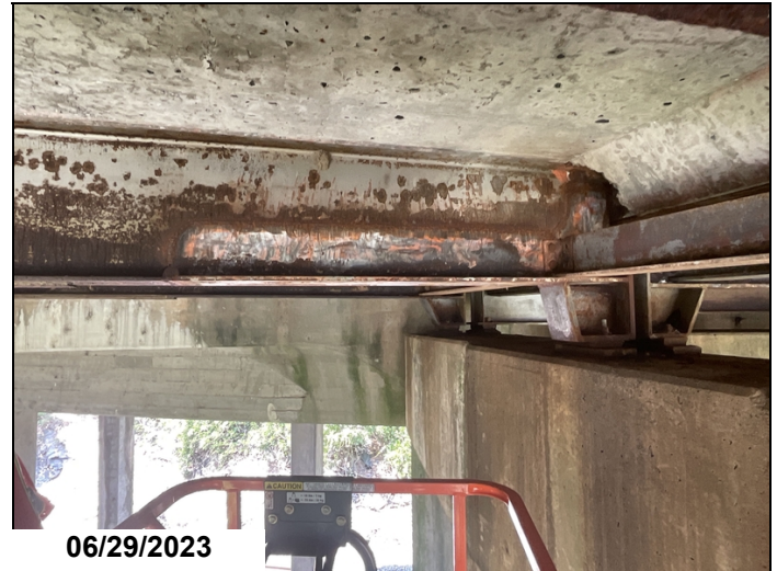
Bent 16 span 16 beam 2, t-splice repair 2023
