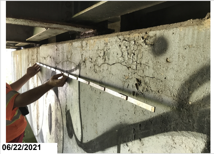
Ahead side of bent 21: large horizontal crack runs along the entire face. (Approximately up to 1/8" in width.)
