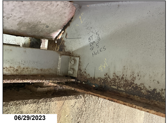
Bent 5, span 5, beam 3: section loss at the beam end with 8"x1" hole in lower web 12" from beam end and 5"x1" hole in haunch
