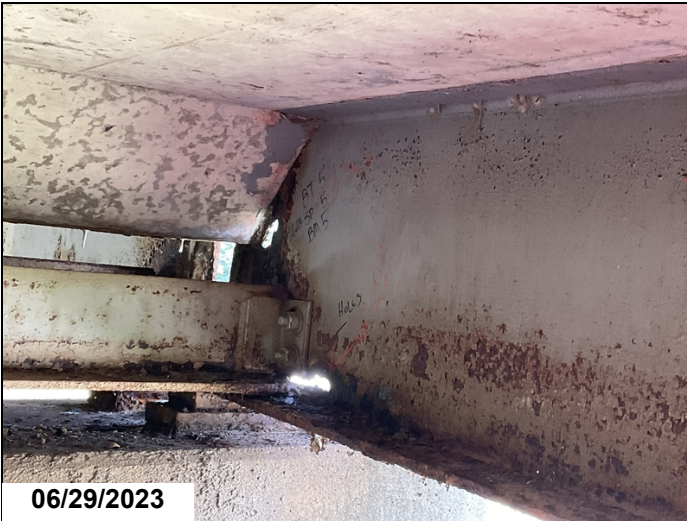
Bent 5, span 5, beam 5: section loss at the beam end with 6"x2" hole in lower web 12" from beam end and 3"x2" hole in haunch
