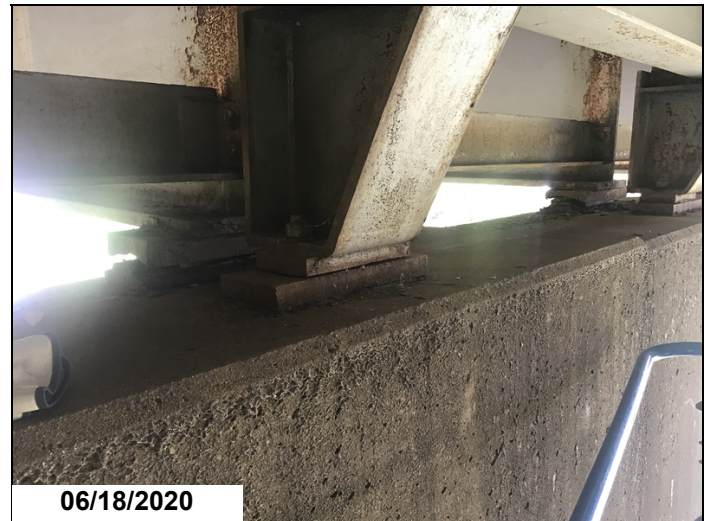
Bent 9 bearing at beams 2 & 3 ahead missing anchor bolts.
