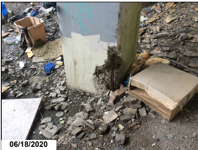
Bent 16 column 1 spall with exposed rebar.
