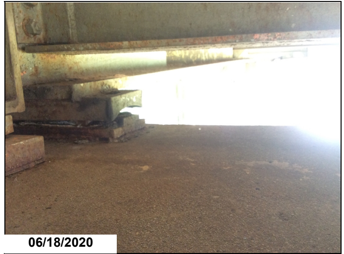
Bent 9 bearings on the ahead side have both anchor bolts rusted out on all five girders. This is typical at bents 10-12 also.
