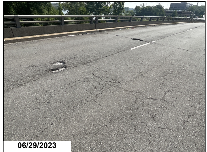
Spalls in asphalt overlay
