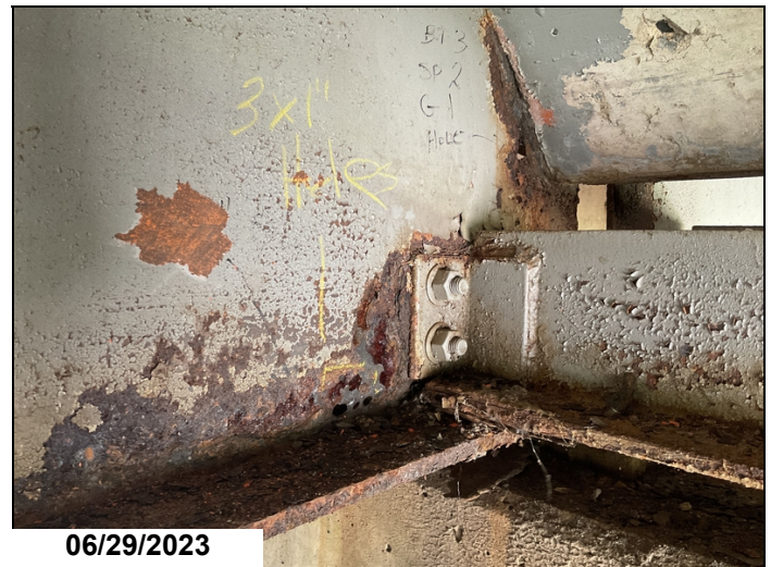
Bent 3, span 2, beam 1: 1-1/2" hole in the web at the haunch. 3"x1" hole in lower web
