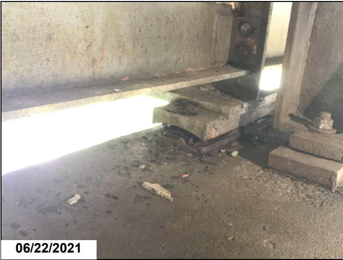
Bent 9, span 10, beam 2: bearing is missing anchor bolts. Common to all moveable bearings at this bent
