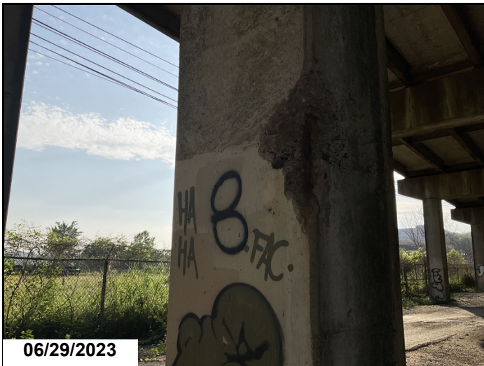
Bent 8 column 1 spall with exposed rebar
