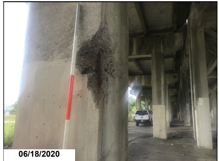
Bent 8 column 2 spall with exposed rebar.
