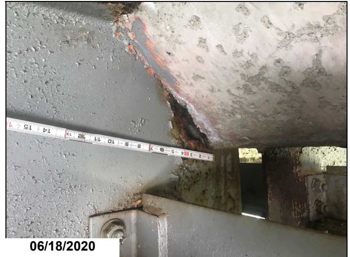
Bent 5 beam 2 back hole in the web.
