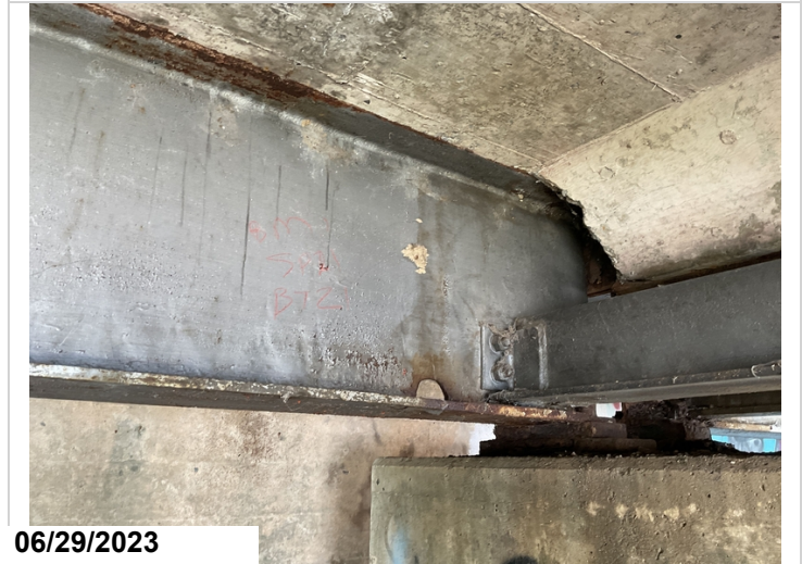
Span 21 beam 1 at bent 21 t-splice repair
