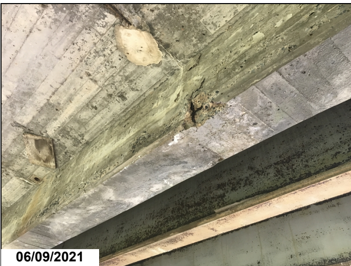
Span 13, girder 5: spall with exposed rebar.
