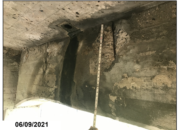
Span 7, girder 1 with multiple spalls with exposed rebar.
