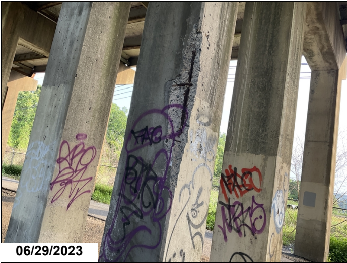
Bent 7 column 3 large spall with exposed rebar
