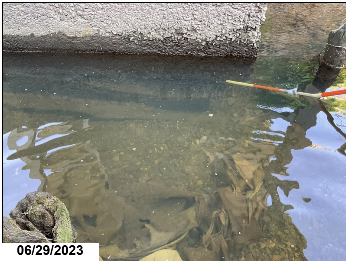
Bent 16 footing is undermined 2' on downstream end
