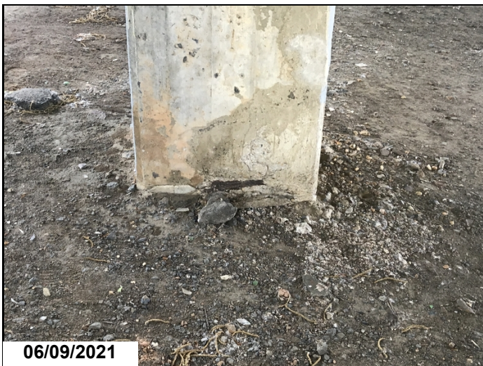
Bent 4, column 2: spall with exposed rebar.
