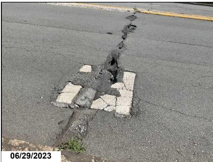
Bent 6 spalls in asphalt overlay at joint
