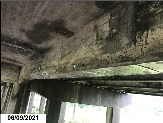
Span 6, girder 5: multiple cracks with efflorescence build up and small spalls.
