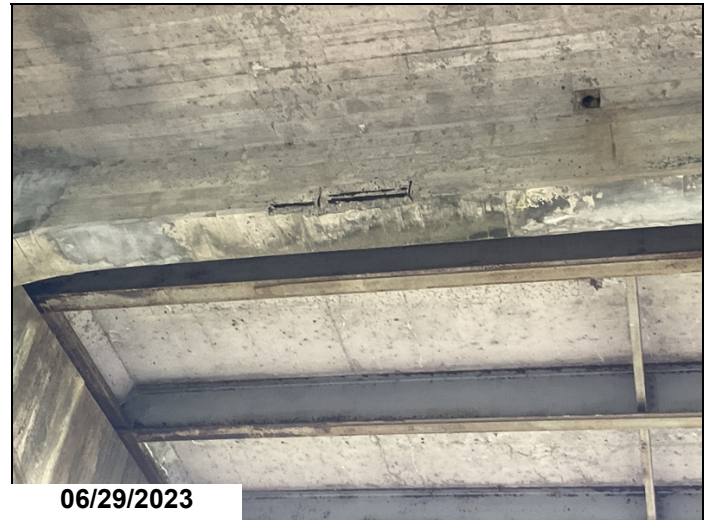
Span 8 girder 4 spall with exposed rebar on left side
