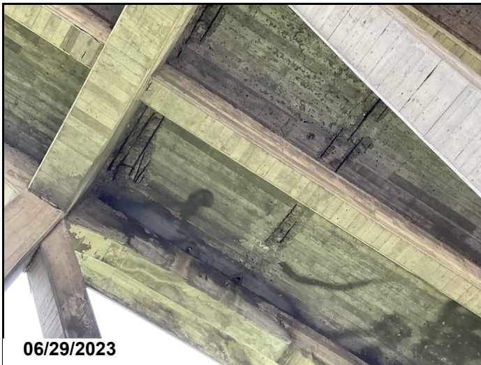
Span 13 exposed rebar on soffit
