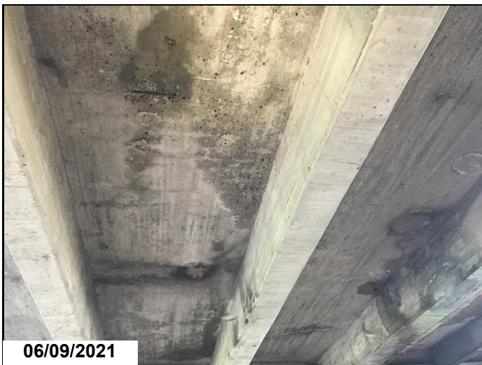
Span 3 has spalls with exposed rebar and multiple cracks with efflorescence staining.
