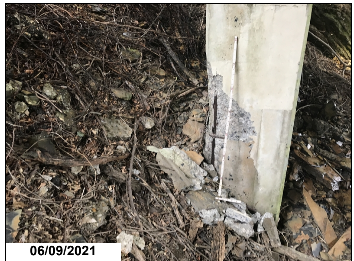
Bent 25, column 1: large spall with exposed rebar that has section loss.
