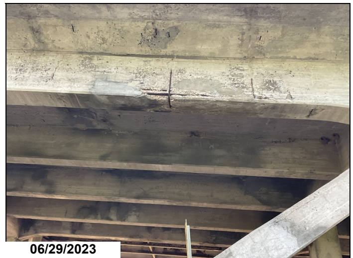
Span 5 girder 1 left side has spall with exposed rebar.
