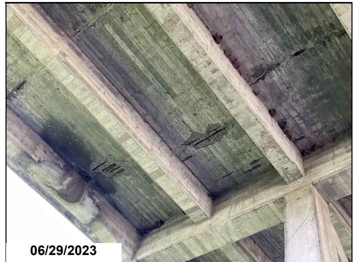
Span 14 exposed rebar on soffit
