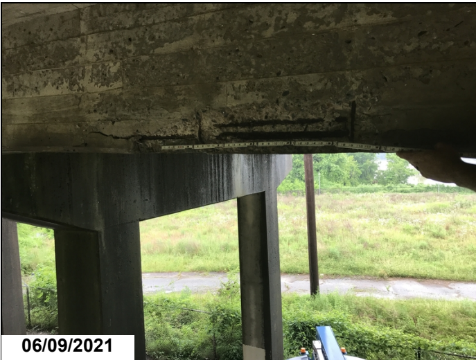
Span 8, girder 3: large spall with exposed rebar. There are 10' of delam on this girder also.
