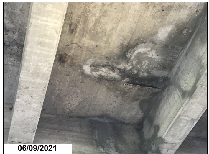
Span 5, between girders 2 and 3: large delam and spall with exposed rebar.
