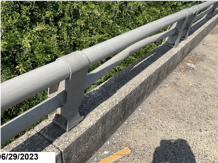
Span 25 damage to metal rail
