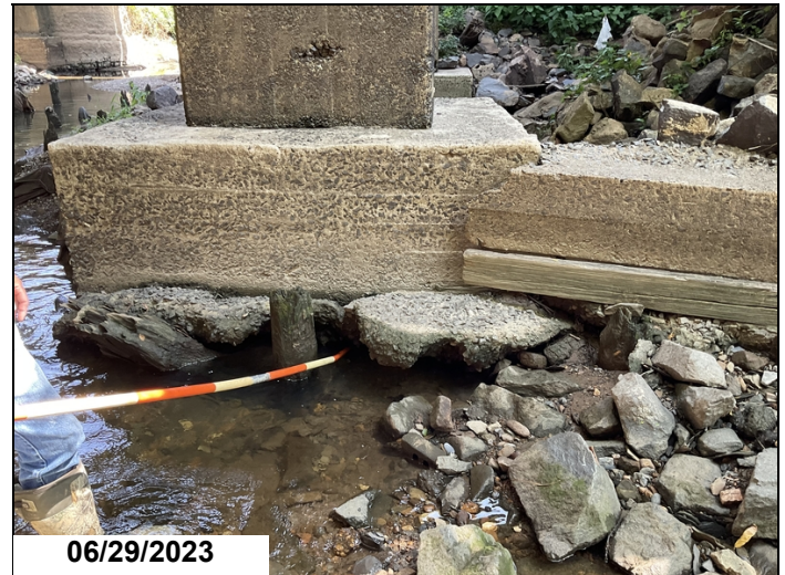
Bent 15 footing is undermined 1' on upstream end
