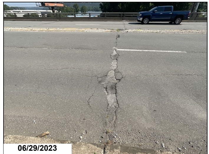
Bent 19 spalls in asphalt overlay at joint
