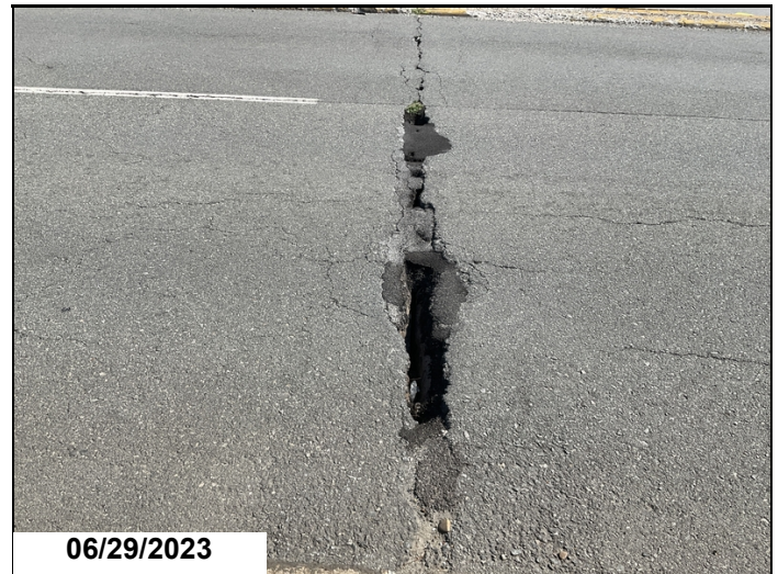
Bent 13 spalls in asphalt overlay at joint
