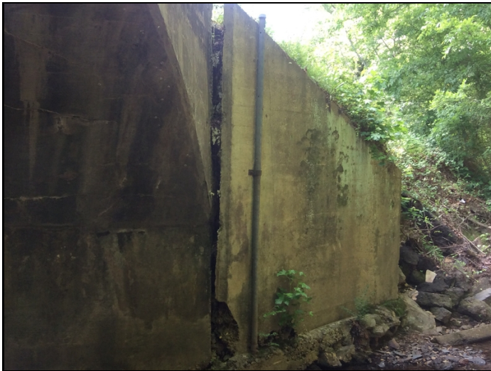
South end of bridge left wing wall has settled and separated from bridge.
