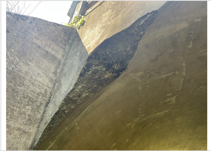
Spall on right side of arch.
