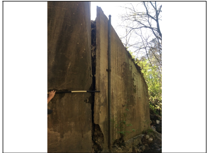
Southwest wing wall leaning on at top six inches.
