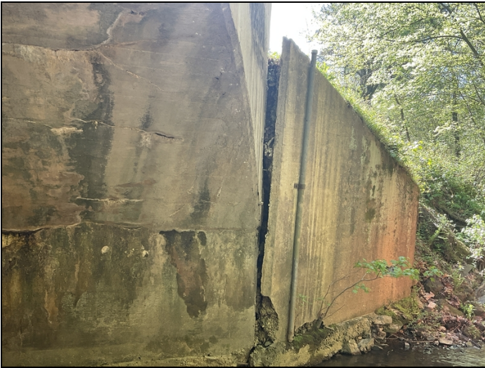
Southwest wing wall leaning on at top six inches. The gap is up to 6 3/4" as of 2022 no change.
