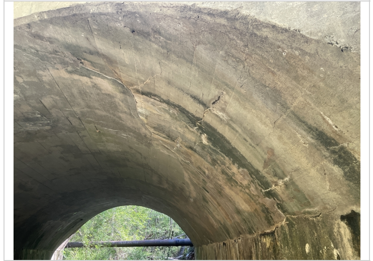
Cracks with efflorescence in the arch.
