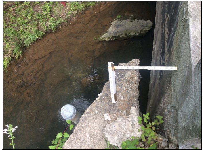
The southwest wing wall has a 6 3/4" gap, leaning away from the bridge at the top.
