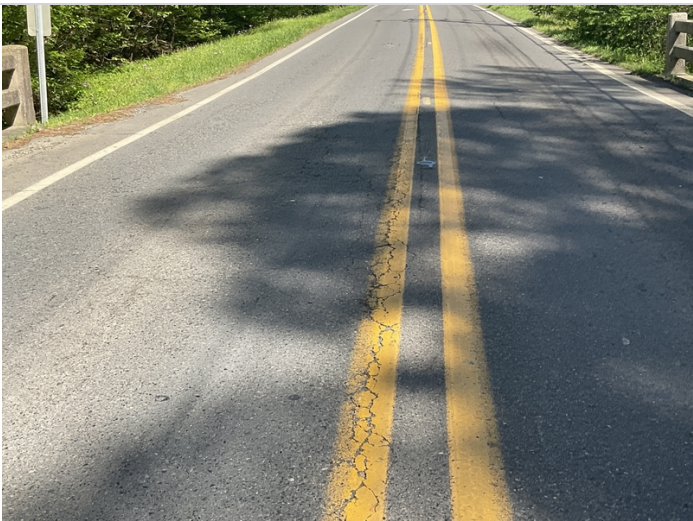
Cracks in the wearing surface.
