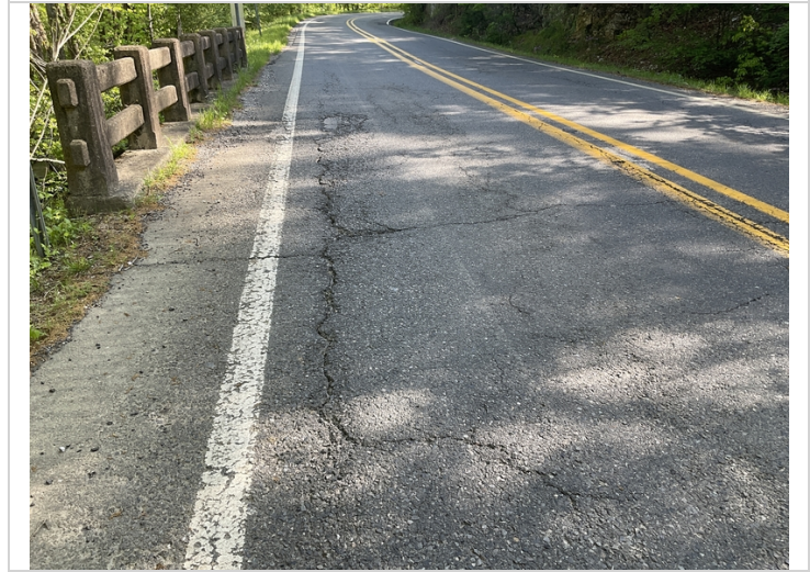
Large cracks in asphalt wearing surface.
