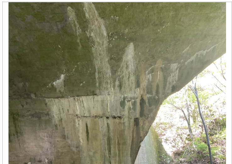
Cracks with efflorescence in the soffit of arch.
