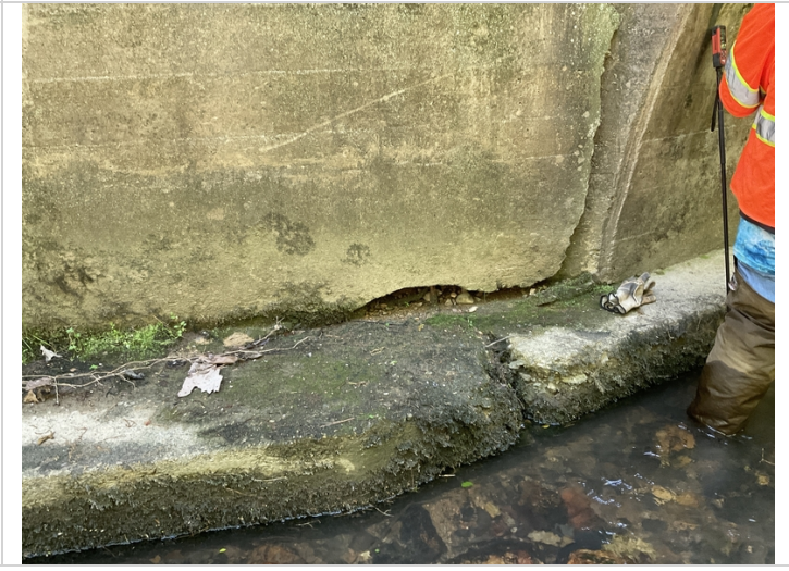
Abrasion left side abutment 2 wing wall
