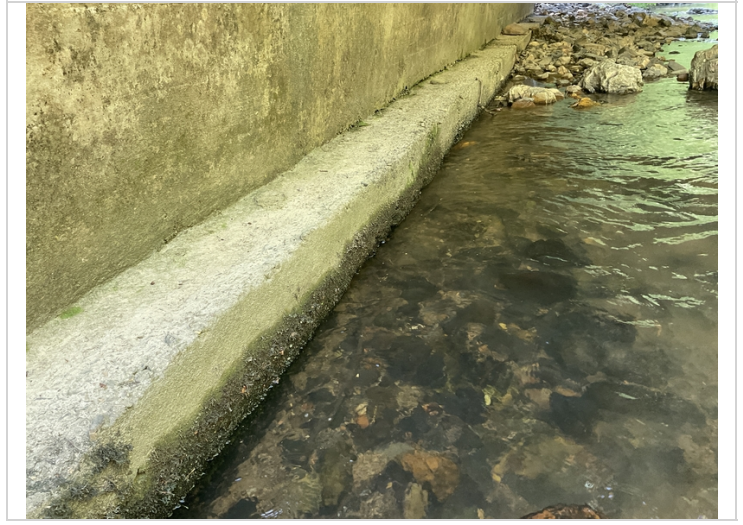
Abrasion bent 2 footing.
