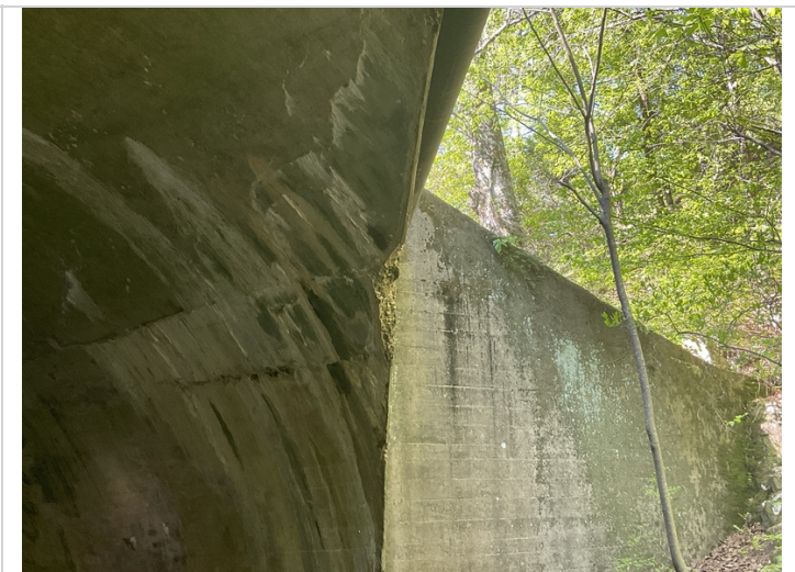
Spall on left side of arch.
