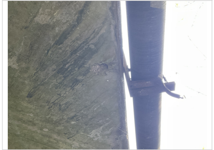
Spall with exposed rebar on right side on arch.
