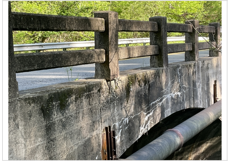
Right rail has exposed rebar.
