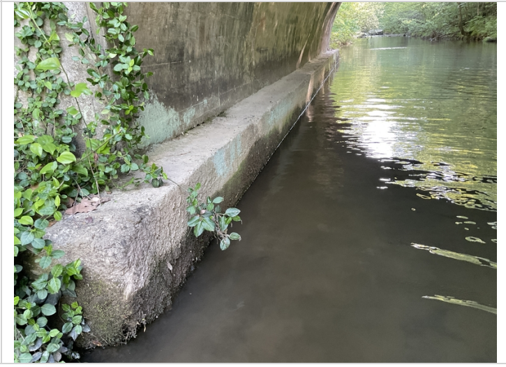
Exposed footing at abutment 2 with abrasion.
