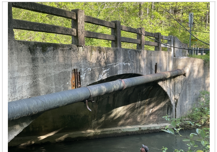
Cracks with efflorescence on right side of arch.
