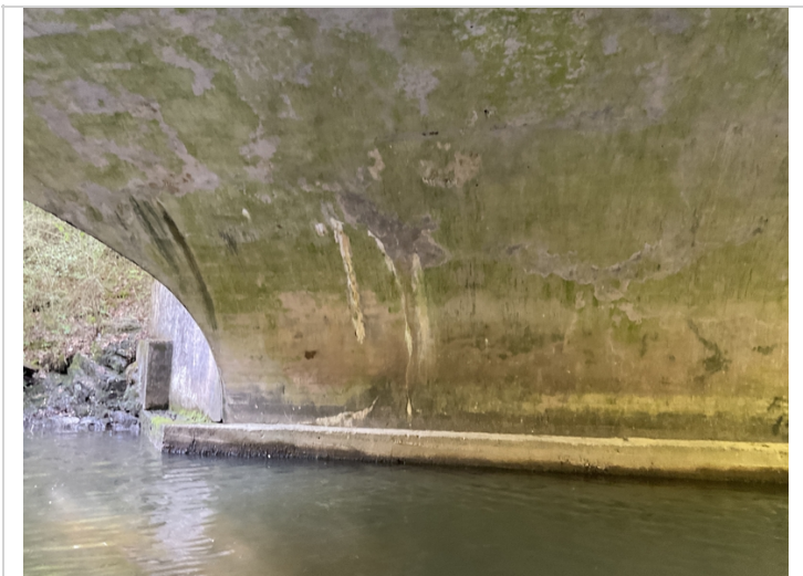
Cracks with efflorescence in the arch at abutment 1.
