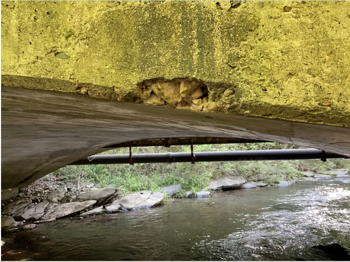
Spall on left side of arch.
