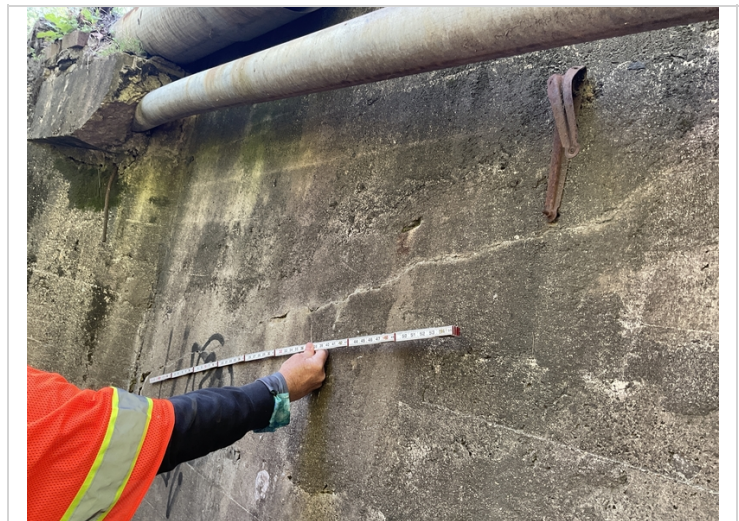
Bent 2 left side of arch crack.
