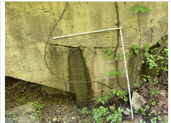
Crack in left side of arch.
