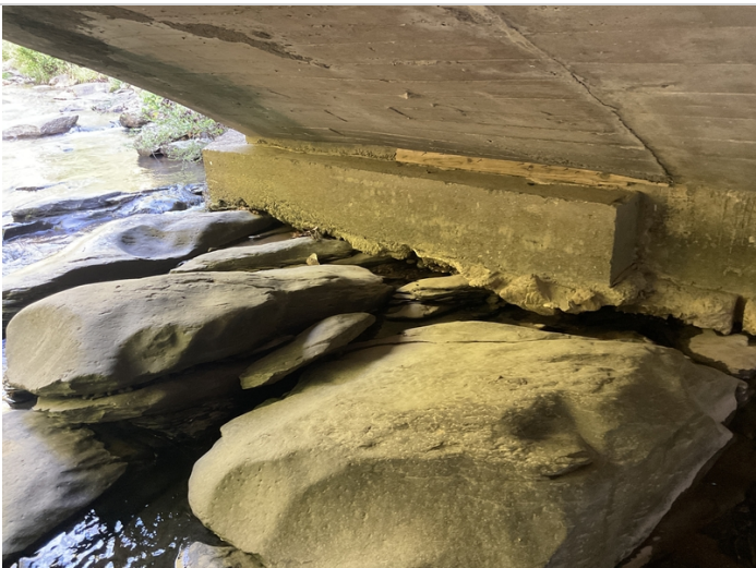
Bt. 2 has been undermined 6" but supported by solid rock formation.
