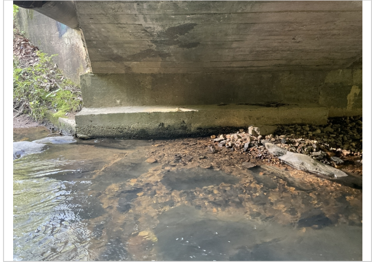
Bent 1 has 6' of abrasion on right end.
