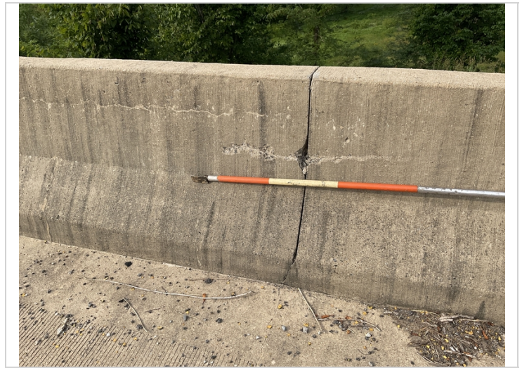
Contact spall in the bridge rail at bent 6 abutment
