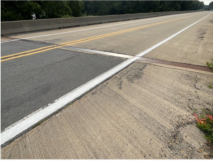
Joint at bent 6
