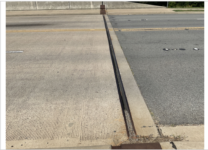
Joint at bent 1 needs cleaning
