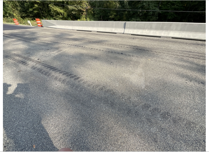
Polymer overlay added
