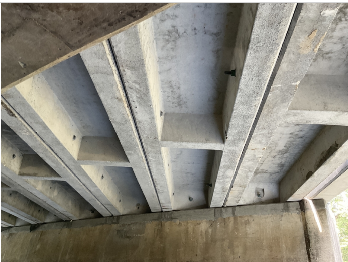
Units are bolted and grouted
