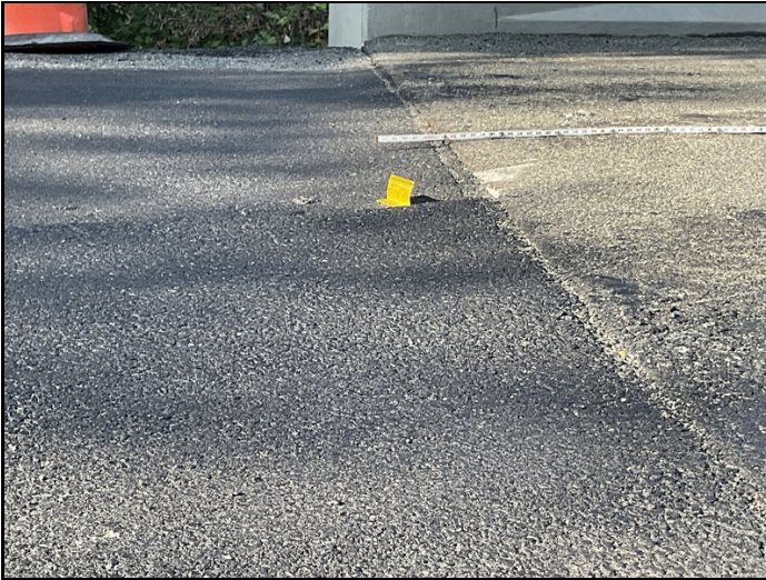
Approach roadway has settled at the east end of the bridge
