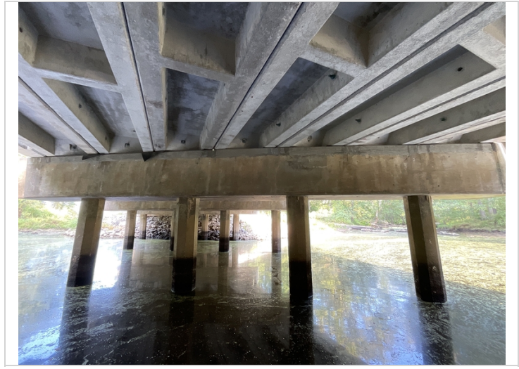
Caps have crown added 5" at ends 6" in the middle
