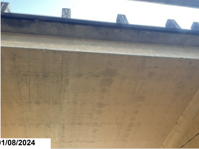
Small spalls on left side of slab
