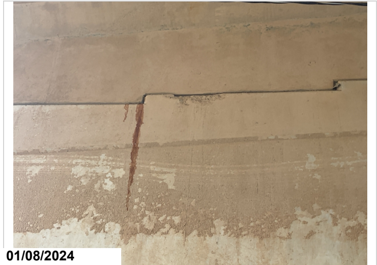
Bent 1 small spall
