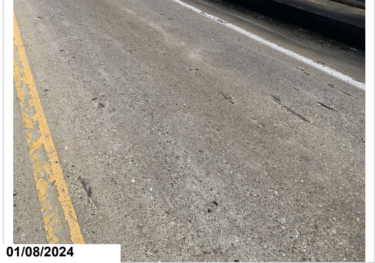
Deck, spalls with exposed rebar in right lane
