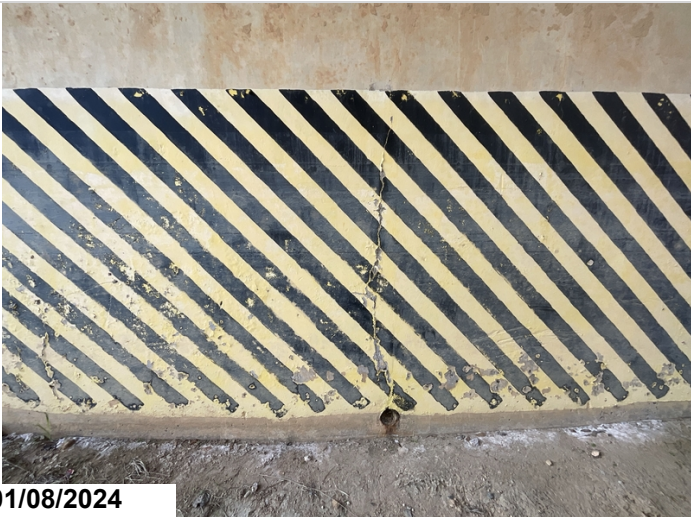
Bent 1 vertical crack up to 0.030"
