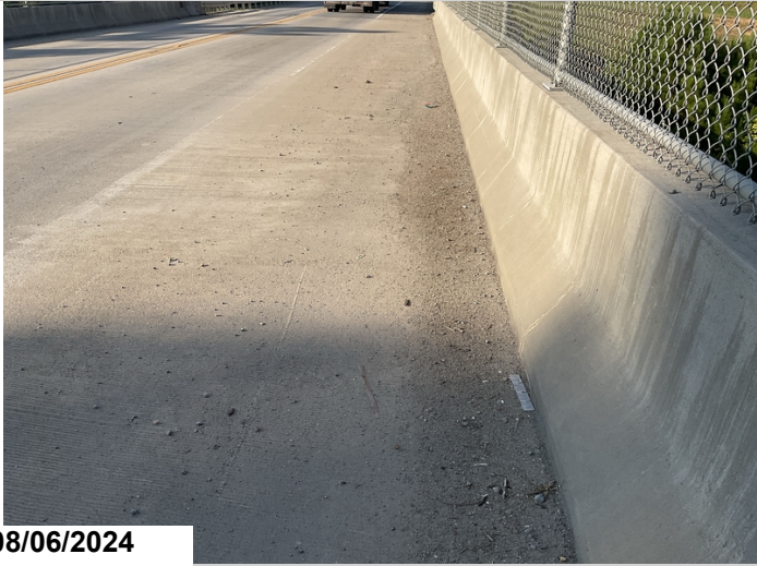
Gutter line is full of debris.
