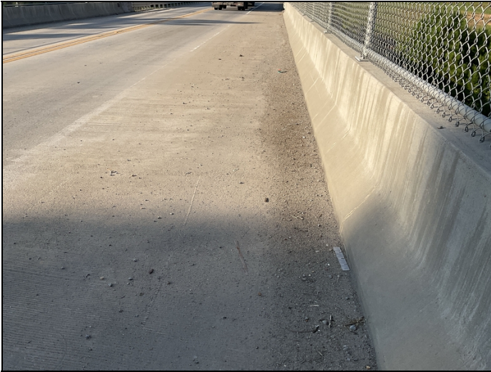
Gutter line is full of debris.
