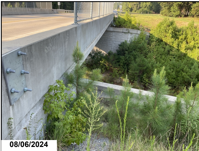
Small trees are growing up against the bridge on all four corners and MSE wall.
