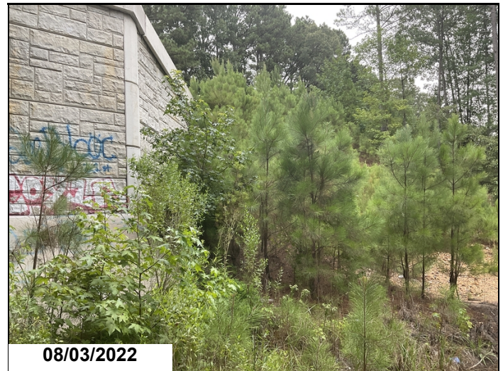
Trees growing at MSE wall at northeast corner.
