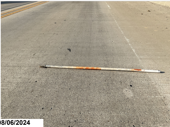
Multiple unsealed longitudinal cracks that span the entire length of the deck.
