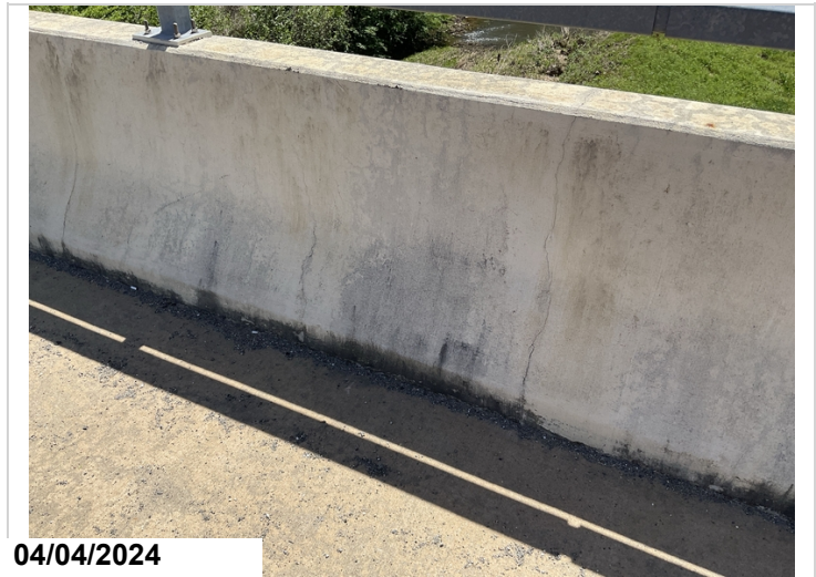
Span 1 right bridge rail. Typical cracks up to 0.020". CS2
