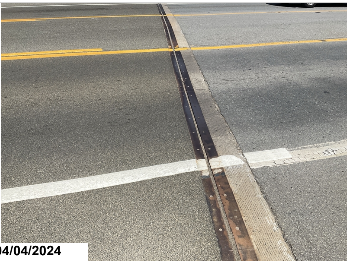
Bent 4 Joint seal is particularly filled with debris
