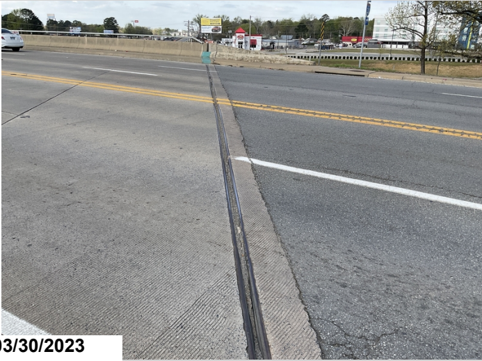
Bent 5 joint seal is torn and leaking
