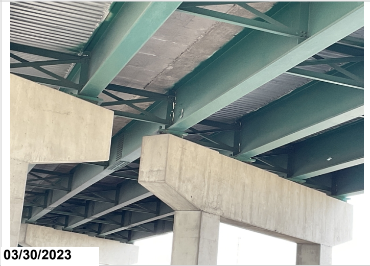
Span 4 girders 1,3&4 at bent 4 have peeling paint
