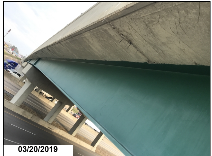
Span 1 left side soffit overhang has cracks with efflorescence and stalactites.
