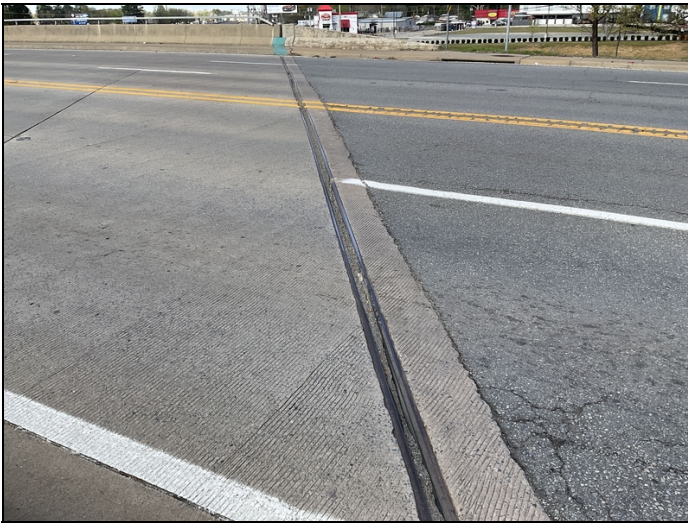
Joint seal at bent 5 is full of debris
