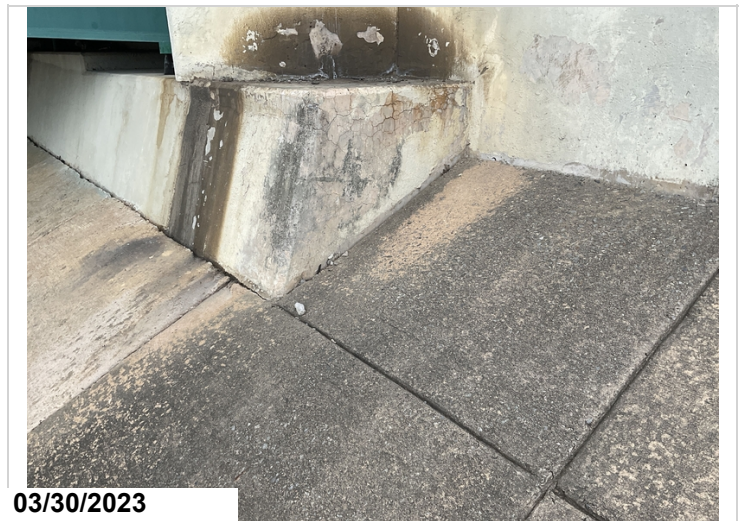
Map cracking on left end of bent 1
