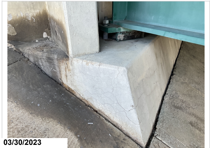
Bent 5 cracks on left end. Common right end
