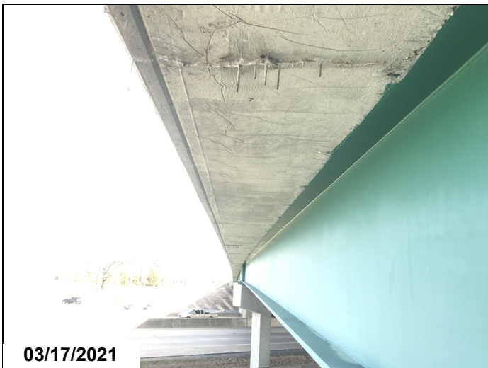
Span 1: left overhang has transvers cracking with heavy efflorescence build up.
