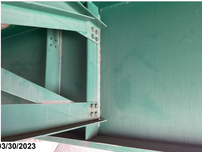
Bent 1 girder 4, loose diaphragm bolts on right side Common left side of girder 5
