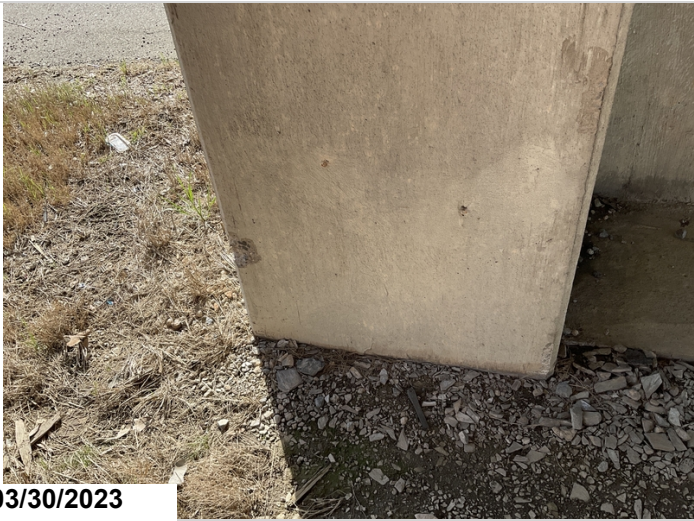
Small spall column 4 at bent 2
