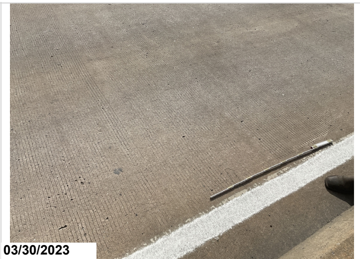
Span 1 map cracking
