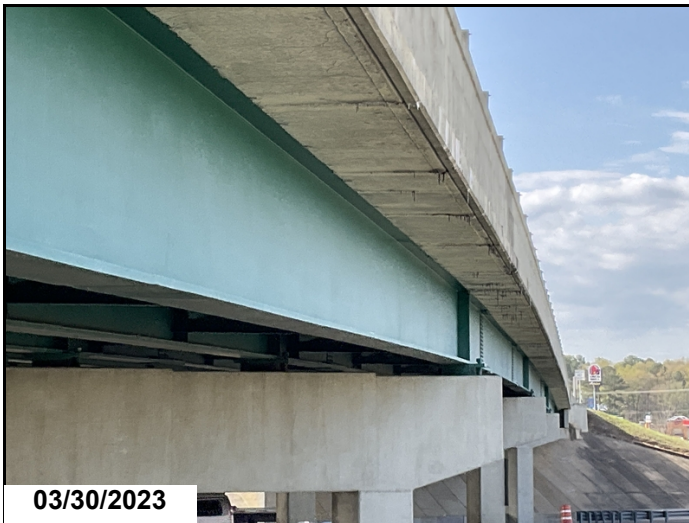
Spans 3&4 left side soffit overhang has cracks with efflorescence and stalactites.
