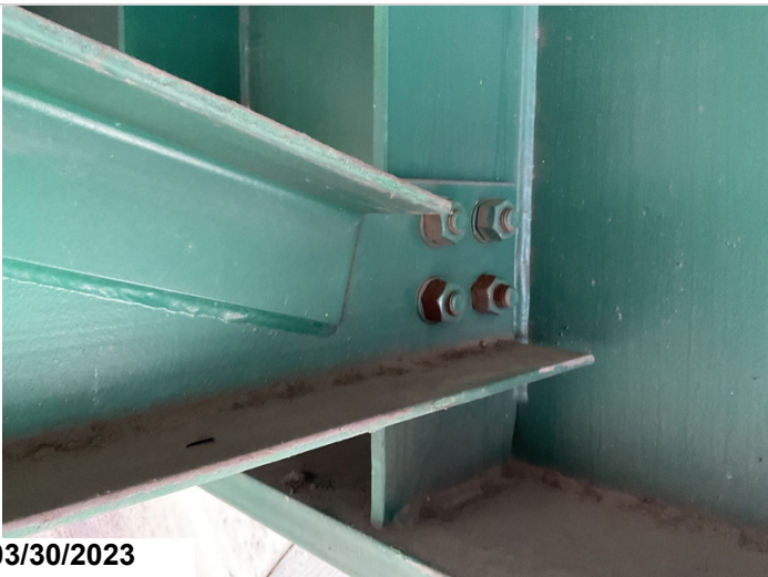
Bent 5 girder 5 left side 3 loose diaphragm bolts
