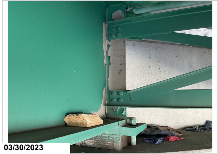
Bent 1 girder 3 peeling paint
