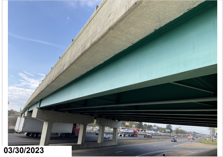
Paint is chalky on outside of girder 9
