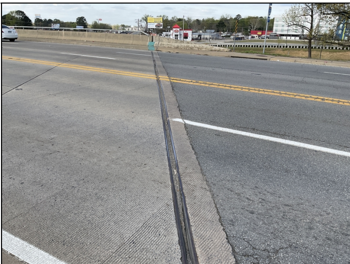
Bent 5 joint seal is torn and leaking
