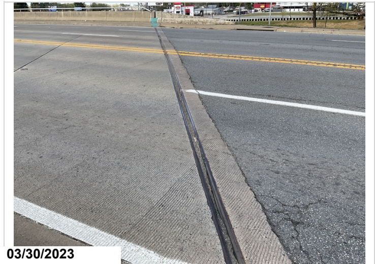
Joint seal at bent 5 is full of debris
