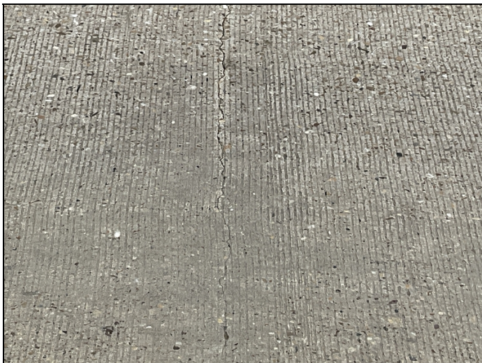
Span 6 transverse crack up to .040" wide.
