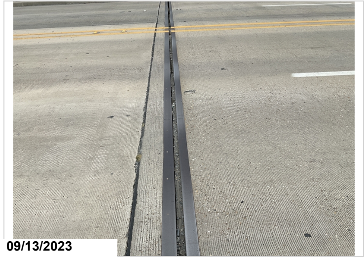
Bent 1 pourable joint seal has lost bond.
