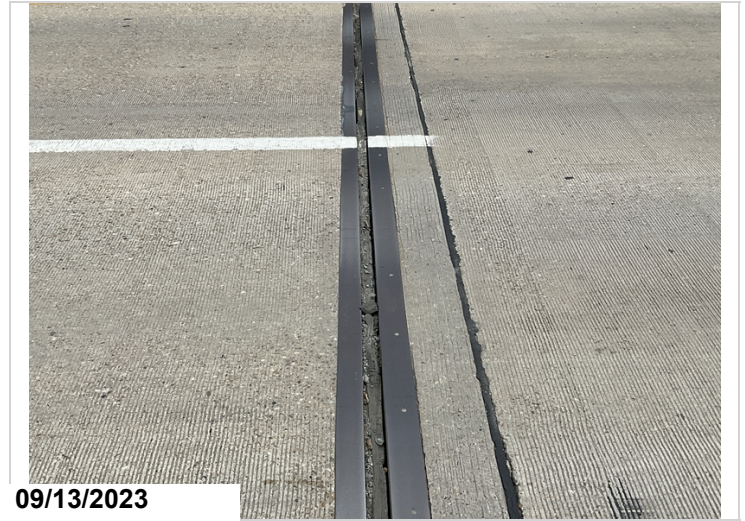
Bent 6 pourable joint seal has lost bond.
