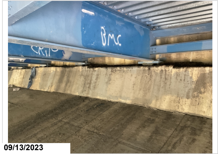
Bent 6 dirt and debris built up on abutment due to leaking joint seals.
