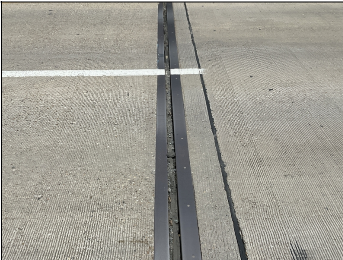
Bent 6 pourable joint seal has lost bond.
