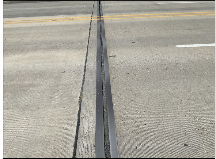
Bent 1 pourable joint seal has lost bond.
