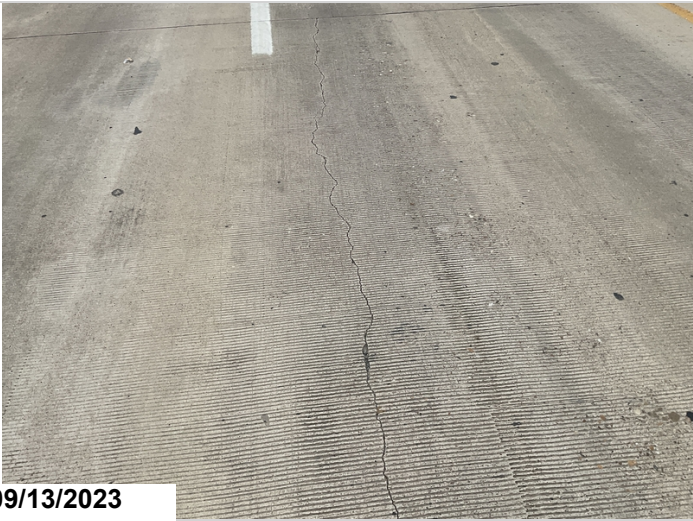
South approach slab longitudinal crack. Up to 0.60" wide.
