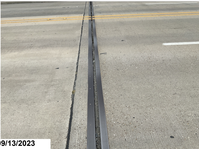
Bent 1 pourable joint seal has lost bond.
