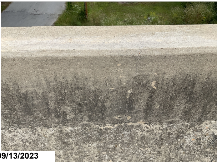
Span 1 bridge rail left side small vertical crack.
