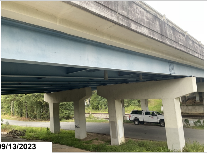
Span 1 beam 8 paint system is chalky.
