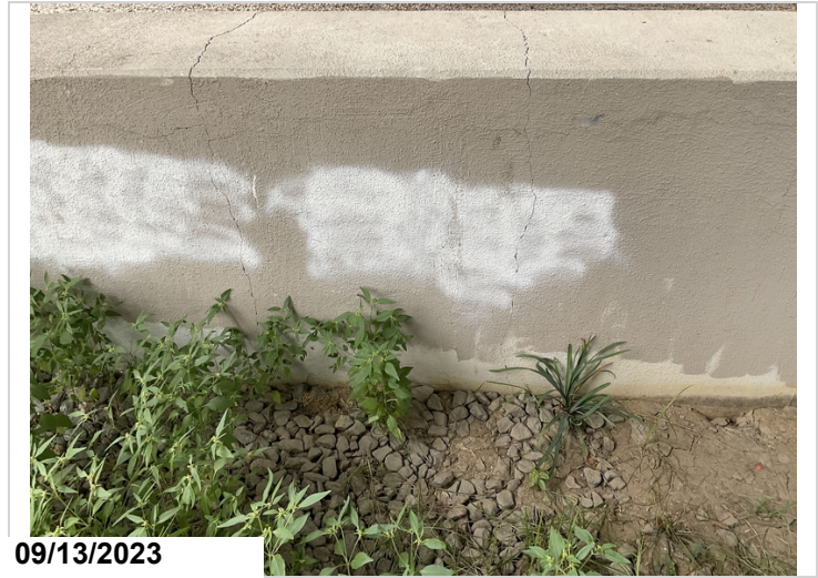
Bent 2 pier wall between columns 1 & 2 cracks.
