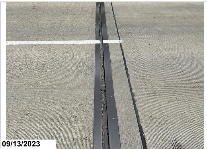
Bent 6 pourable joint seal has lost bond.
