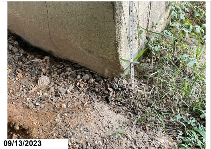
Bent 5 column 4 back left side at ground line minor spall.
