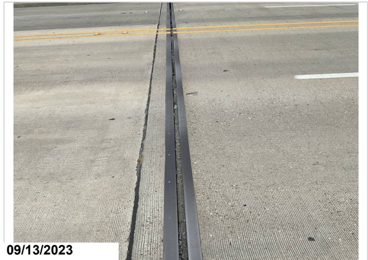
Bent 1 pourable joint seal has lost bond.
