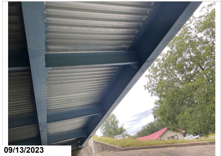
Beam 7 & 8 minor scrapes to bottom flanges due to traffic impact.
