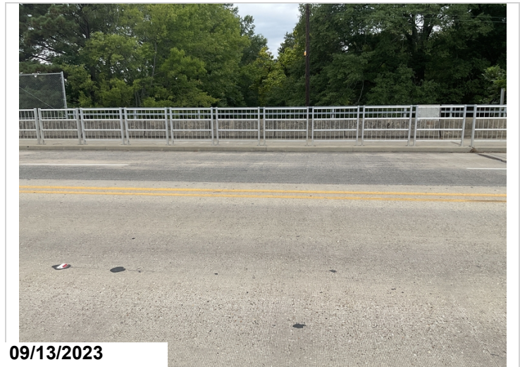
Span 6 south bound lanes have light abrasion.
