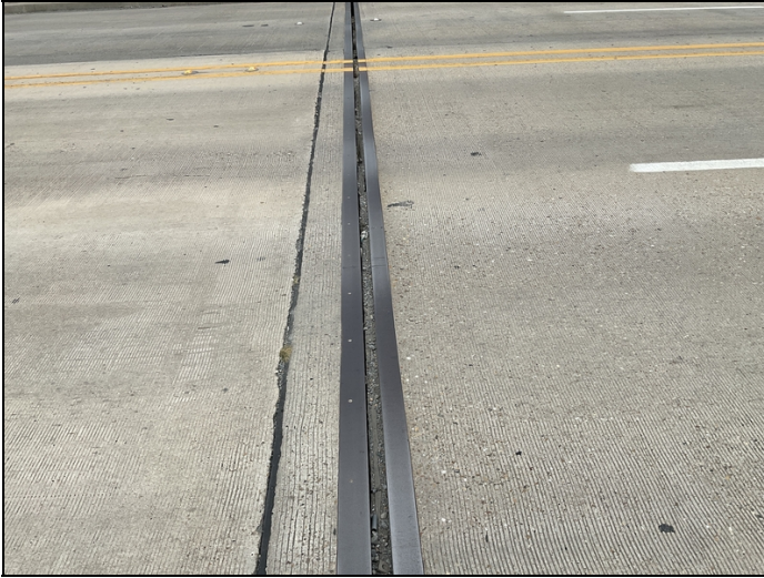
Bent 1 pourable joint seal has lost bond.
