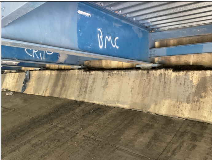
Bent 6 dirt and debris built up on abutment due to leaking joint seals.
