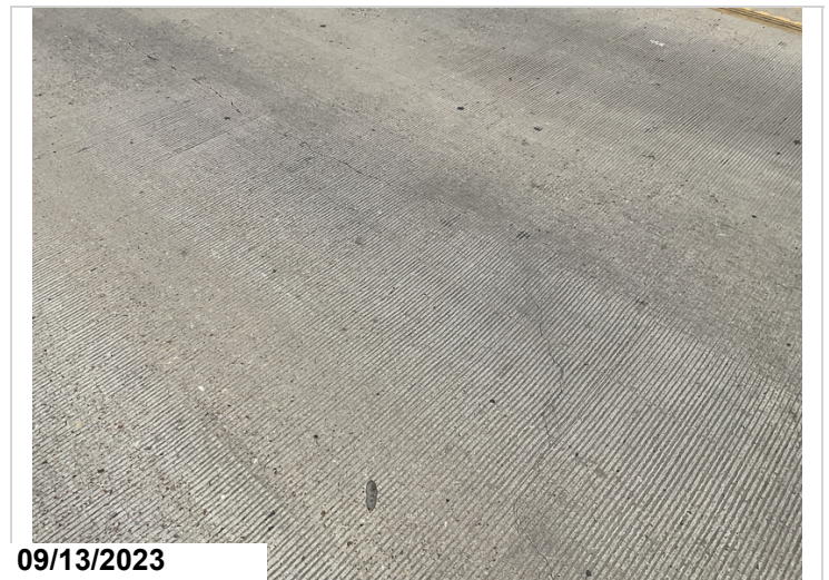
North approach slabs has small cracks.
