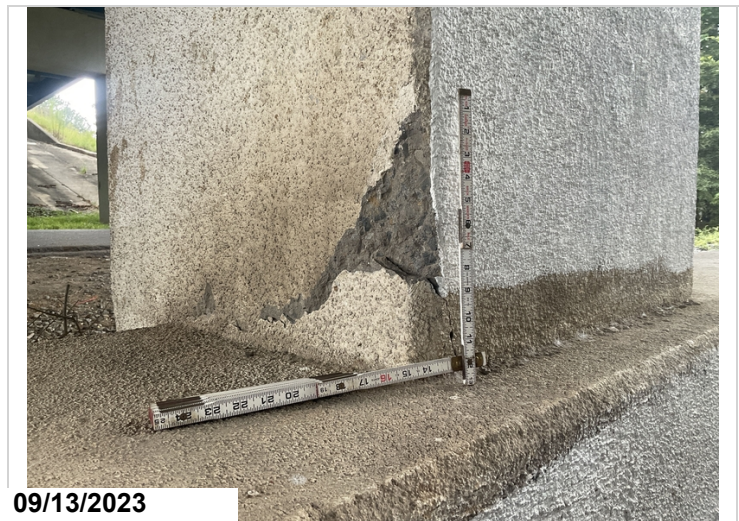
Bent 2 column 2 right side above pier wall spall.
