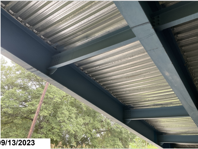
Beam 1 & 2 minor scrapes to bottom flanges due to traffic impact.
