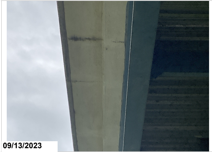
Span 4 soffit overhang cracks with light efflorescence.
