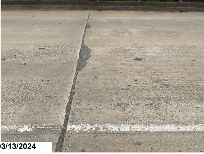
Span 3 at bent 3 spall and spall filled with asphalt.
