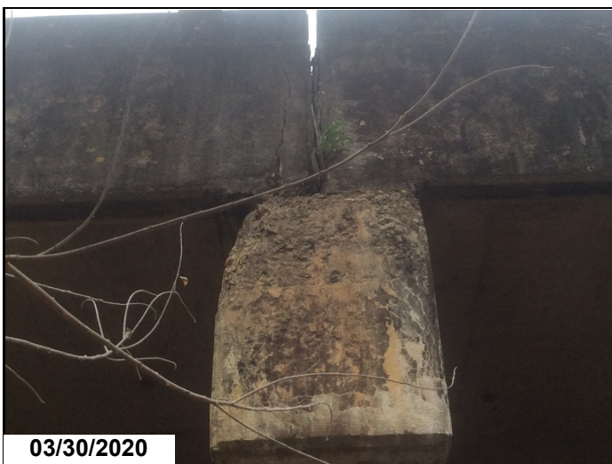
Span 2 right side at bent 3 delam on slab and spall on end of cap.
