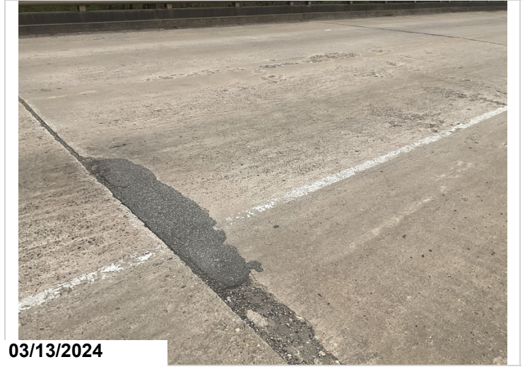
Span 5 spalls and spalls filled with asphalt.
