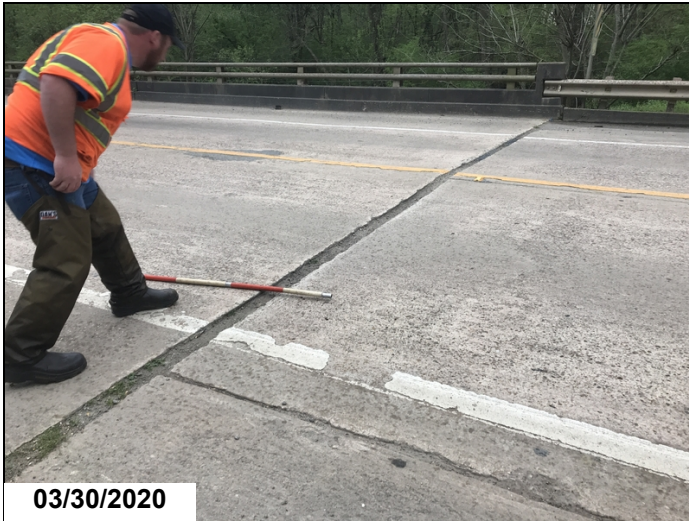
Approach at north end of bridge has setteled.
