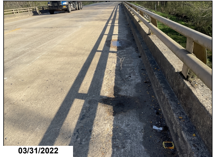
Span 3, right shoulder: couple open spalls
