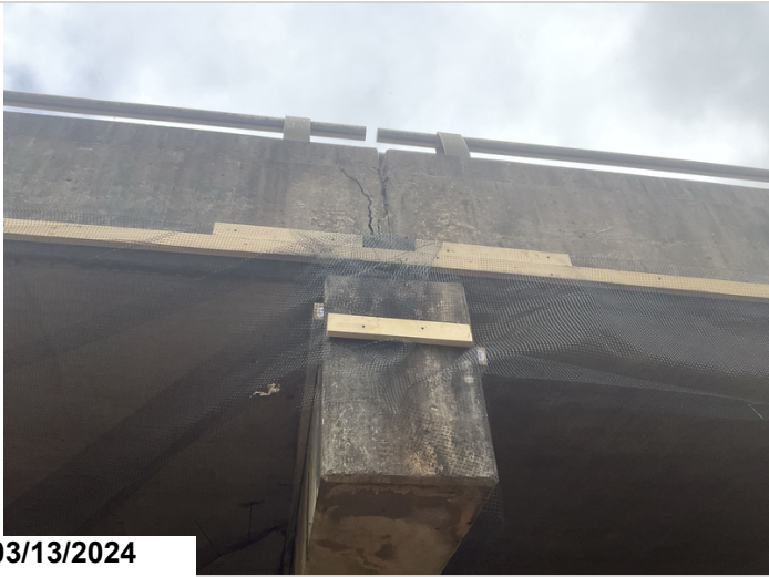
Span 3 right side of slab at bent 3 delamination.
