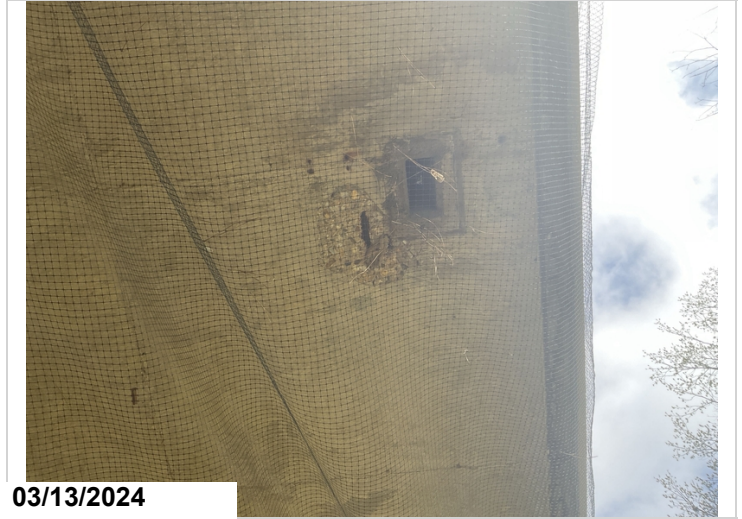
Span 5 spall with exposed rebar at right scupper drain.
