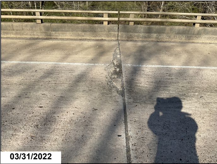
Bent 6: Spall in the left lane
