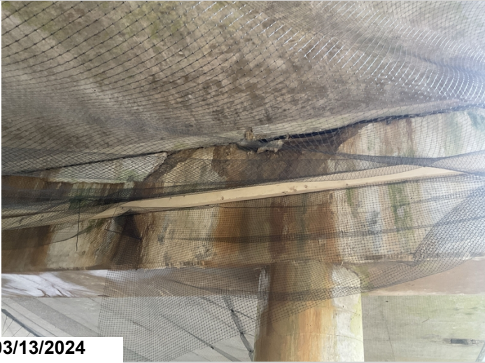
Bent 2 cap back at column 3 spall and delam.
