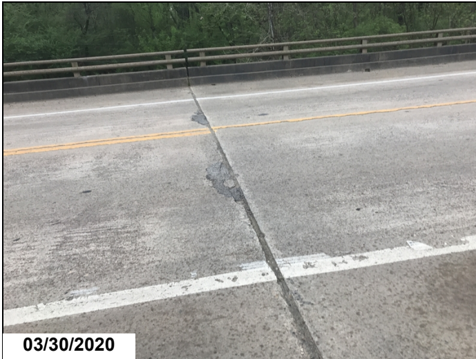
Span 3 spalls filled with asphalt.
