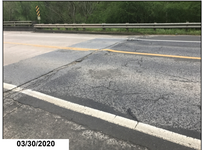
Asphalt has heaved up causing traffic to impact load the approach slab at the north end of the bridge.
