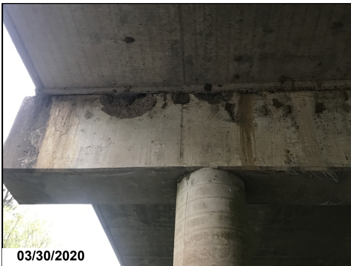
Cap at Bt. 4, back left side, spall.
