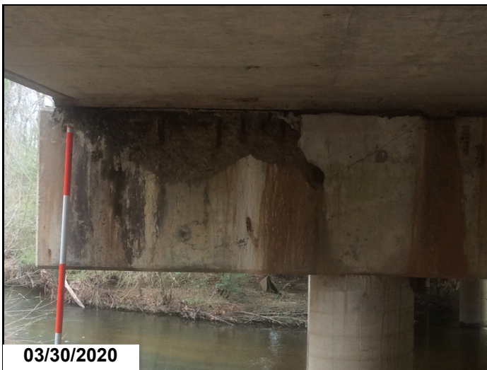
Bent 2 cap back left of column 1 spall with exposed rebar.
