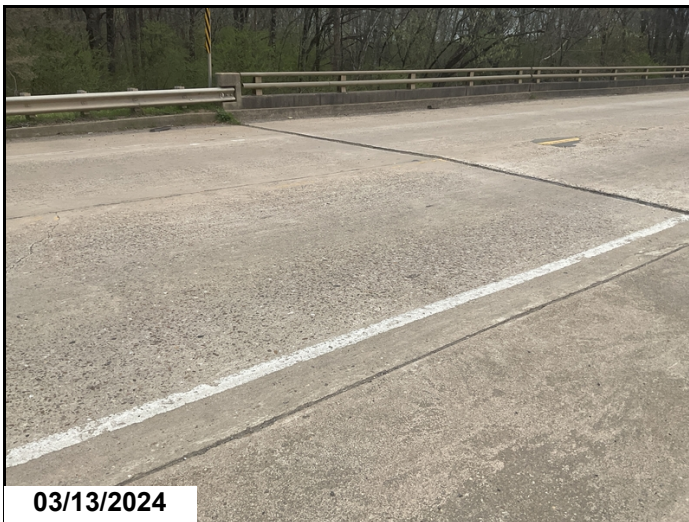
North approach slab has settled up to 2"
