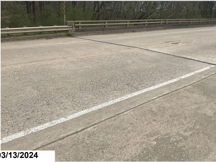
North approach slab has settled up to 2"
