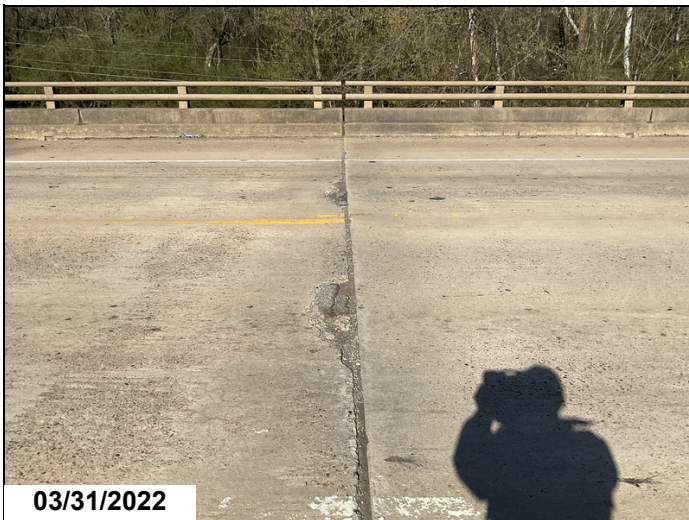
Bent 4: couple open spalls at the joint.
