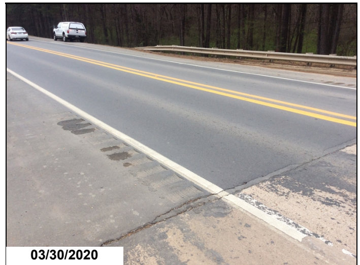
The south approach slab that has been overlaid.
