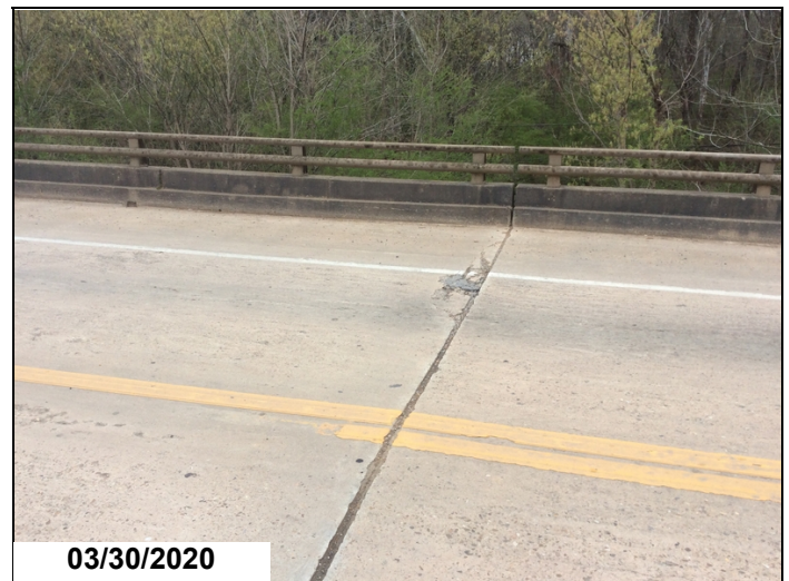
Spalls in the deck at span 3 bent 4.
