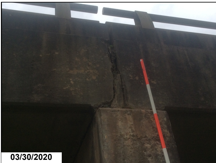
Span 5 at bent 6 delamination on the right side of slab.
