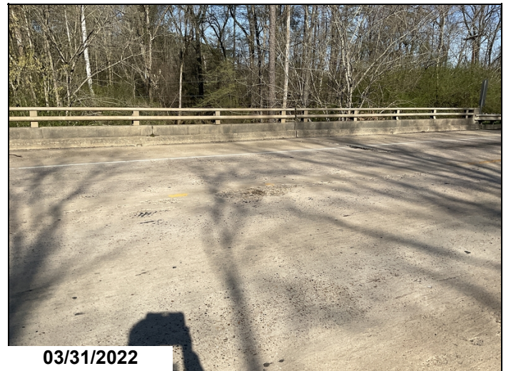
Span 5: Spall at centerline.
