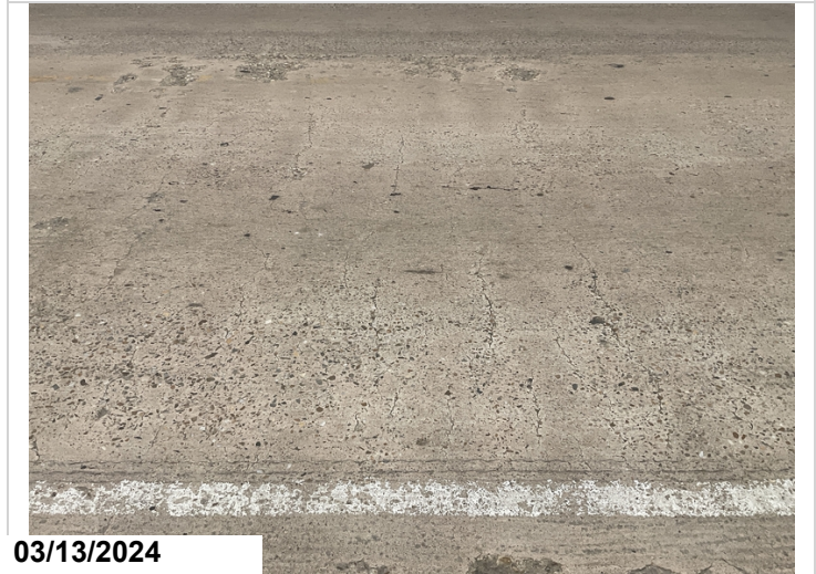
Deck span 2 transverse cracks on two foot centers.
