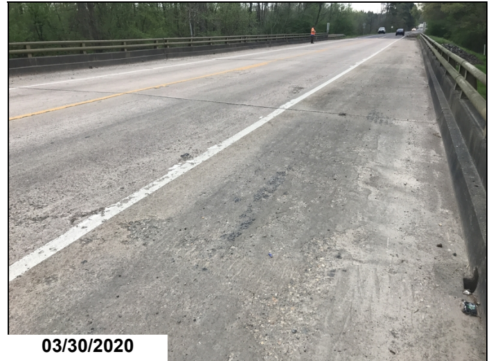
Spans 1 & 2, heavy scaling.
