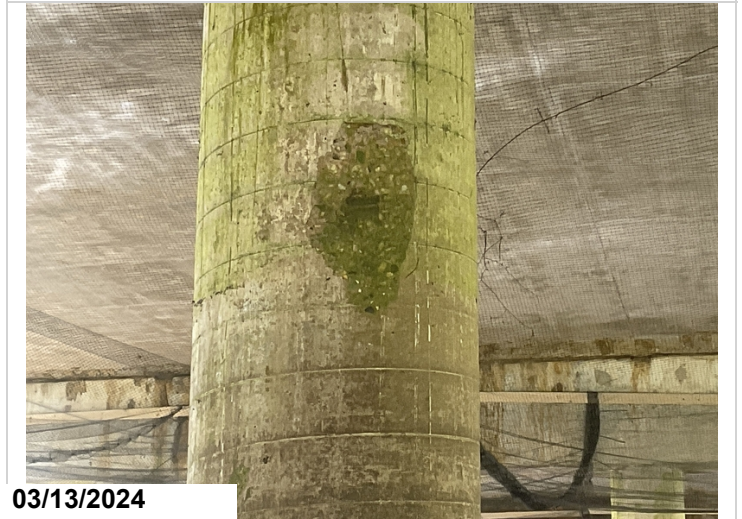
Bent 2 column 5 ahead spall with rebar.
