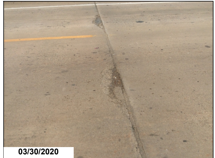
Spalls in the deck at span 3 bent 4.
