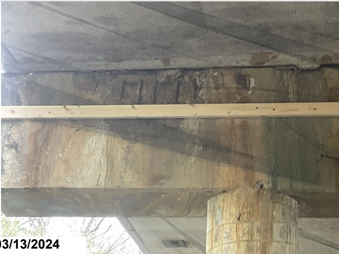
Bent 6 cap back left of column 1 spall with rebar.
