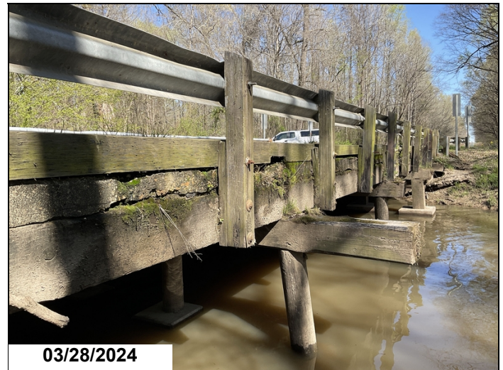
Bridge rail post are loose on both left and right sides.
