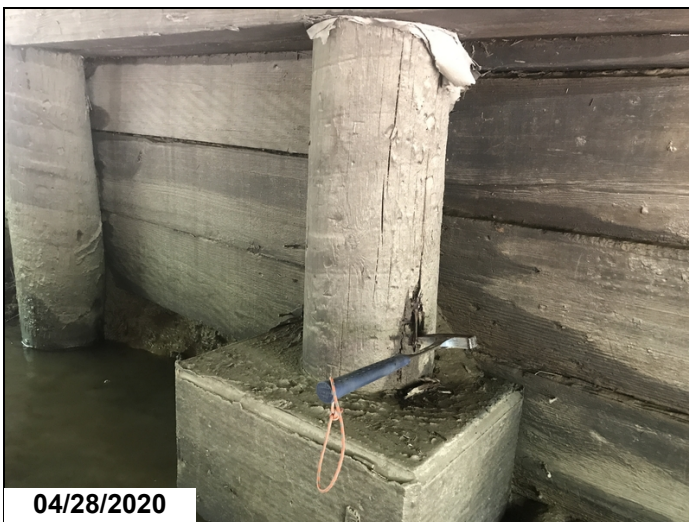
Bent 6, pile 3: the pile is cracked and is decaying.
