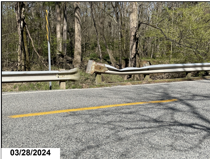
Tree has fallen on left bridge rail at bent 1 causing damage to 15'.
