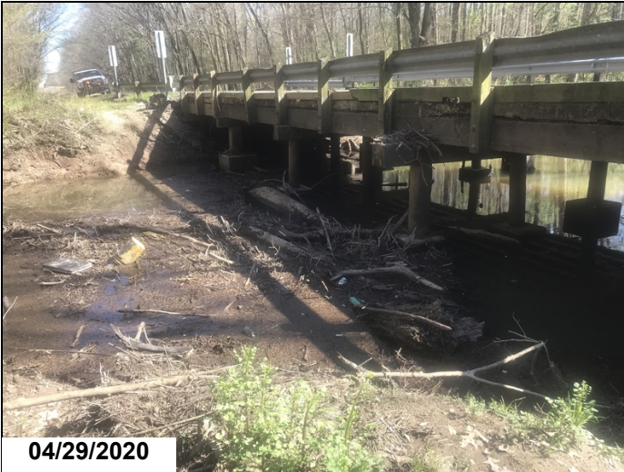
Logs and debris build up at west end of the bridge restricting water flow
