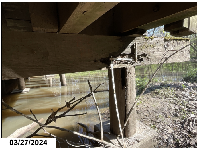
Bent 2 pile 5 is decayed and split
