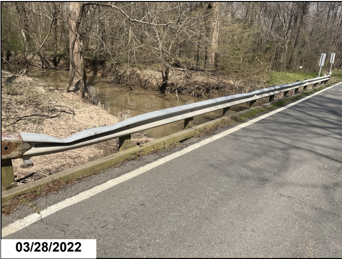
Left bridge rail is damaged
