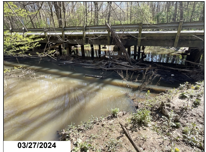
Logs and debris on west side
