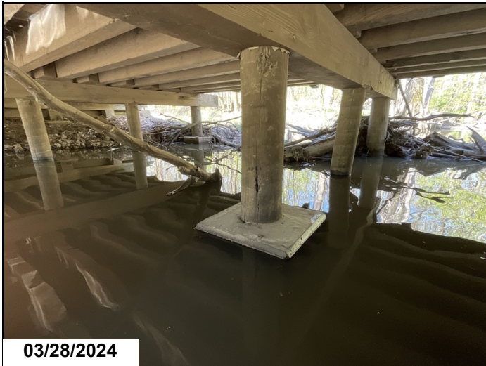
Bent 3 pile 3 cracked with decay
