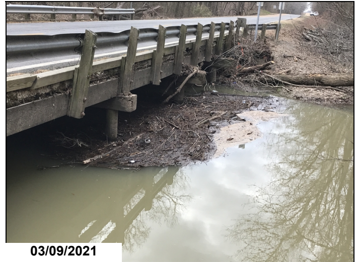
Logs and debris build up at west end of the bridge
