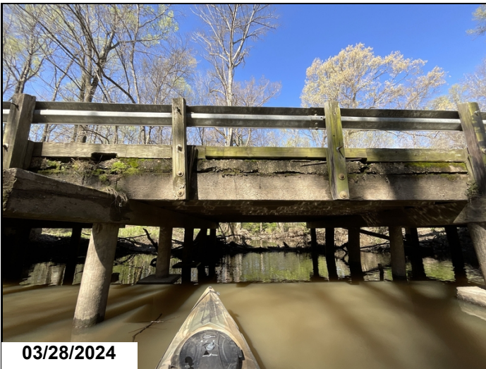
Concrete deteriorating at both left and right sides of the deck
