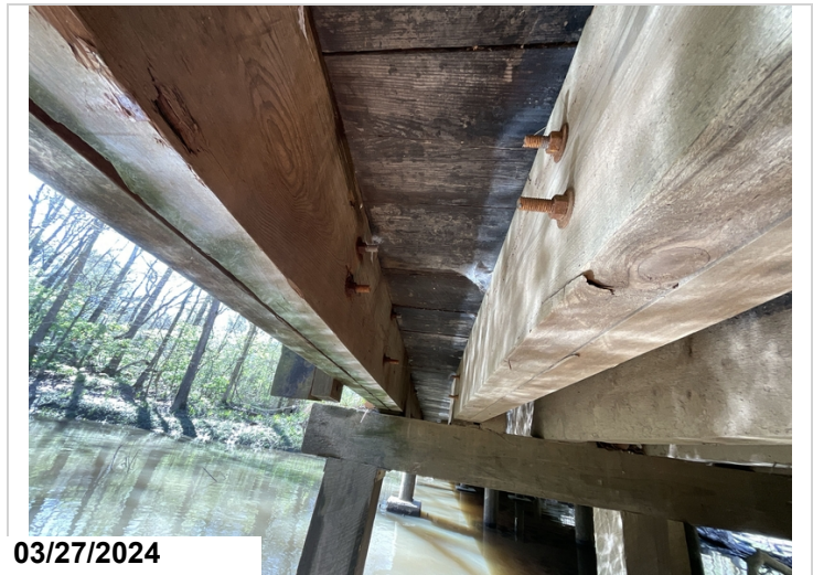
span 5 girder 12 has a split to one of the bolted together girders.
