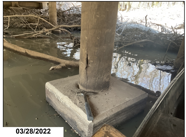
Bent 3 pile 3 is split and decayed.
