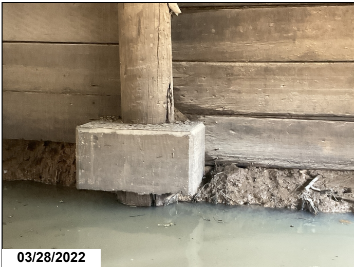
Bent 6 pile 3 is split and decayed at bottom near concrete collar
