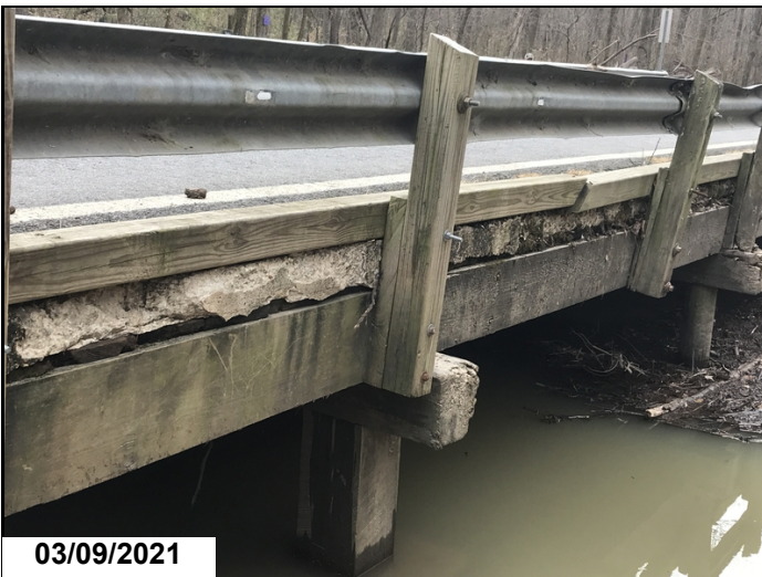
Span 2 and 3 right side of deck has spalls
