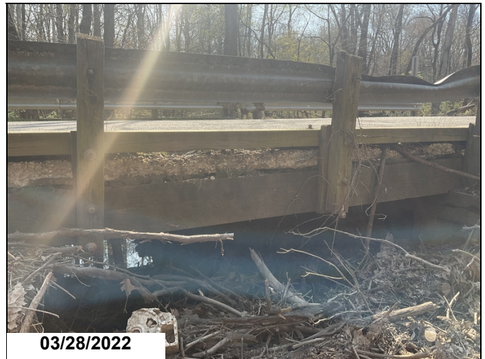
Span 1 left side spalling due to concrete deterioration.
