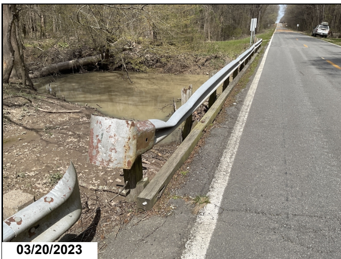
Guardrail damage at southwest end
