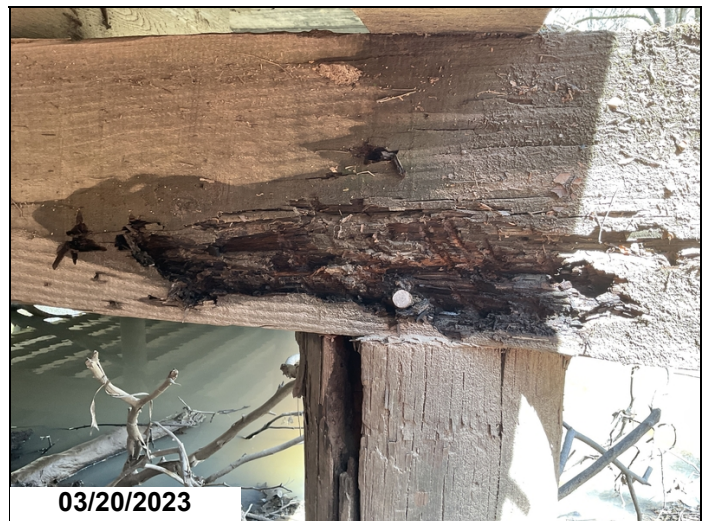
Bent 2 cap over pile 5 has a 2'x 6" x1" deep decay
