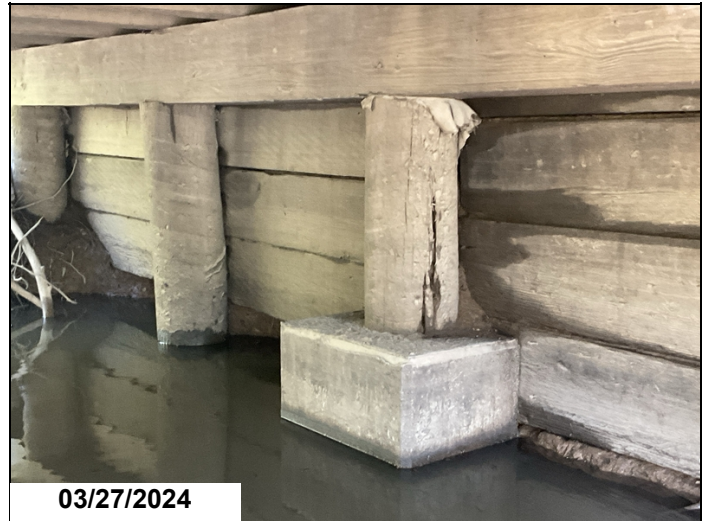
Bent 6 pile 3 split and decayed
