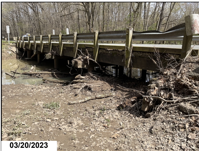
Debris at bent 2 and 3 upstream end
