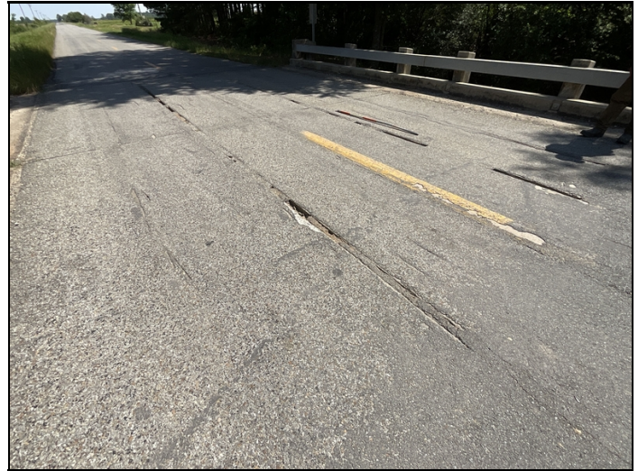
Grout missing from between channel units
