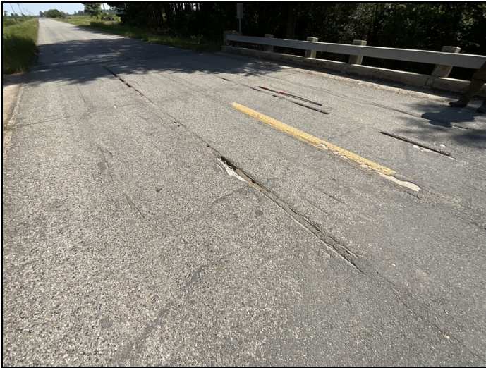
Grout missing from between channel units
