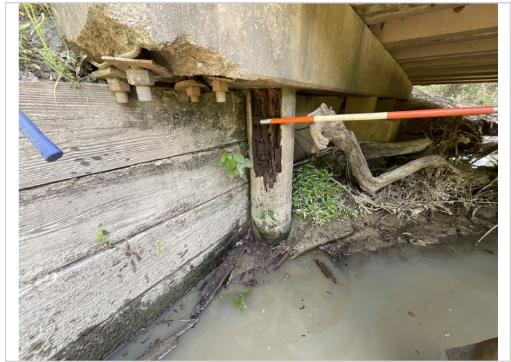
Bent 1 pile 5 2' tall 6" deep decayed section
