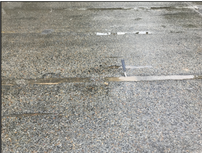
Deck has small spalls in grouted keyways between channel units.
