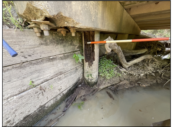
Bent 1 pile 5 2' tall 6" deep decayed section
