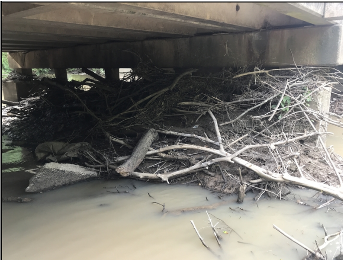
Bent 2: large amount of drift and sediment against pile.
