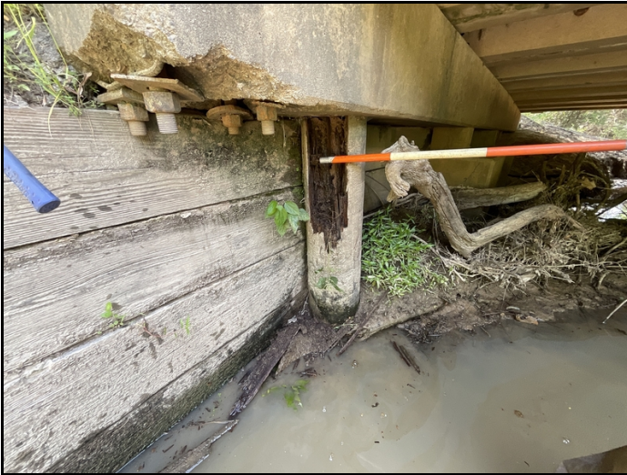
Bent 1 pile 5 2' tall 6" deep decayed section
