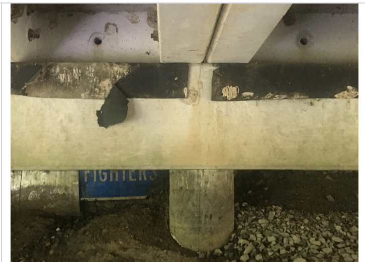
Bent 4 cap has a vertical crack above pile 3
