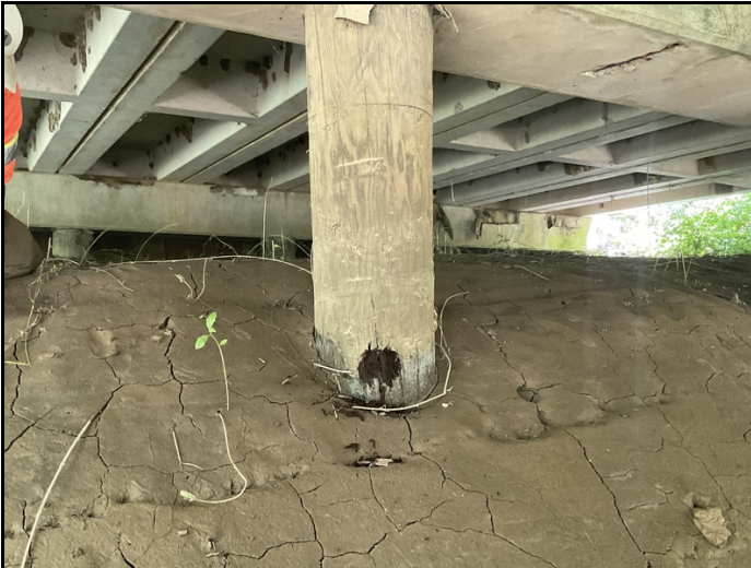
Bent 2 pile 4 ahead side decay at bank line
