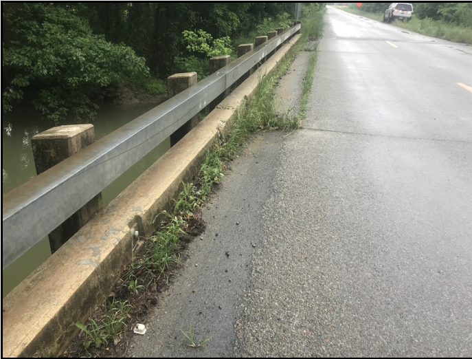
Debris and vegetation in both gutter lines.
