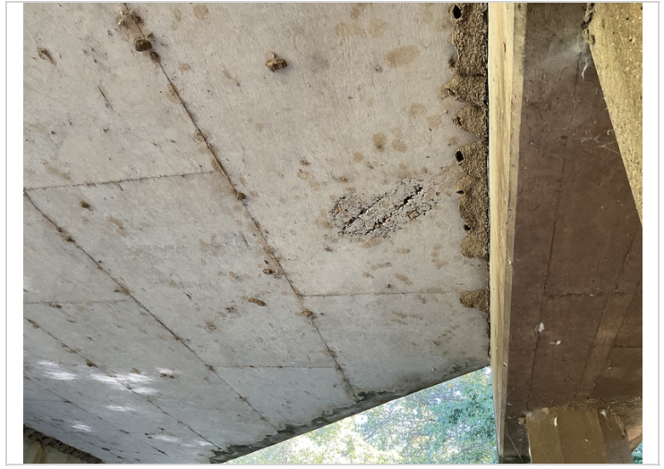
Honeycomb in soffit at bent 3
