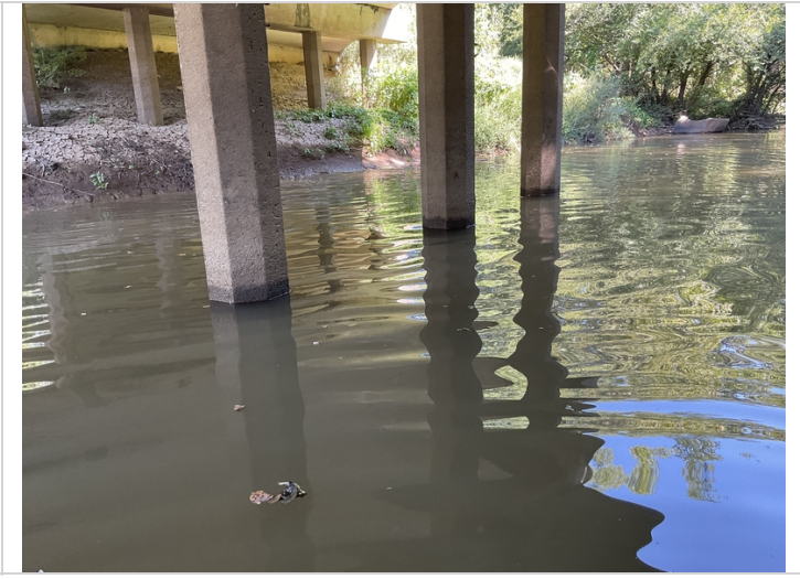
Abrasion to piles at the water line
