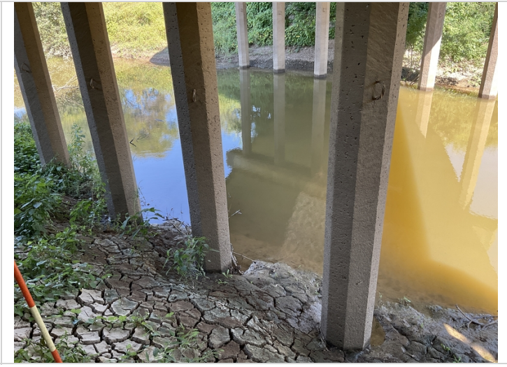
Abrasion to the piles
