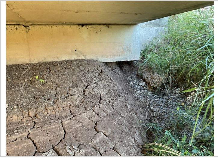
Bent 4 right side exposed pile
