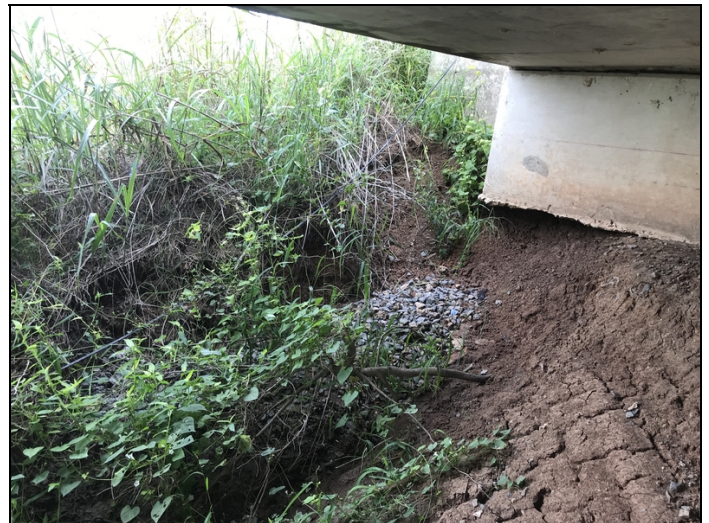
Bent 1: the embankment is eroding and undermining the abutment
