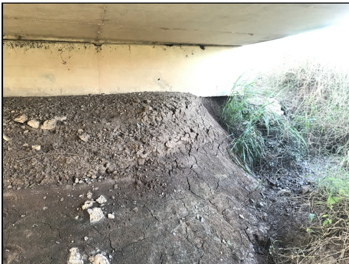
Bent 4: left end of abutment, the embankment is eroding
