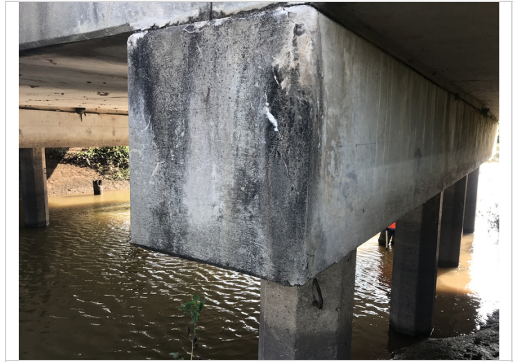
Right end of bent 3 cap has small cracks with efflorescence
