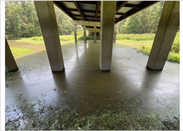
Abrasion to bottom of piles
