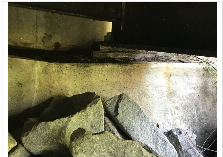
Laminating rust on bearing 1 at bent 1
