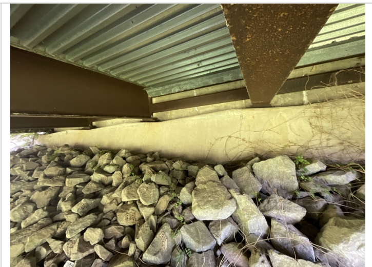
Bent 7 abutment vertical cracks with efflorescence
