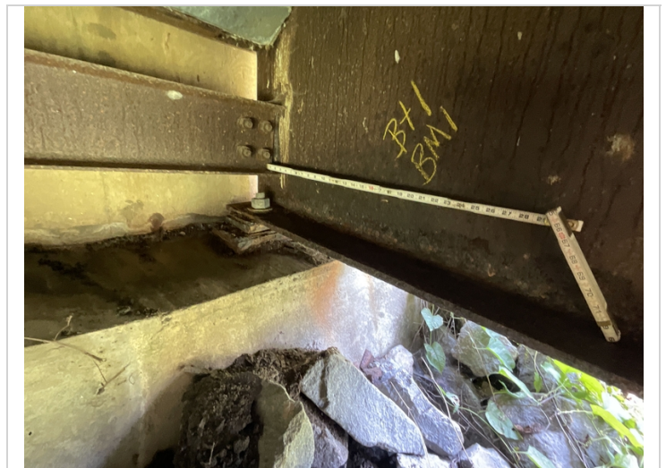
Corrosion at bent 1 beam 1
