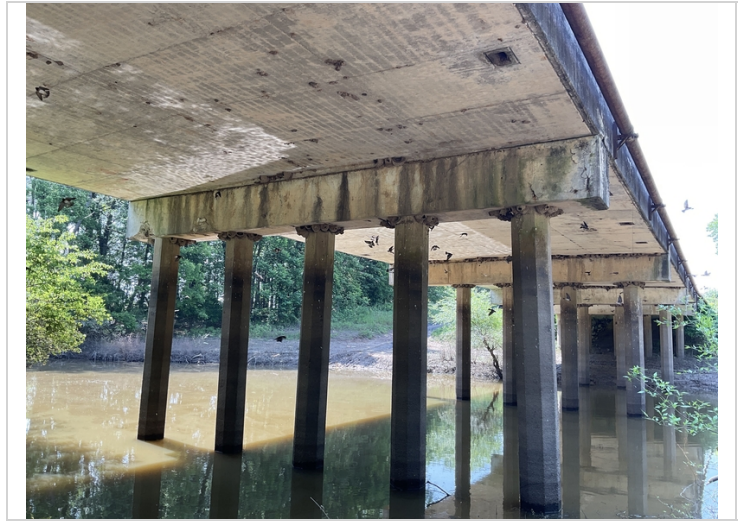
Bent 5 cap has spalls with rebar on both left and right end ahead side
