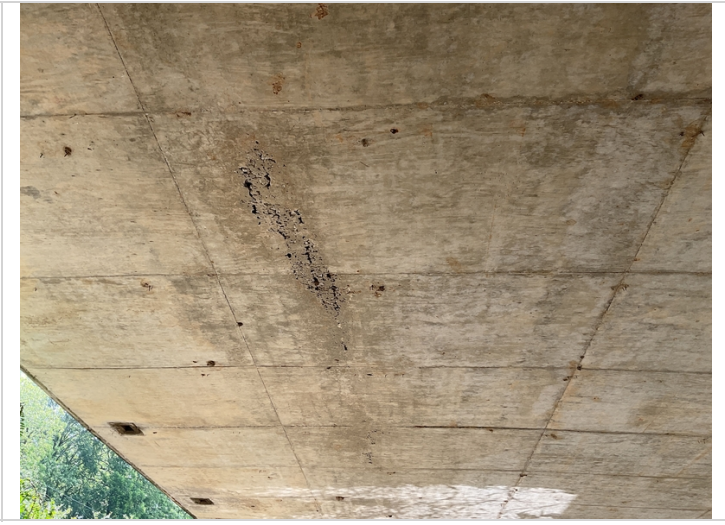
Honeycomb in the soffit span 6
