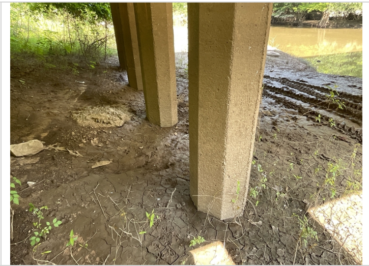
Abrasion to the columns
