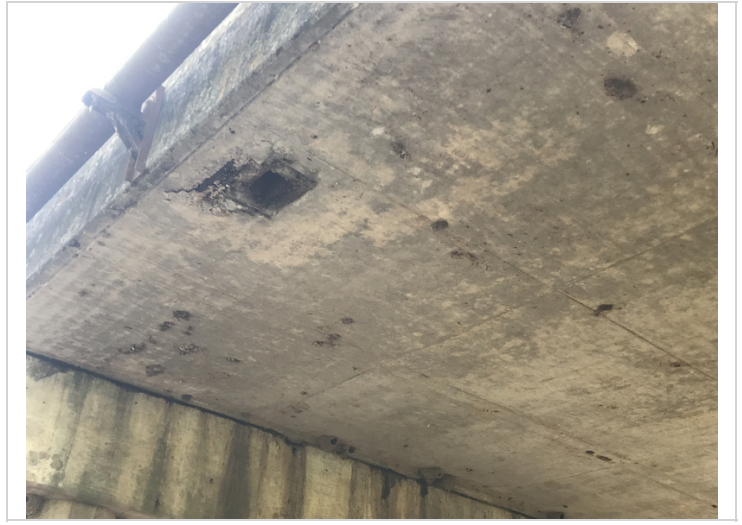
Span 2 left side has exposed rebar around drain.
