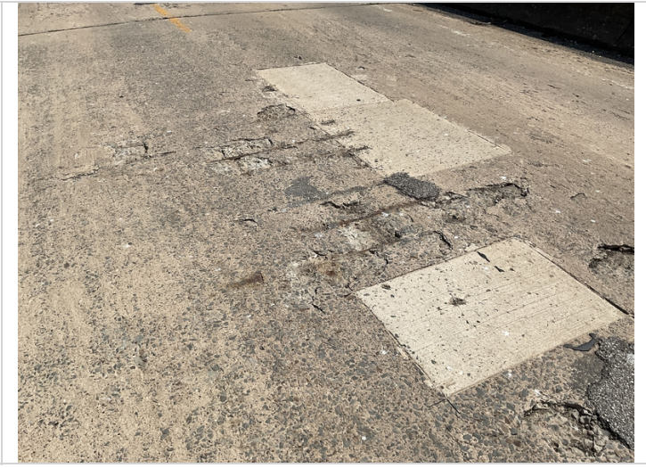
Spalls with rebar span 3
