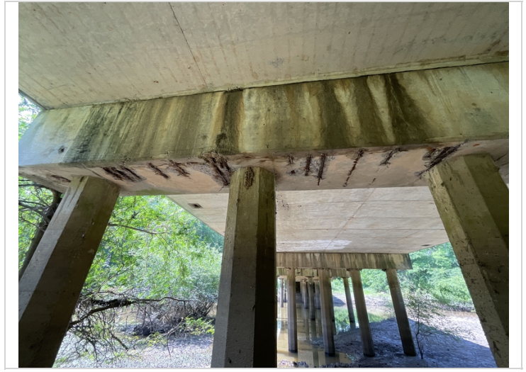
Bent 7 exposed rebar
