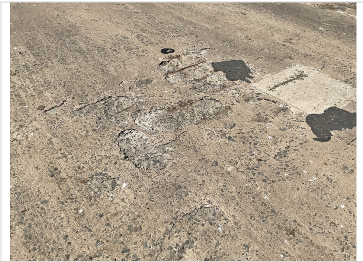
Rebar exposed in the deck
