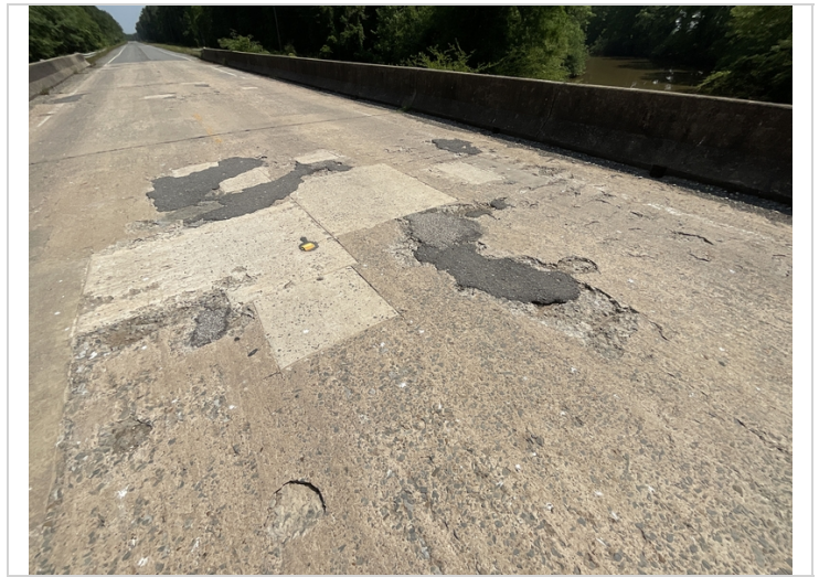
Spalls with rebar span 4
