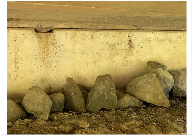
Cracks at bent 1
