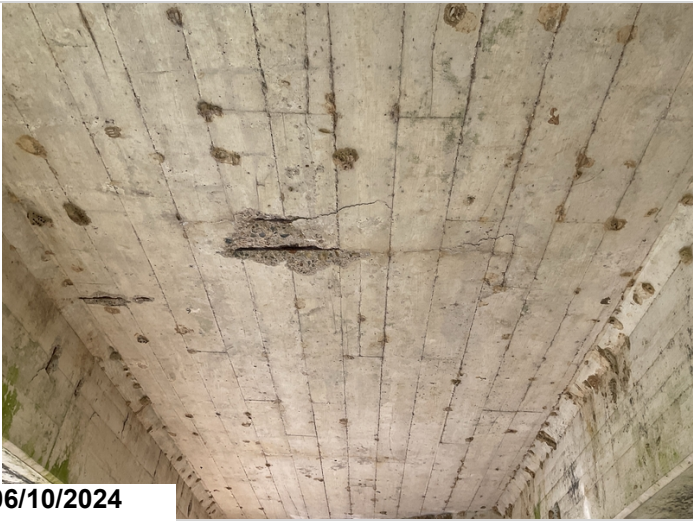
Span 2, right bay: spall with exposed rebar. CS3-3sf
