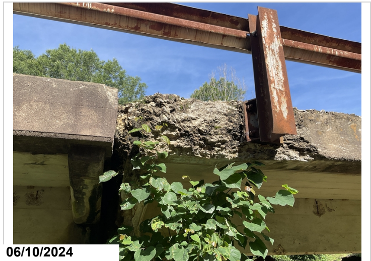
Span 3: right edge of deck is deteriorating and beginning to spall.
