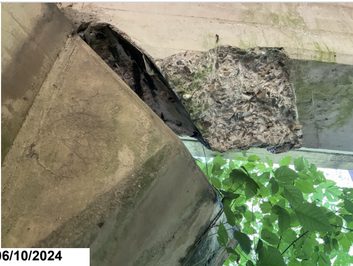
Bent 3, span 3, girder 1: spall with exposed rebar. CS3-1'
