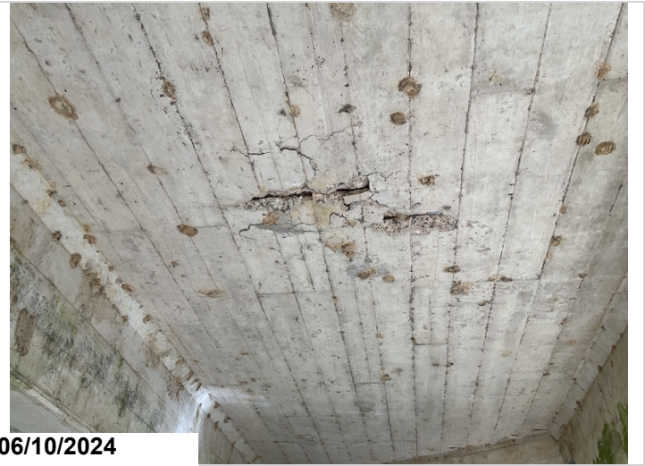
Span 1, between girders 2&3: spalls with exposed rebar. CS3-5sf
