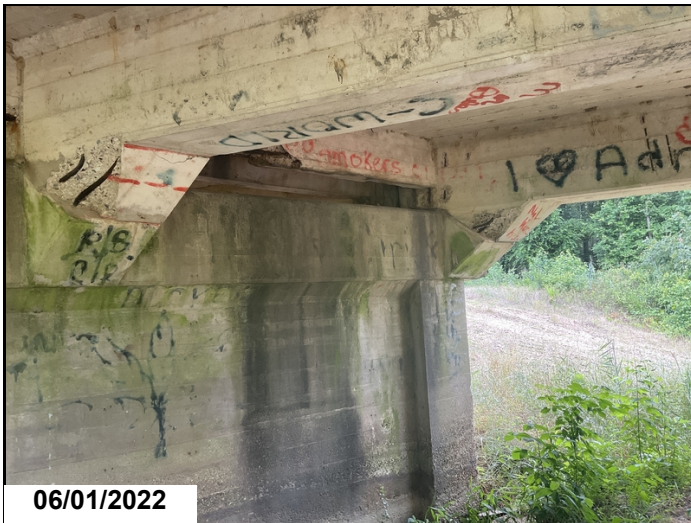
Bent girders 2 & 3 have spalls with exposed rebar.
