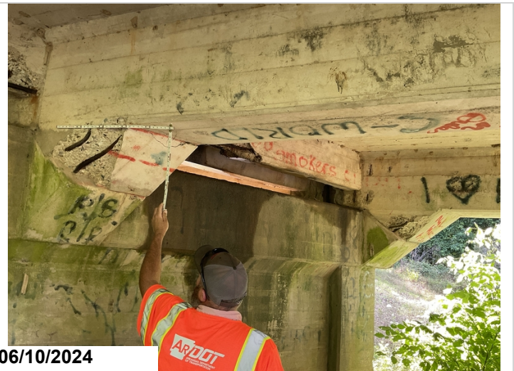
Backside bent 3, girders 2 and 3 are spalled with exposed rebar. CS3-2'.
