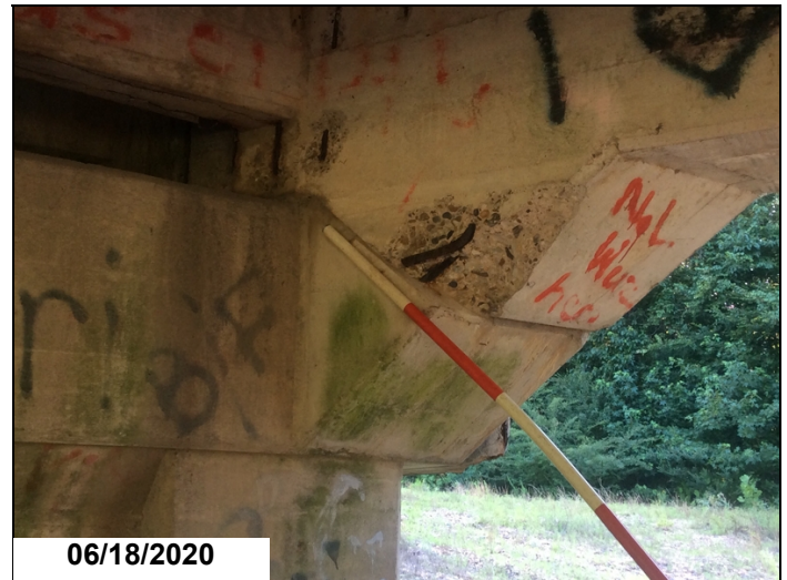
Span 2 girder 3 at bent 3 has spall with exposed rebar.
