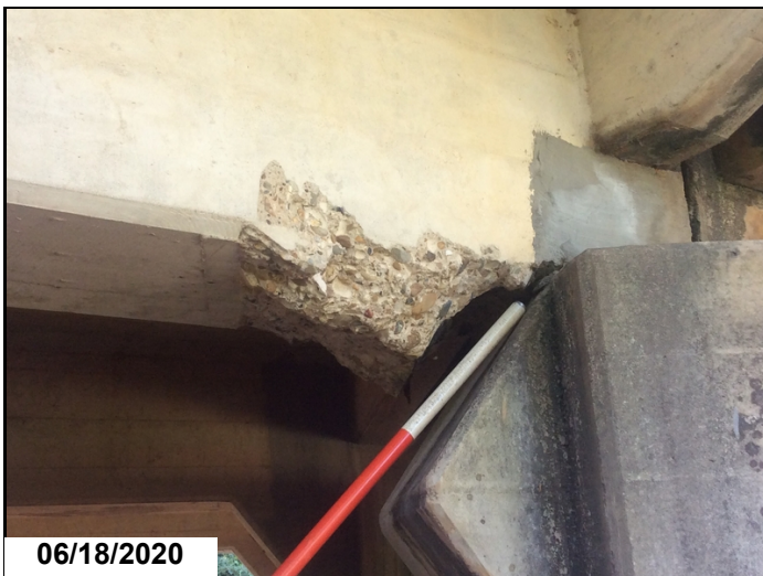
Span 3 girder 1 at bent 3 has spall.
