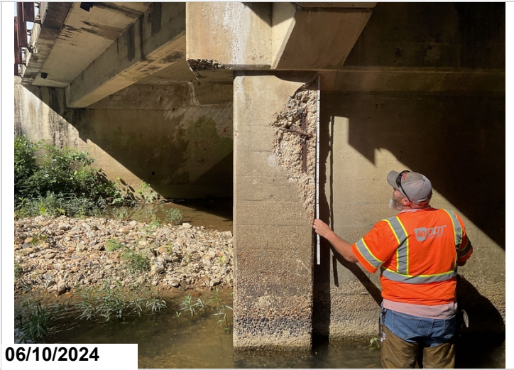
Ahead side bent 2, column 2: large spall with exposed rebar. CS3-1ea.
