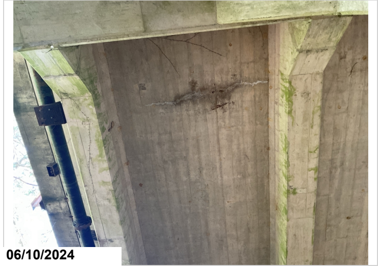
Span 3: transverse crack with efflorescence staining. CS3-8'
