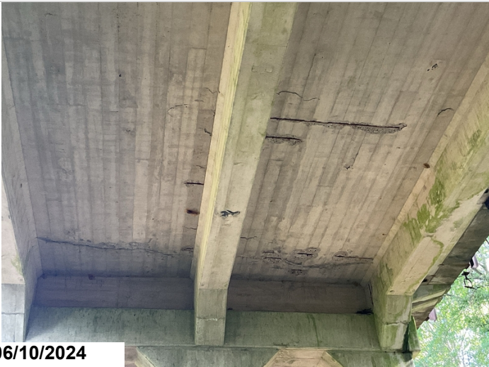
Span 2: numerous spalls with exposed rebar. CS3-33'
