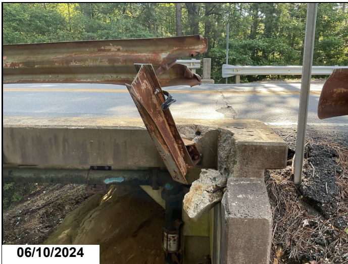
South west guardrail has been damaged. 2024
