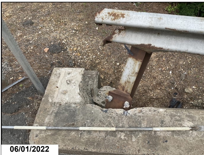
Span 1 left side bridge rail and end post damaged due to traffic impact.
