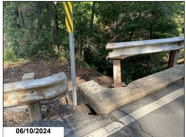
South west guardrail has been damaged. 2024
