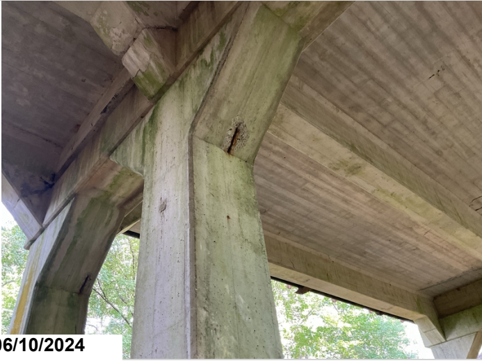
Bent 2, column 2: small spall with exposed rebar. CS3-1ea
