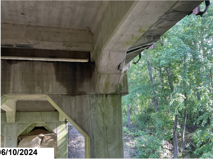
Span 1 at bent 2, girder 3: spall with exposed rebar to the bottom of the girder. CS3-1'
