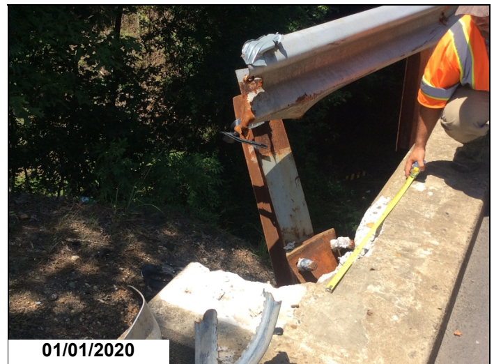
Bridge rail end post damaged left side.
