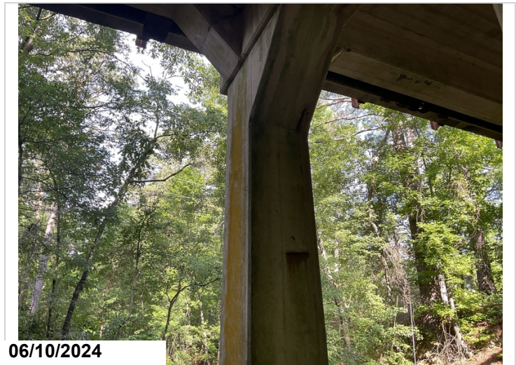
Bent 2, column 1: couple small spalls with exposed rebar. CS3-1ea
