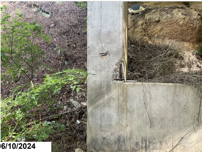
Bent 3, column 1: spall with exposed rebar. CS3-1ea
