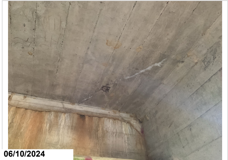
Span 1: Under surface with diagonal crack with some efflorescence staining. CS2-3'
