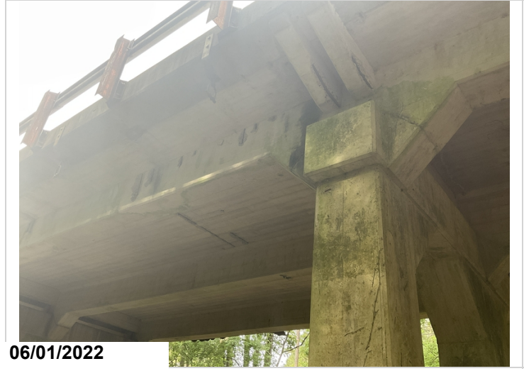
Spalls with exposed rebar in girder 3 right side span 2.
