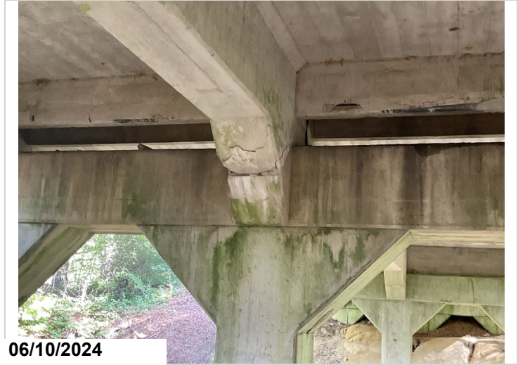
Span 1, bent 2, girder 2: the bottom of girder has a delam. CS3-2'
