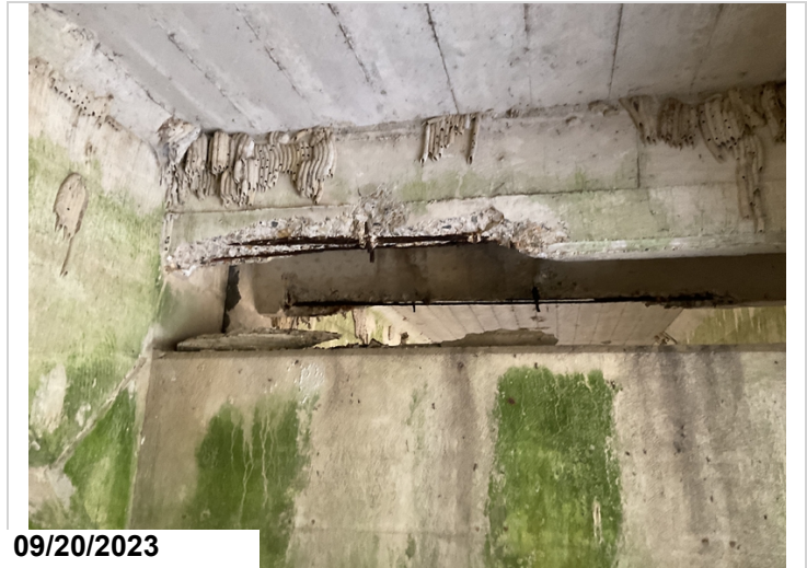
Bent 2: the concrete diaphragms are spalled with exposed rebar.
