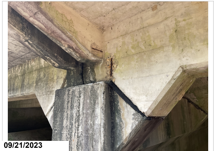
Span 1, girder 1, bent 2: left side of girder has spall with exposed rebar
