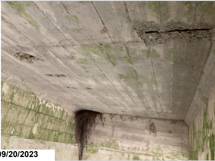
Span 2 soffit, between girders 3&4: small spalls with exposed rebar. The largest is 5"x13".
