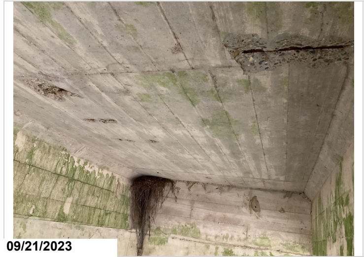
Span 2 soffit, between girders 3&4: small spalls with exposed rebar. The largest is 5"x13".
