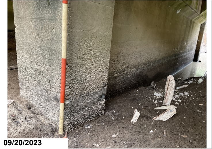
Bent 2, column 2: abrasion up to 3' from ground line typical to column 1 and pier wall.
