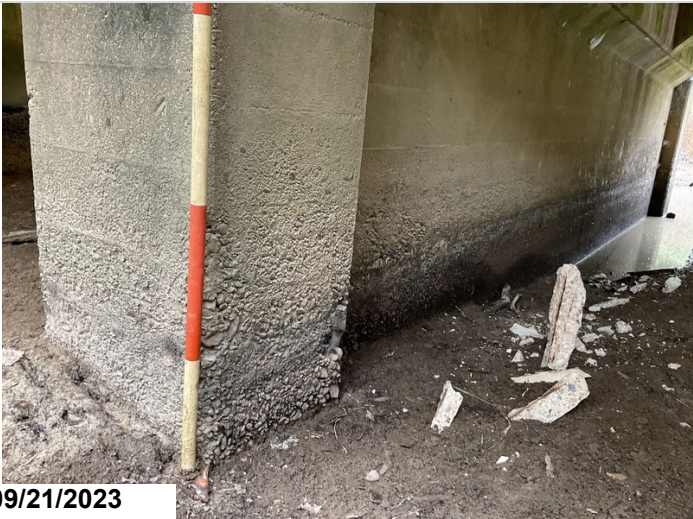
Bent 2, column 2: abrasion up to 3' from ground line typical to column 1 and pier wall.
