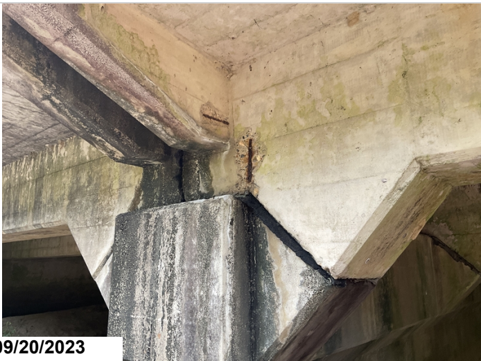
Span 1, girder 1, bent 2: left side of girder has spall with exposed rebar
