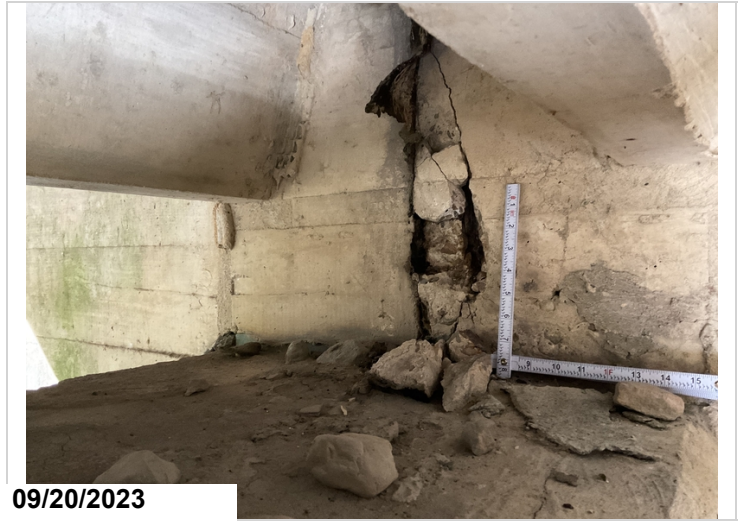
Bent 2, span 2, girder 2: spall with exposed rebar at the joint.
