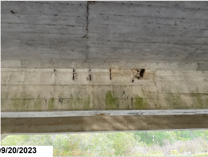
Span 2: right side of girder 2 small spalls with exposed rebar. Similar condition at girder 4.
