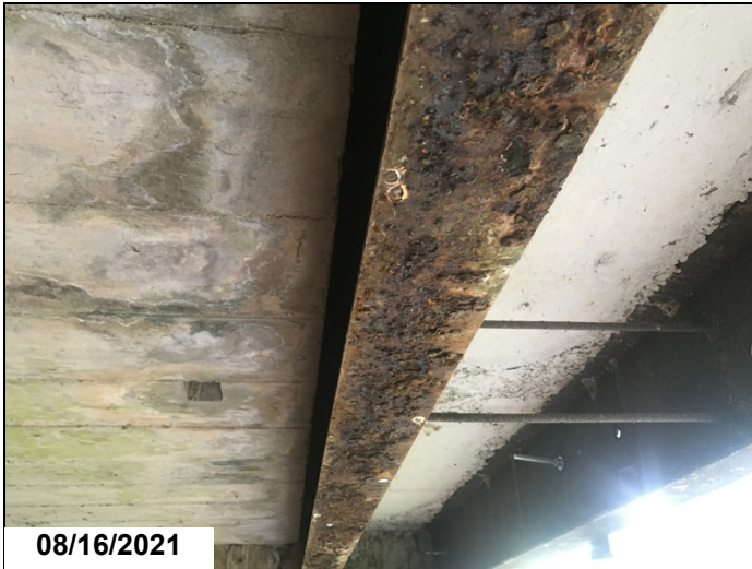
Beam 3 span 2 active corrosion with moderate pitting.
