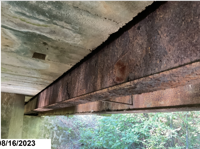
Beam 2: active rust with moderate pitting.
