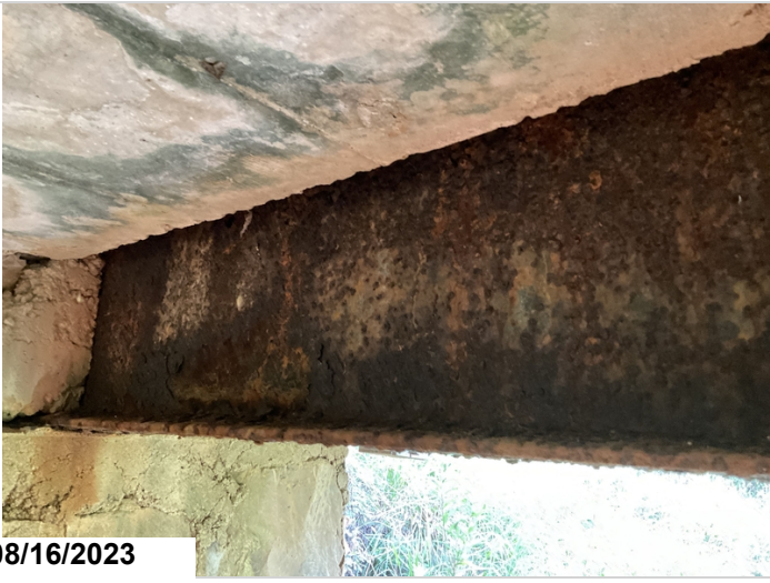
Beam 3: active rust with moderate pitting.
