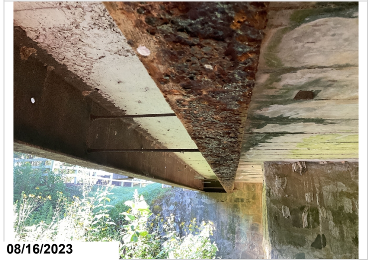
Beam 3: active rust with moderate pitting.
