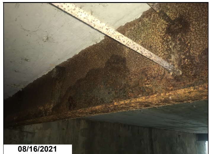
Span 2 beam 2 has active corrosion with pitting to bottom flange and web. Common beam 3.
