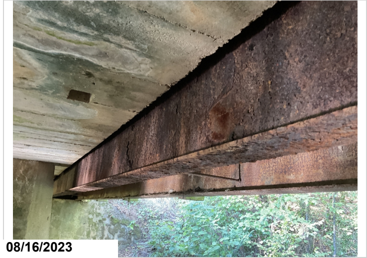
Beam 2: active rust with moderate pitting.
