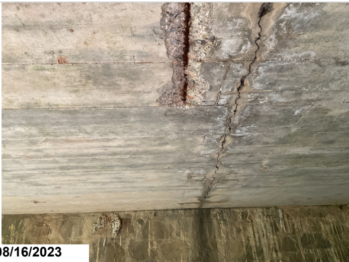
Span 1: spall with exposed rebar and crack in the soffit near center line
