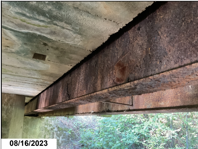
Beam 2: active rust with moderate pitting.
