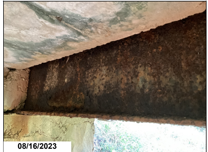
Beam 3: active rust with moderate pitting.
