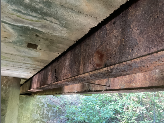
Beam 2: active rust with moderate pitting.
