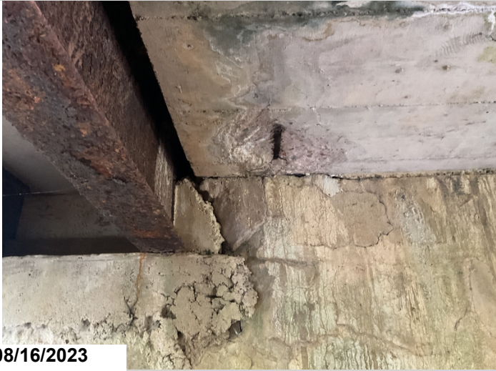
Span 2: small spall with exposed rebar in the soffit
