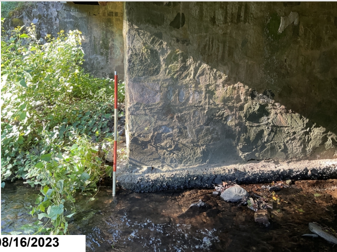
Bent 2: footing exposed and has minor undermining.
