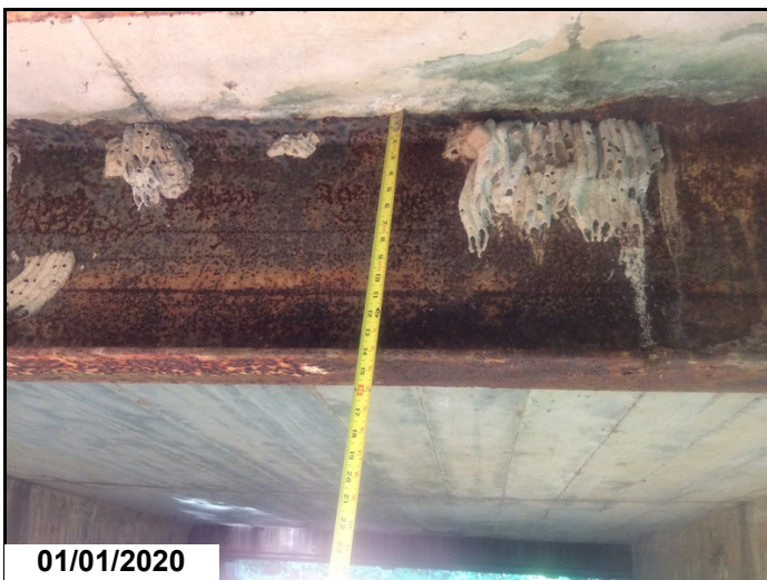
Active corrosion on all of beams.
