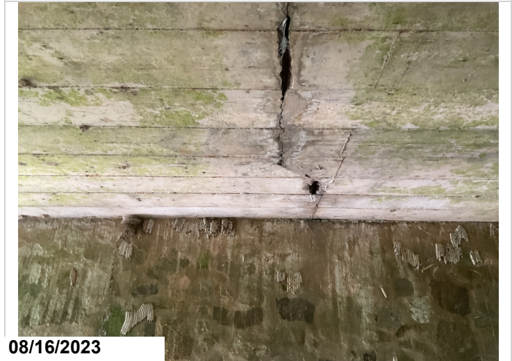
Span 2: crack at centerline with spall exposing rebar.
