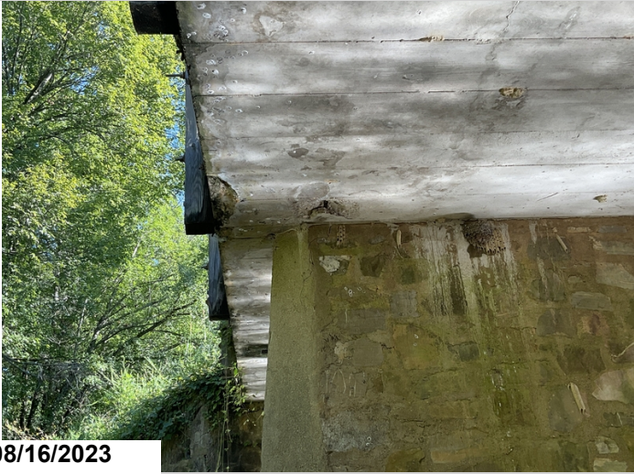
Span 1 at bent 2: couple small spalls in the slab.
