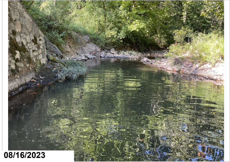
Channel looking upstream. The left embankment is beginning to erode.
