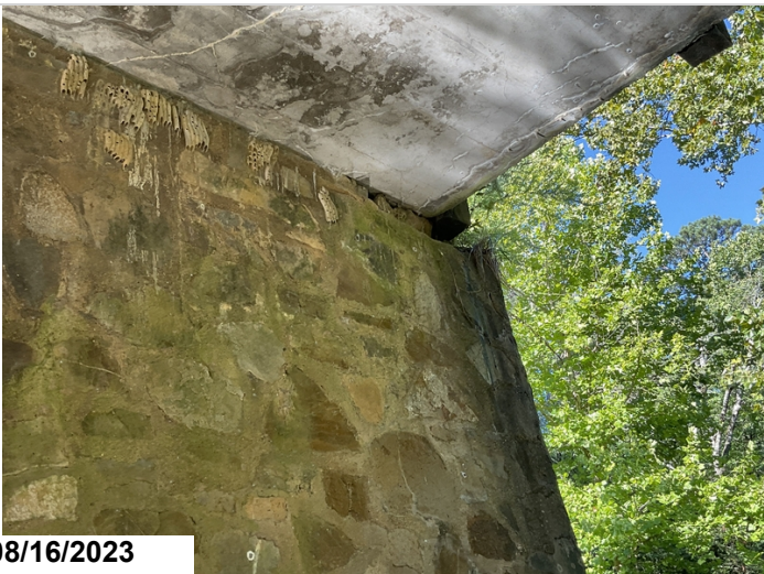
Bent 1: left side at the slab is missing some stone
