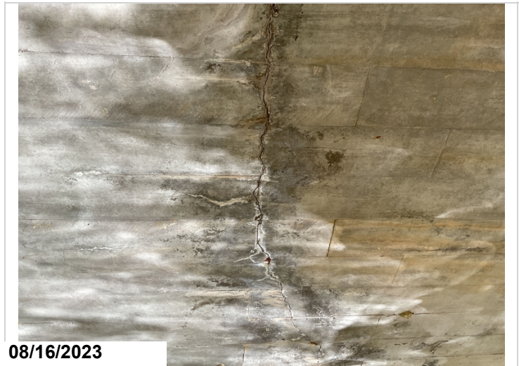
Span 1: soffit with a large longitudinal crack down the centerline.
