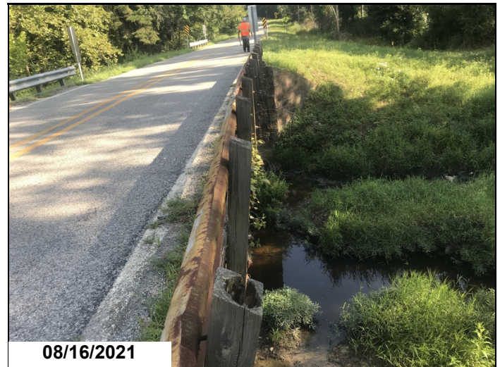
Wooden bridge rail posts are rotten and hollowing.
