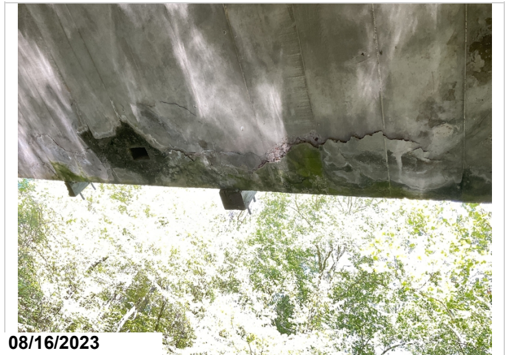
Span 2: left edge of slab has 9' delam.
