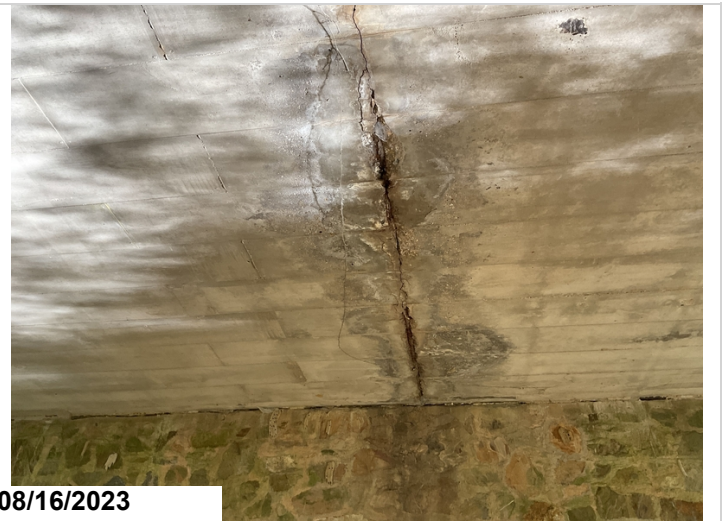
Span 1: large crack at center line.
