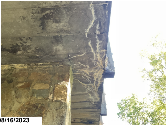
Spans 2&3: right side of slab is cracked with efflorescence staining
