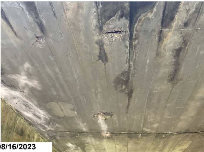
Span 3 multiple spalls to the soffit
