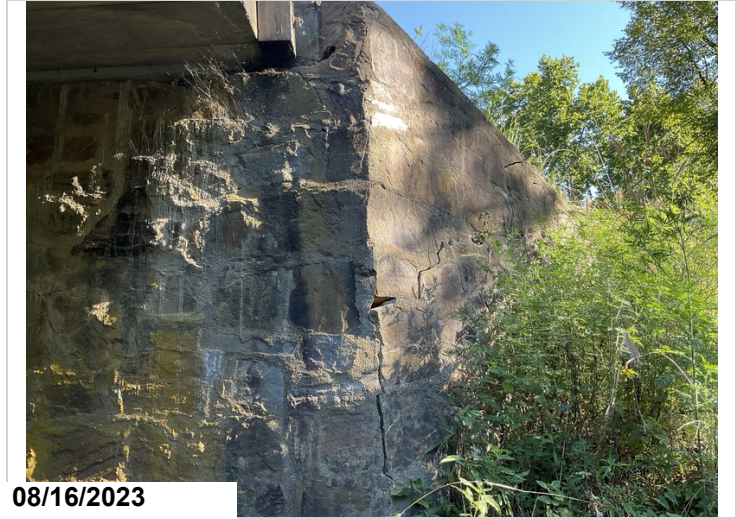
Bent 4: right wing wall is cracked.
