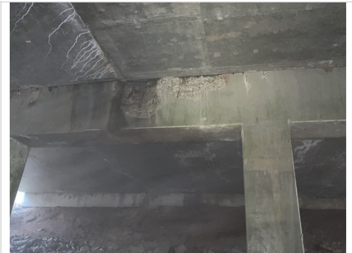
Ahead bent 2: cap has large spall with exposed rebar.
