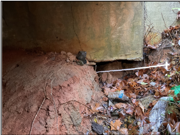
Bent 1: left end erosion has washed material out from under abutment exposing a steel pile. 2022
