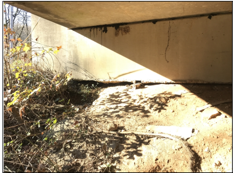
Bent 1 abutment right side undermined due to erosion.
