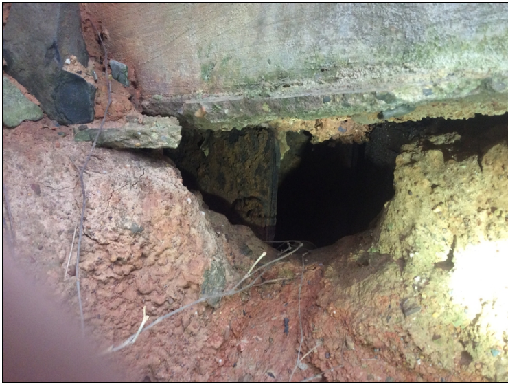
Bent 1, laminating rust on pile exposed due to erosion on the left side.
