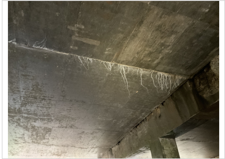
Span 2: soffit has longitudinal cracks with efflorescence staining at centerline.
