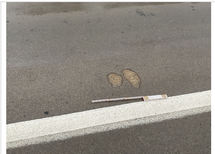
Span 3: the far right lane has couple of small areas where the polymer overlay has peeled away from the deck surface
