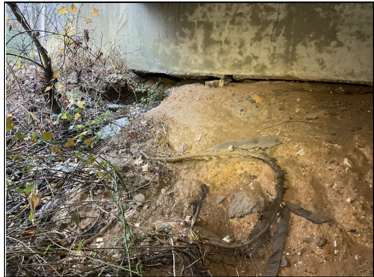
Bent 1: right end of abutment erosion has exposed pile under this bent. 2022
