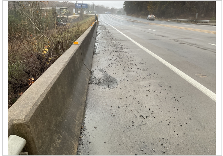
Both gutter lines are full of gravel
