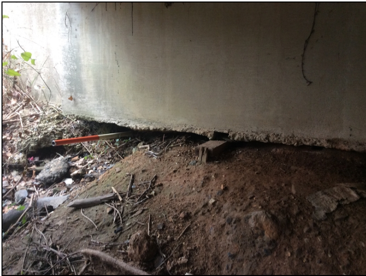
Bent 1 right side undermined due to erosion.
