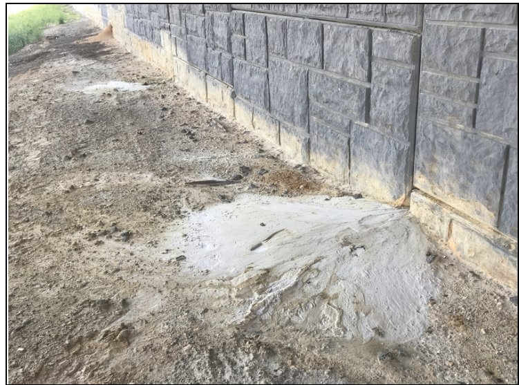
Abutment 2 is leaking dynafill at base of MSE wall.
