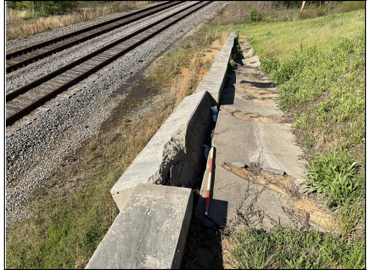
Bent 1, right side: top of MSE wall damaged due to collision.
