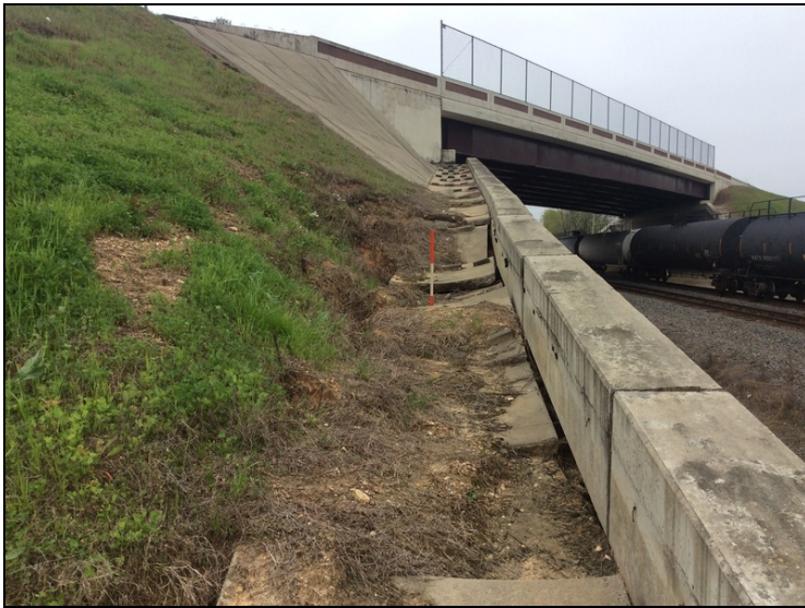
Ditch paving has failed at bent 2 left side. Approximately 35 ' has erosion and ditch paving has dropped 3'.
