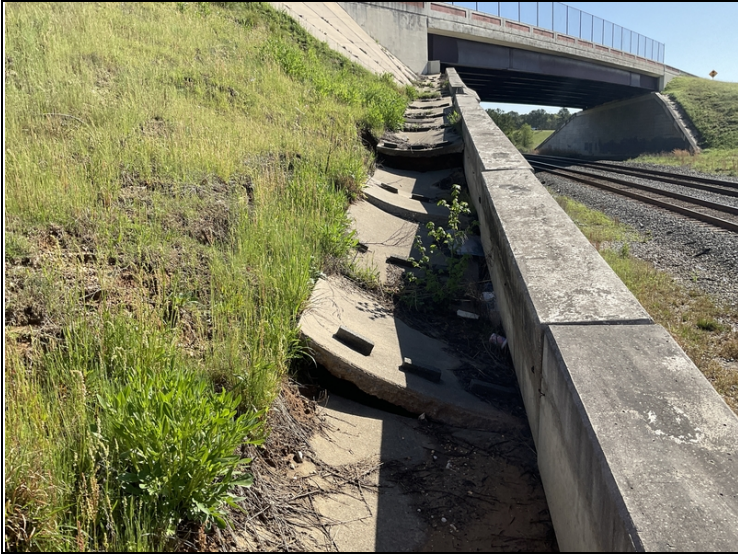
Bent 1, right side: slope paving is failing due to erosion.
