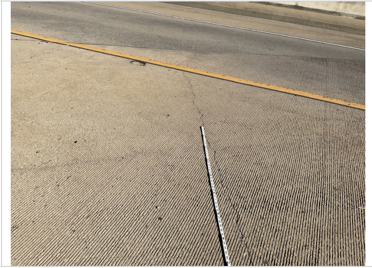
Large diagonal crack
