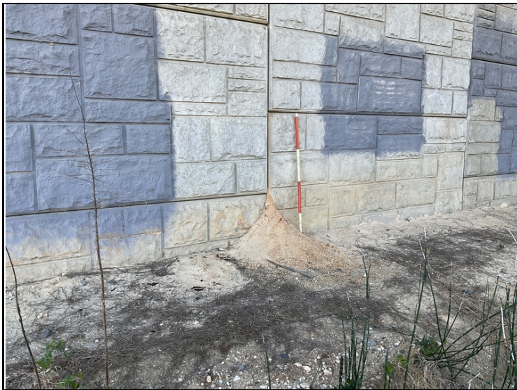
Bent 2: backfill material is leaking through the joint of the MSE wall. Under girder 3
