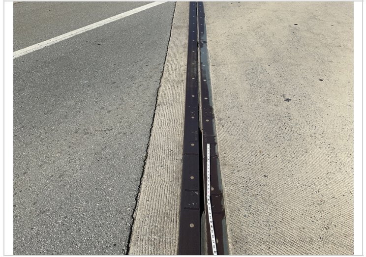
Bent 2, right lane: joint seal with a few holes allowing water to flow through.
