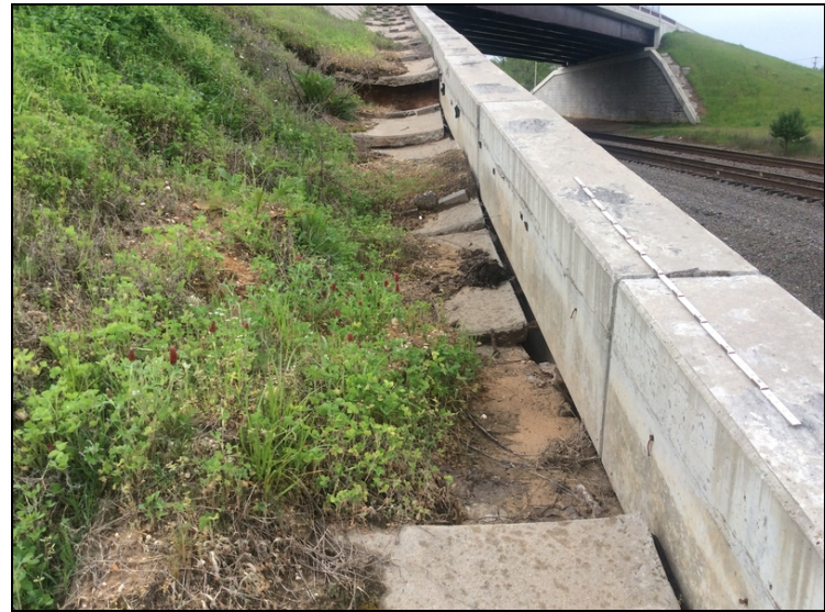
The ditch paving behind the MSE wall at Bent 2 on the left side has failed causing slope erosion and an MSE wall anchor strap is exposed. Photos attached.
