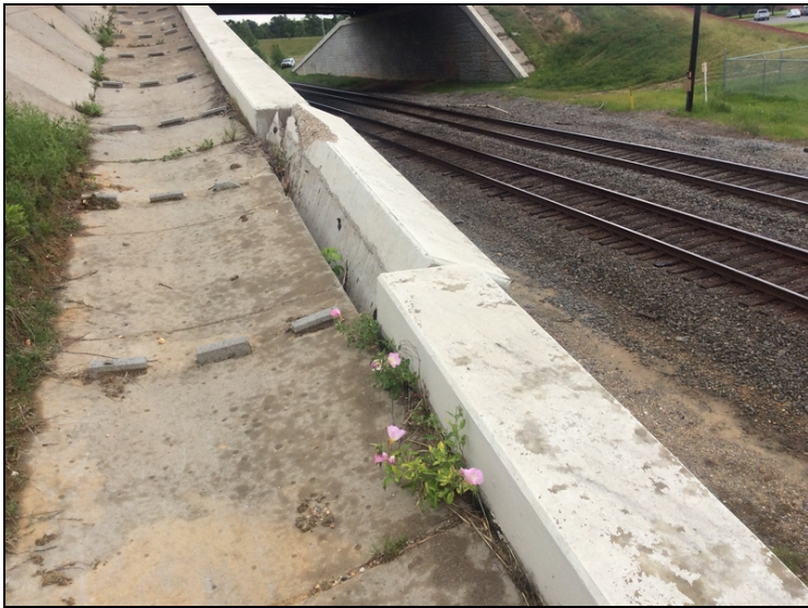
Bent 1 right side traffic impact to top of MSE wall
