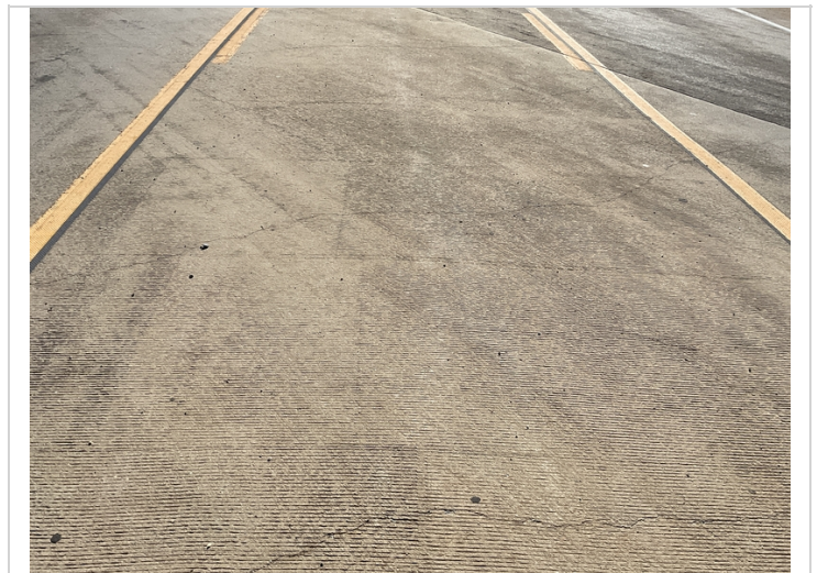
Sealed diagonal cracks
