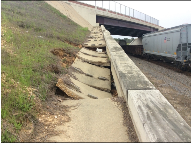
Ditch paving next to MSE wall at the right side of bent one has been undermined and 20' has collapsed.
