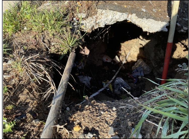
Bent 2, left side of the bridge a large void has been created at the end of the bridge railing near the side walk
