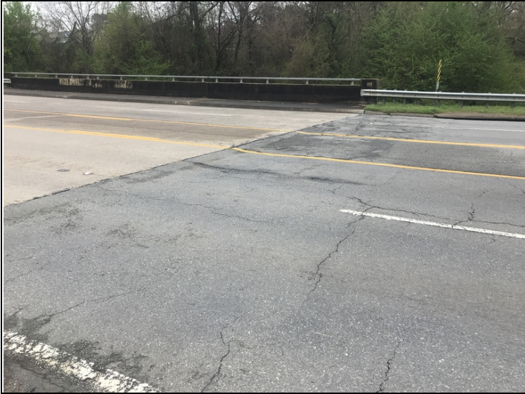
At bent 1 approach roadway has settled. 03/2020
