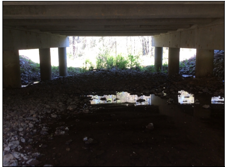
Downstream end of channel has build up of aggregation diverting stream flow to both bents 2 and 3.
