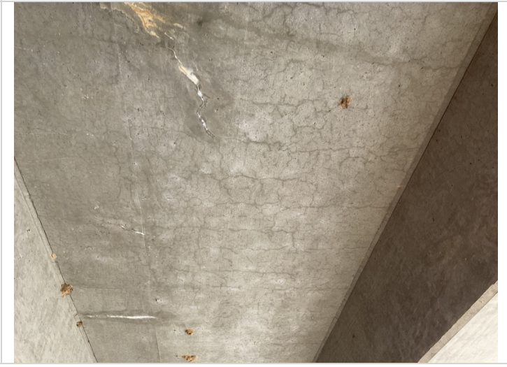
Map cracking in top flange
