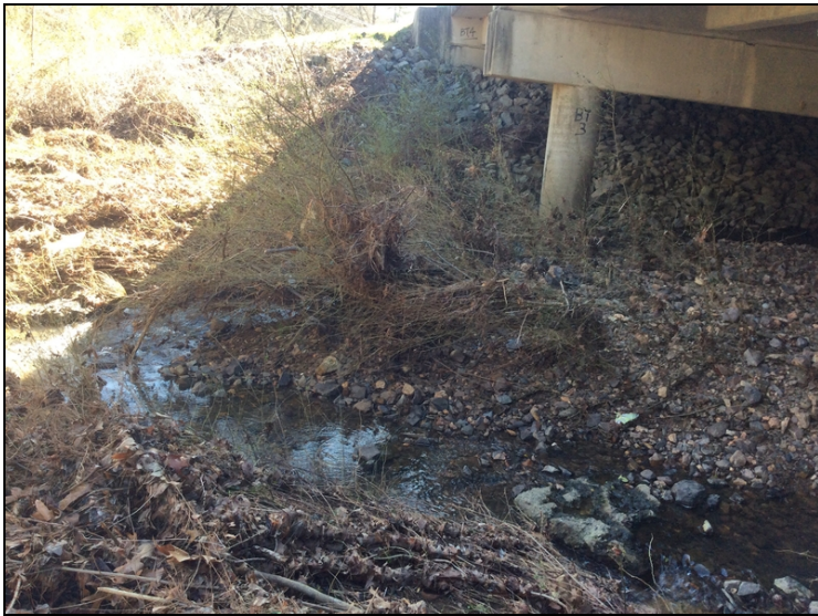
Channel between bents 2 and 3 the thalweg has split.
