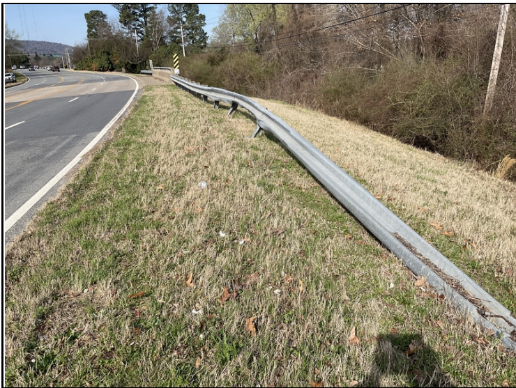
Guardrail damage at northeast end of the bridge
