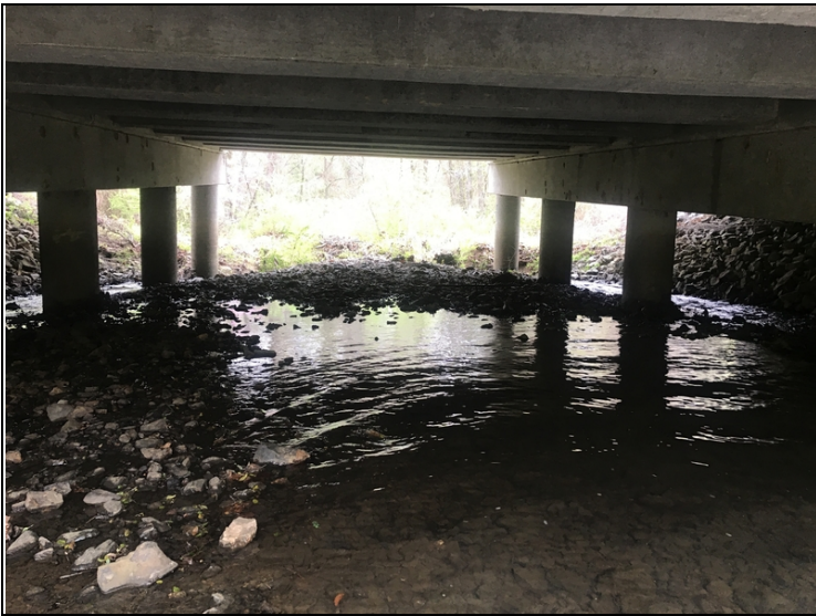
Downstream end of channel has build up of aggregation diverting stream flow to both bents 2 and 3. 03/2020
