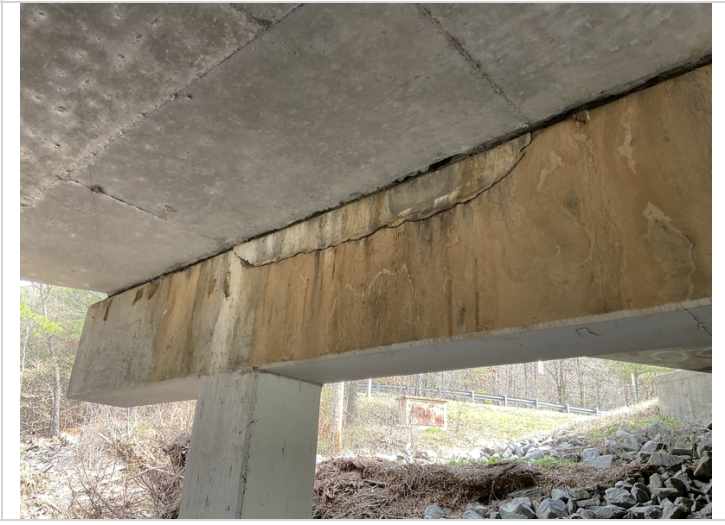
Delamination bent 3 backside
