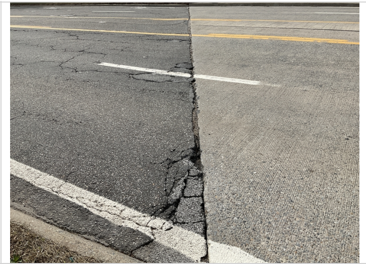
Potholes starting to form at east end of bridge
