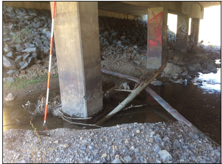
Bent 2 column 4 scour hole silted in covering top of footing. Horse scour at column at this time.
