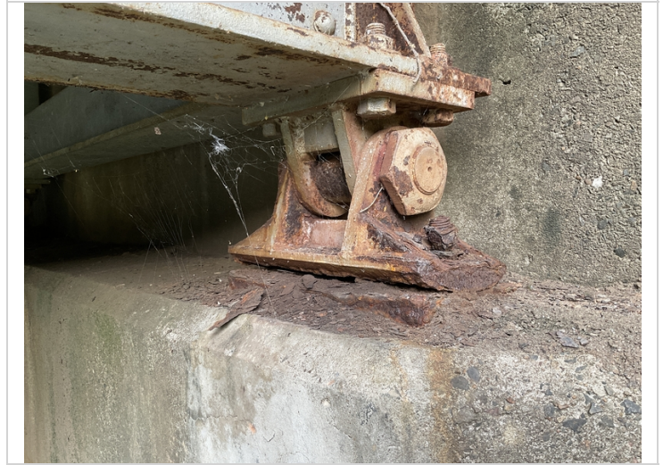
Bent 1, girder 1: bearing with section loss.
