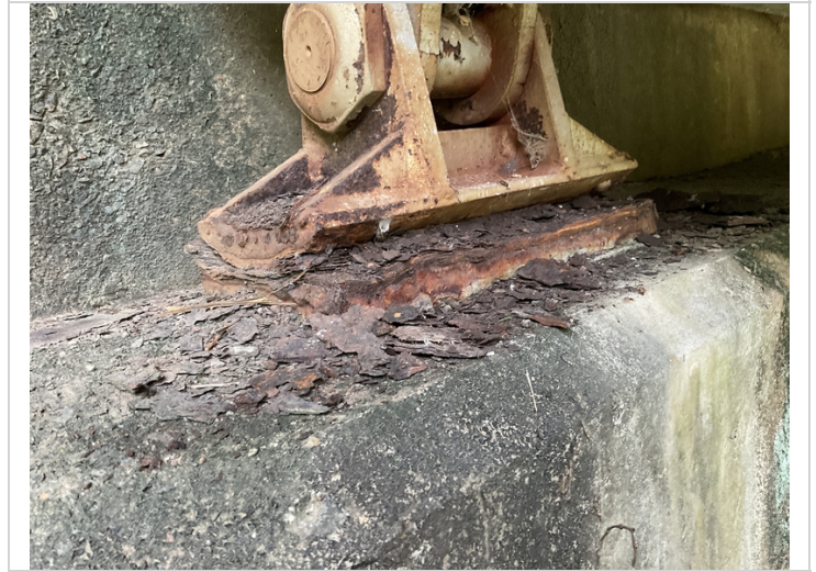
Bent 2: bearing with measurable section loss to the sole plate.
