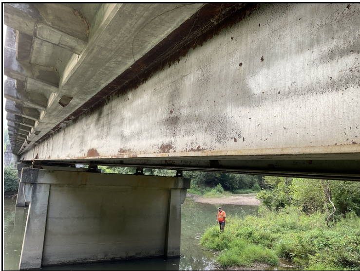
Span 1, girder 1: Typical condition of the paint condition on the girders.
