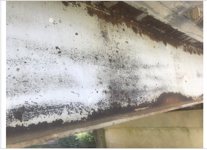
Span 2 beam 4 surface rust with minor pitting. Common all beams.
