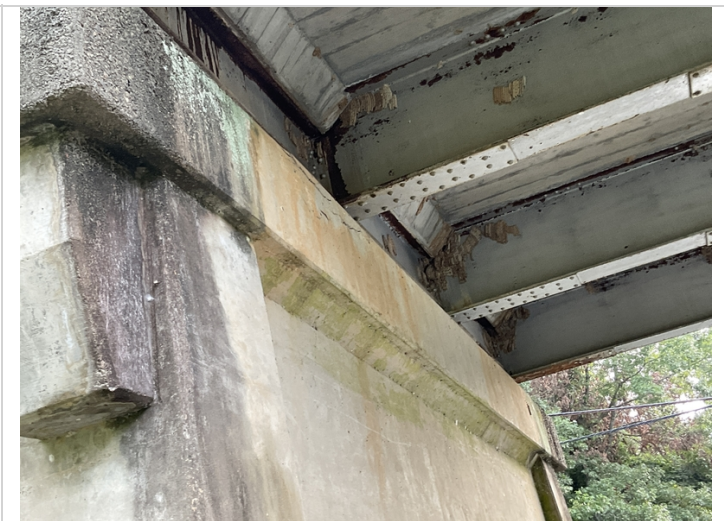
Bent 2: ahead side of cap has delma between beams 3&4.
