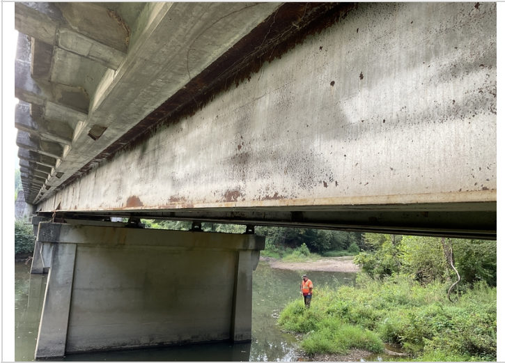
Span 1, girder 1: Typical condition of the paint condition on the girders.
