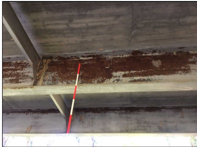
Span 1 beam 3 surface rust with light to moderate pitting. Common on all beams.
