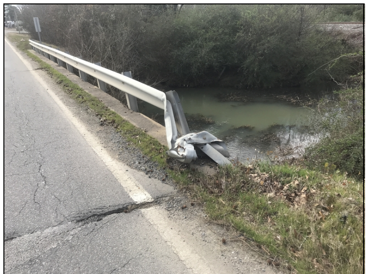
Right guardrail has collision damage
