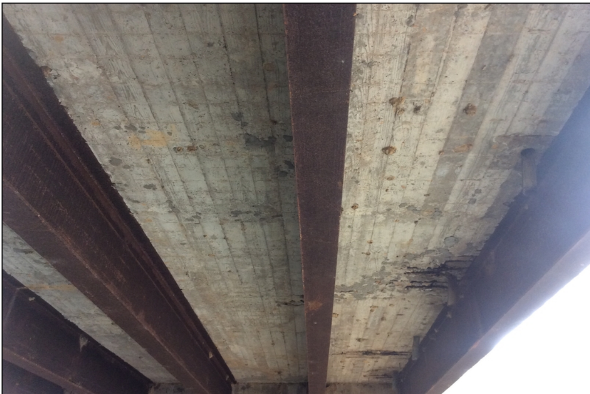
Soffit has spalls with exposed rebar at span 2 between beams 7&8.
