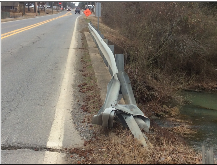
Right guardrail has collision damage.
