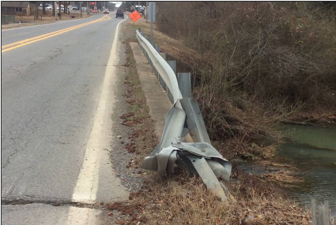
Right guardrail has collision damage.
