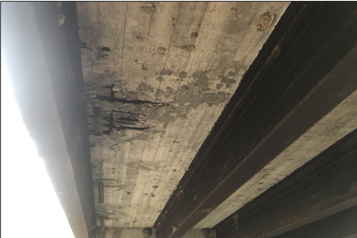
Span 2, between beams 7 & 8: large spall in soffit with exposed steel. Multiple locations with similar spalls.
