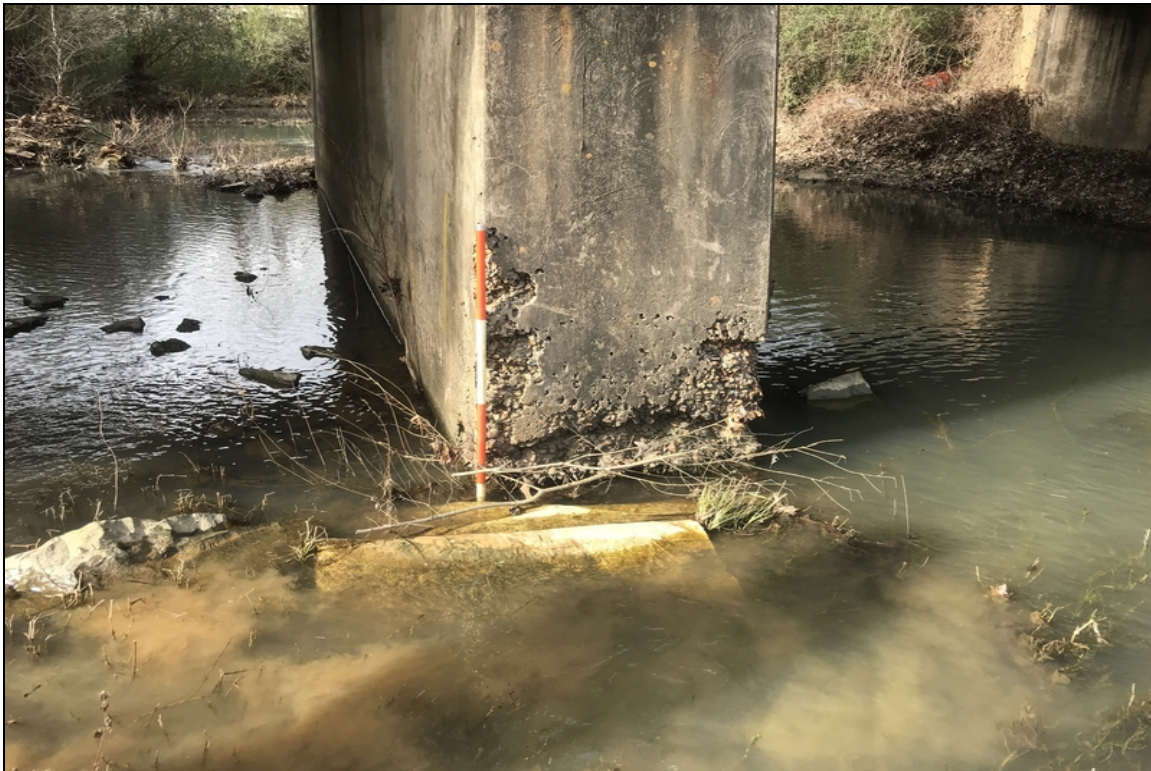
Bent 2, left end with severe abrasion exposing reinforcing steel
