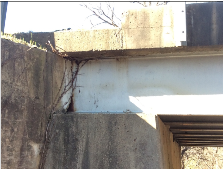
Bent 2, beam 1 Active rust with minor pitting at the end.
