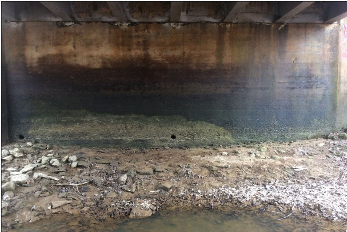
Abrasion at bent 2 abutment.
