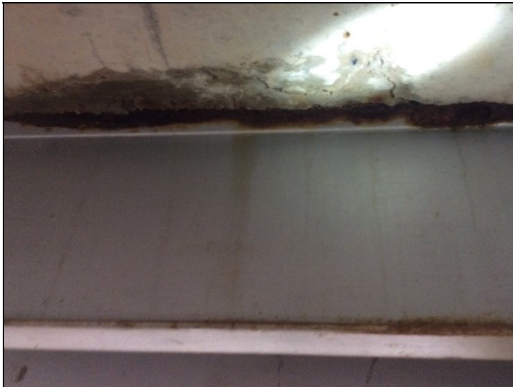
Beam 6 back from bent 2 active rust with moderate pitting on the upper flange. Common at bent 1.
