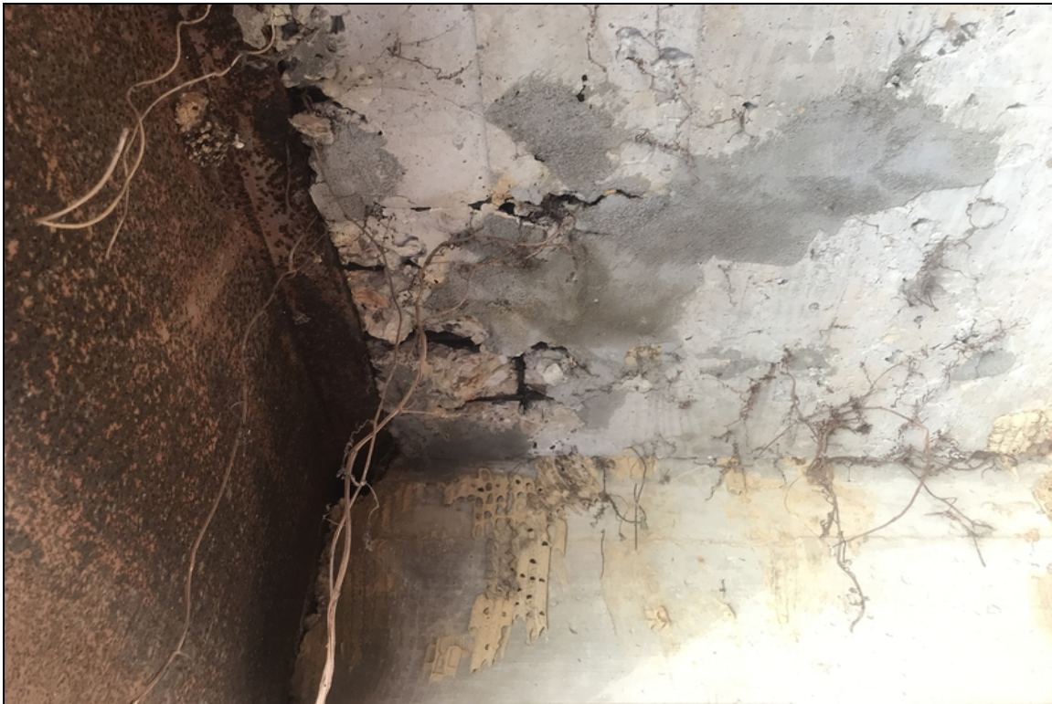
Soffit near bent 2 between beams 1 & 2 with patched area beginning to deteriorate and spall exposing reinforcing steel.
