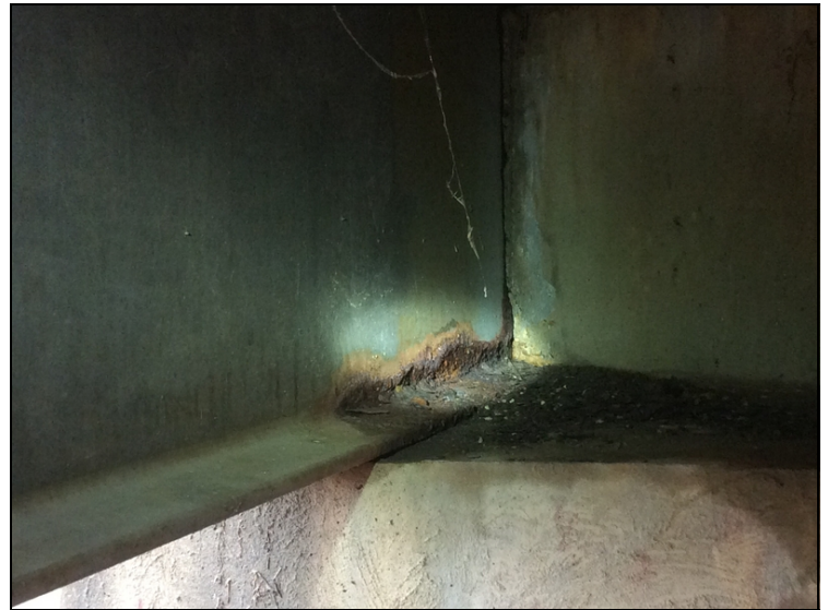
Bent 1 beam 9 has active rust with pitting on lower web and flange common beam 8.
