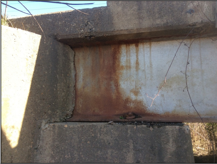
Bent 1, beam 9 Corrosion with pitting.
