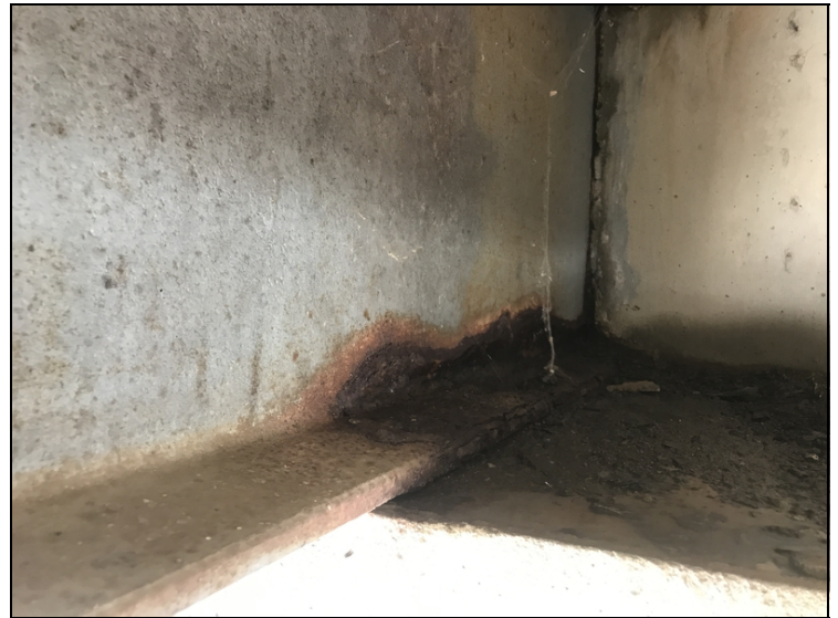
Bent 1, beam 9: measurable section loss to the lower web and bottom flange up to 2 foot from the end of the beam.
