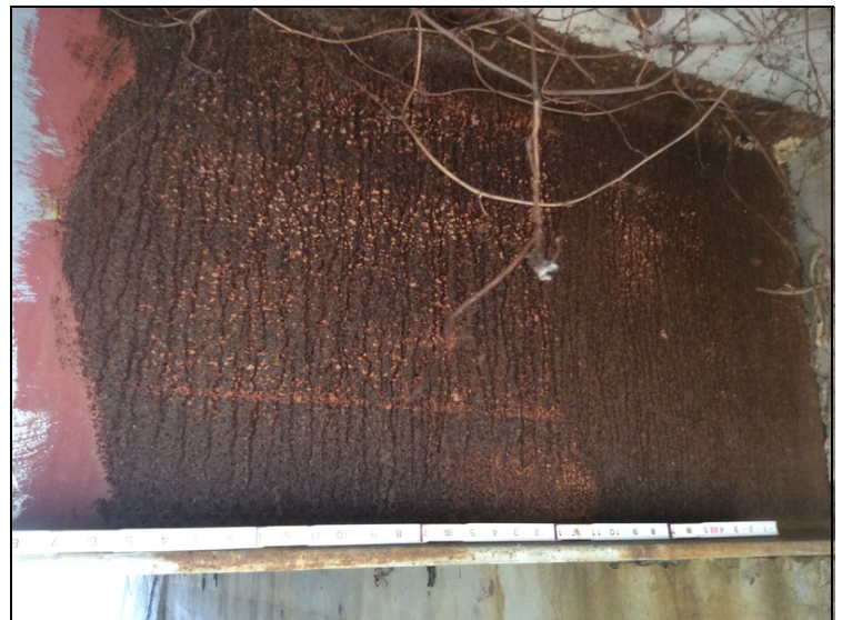
Bent 1, beam 2 Surface rust. Beam 1 similar.
