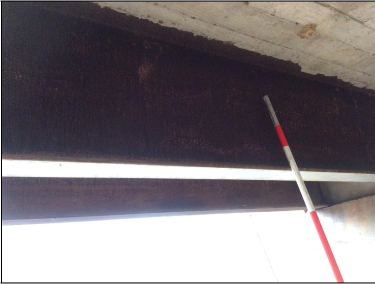
Beams 1&2 have active surface rust.
