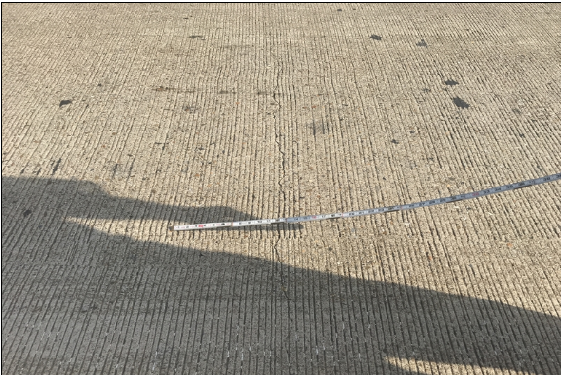
Deck span 2 has transverse cracks.
