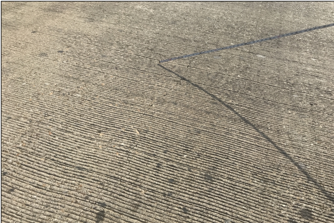
Deck span 3 has longitudinal crack.
