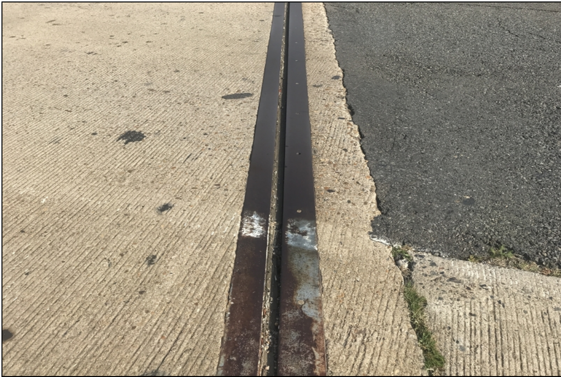
Bent 4 joint seal has lost bond and is leaking.
