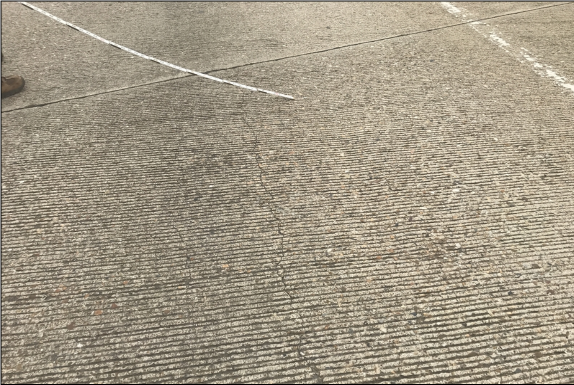
Deck span 3 has longitudinal cracks.
