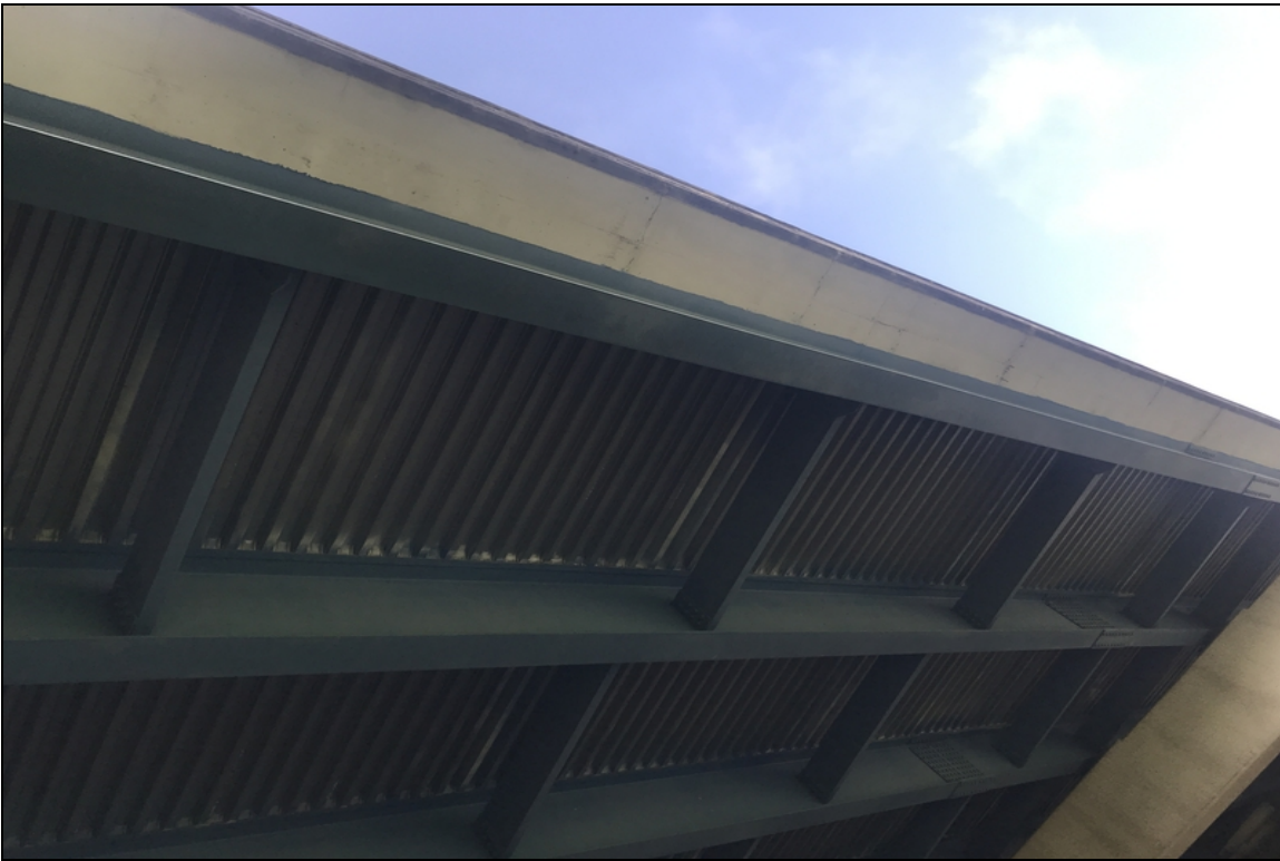
Span 2 left side soffit overhang has cracks with efflorescence.
