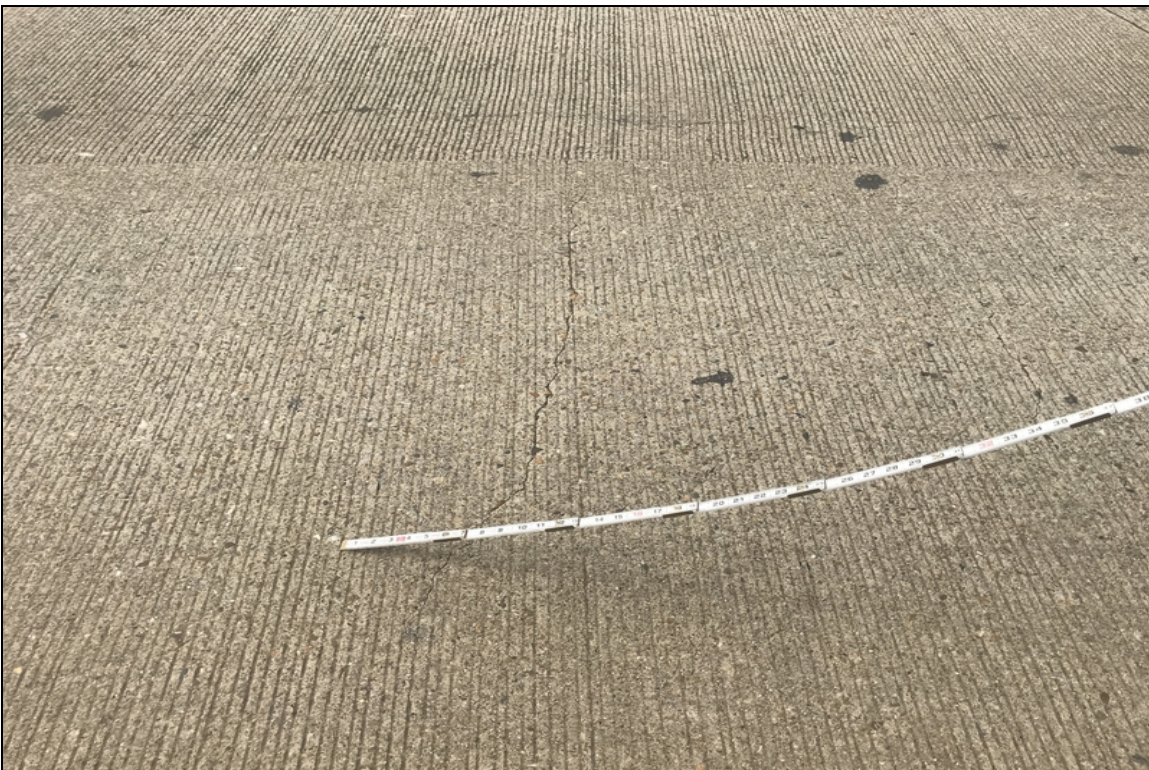
Deck span 1 has transverse cracks.
