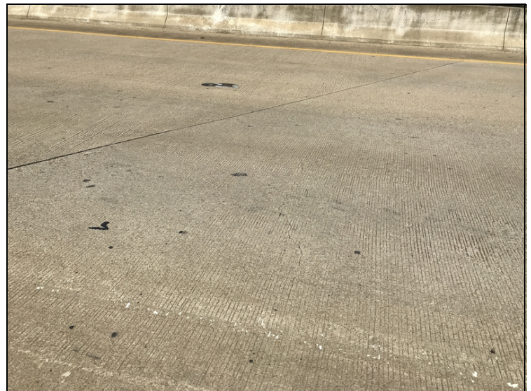
Large transverse cracks.
