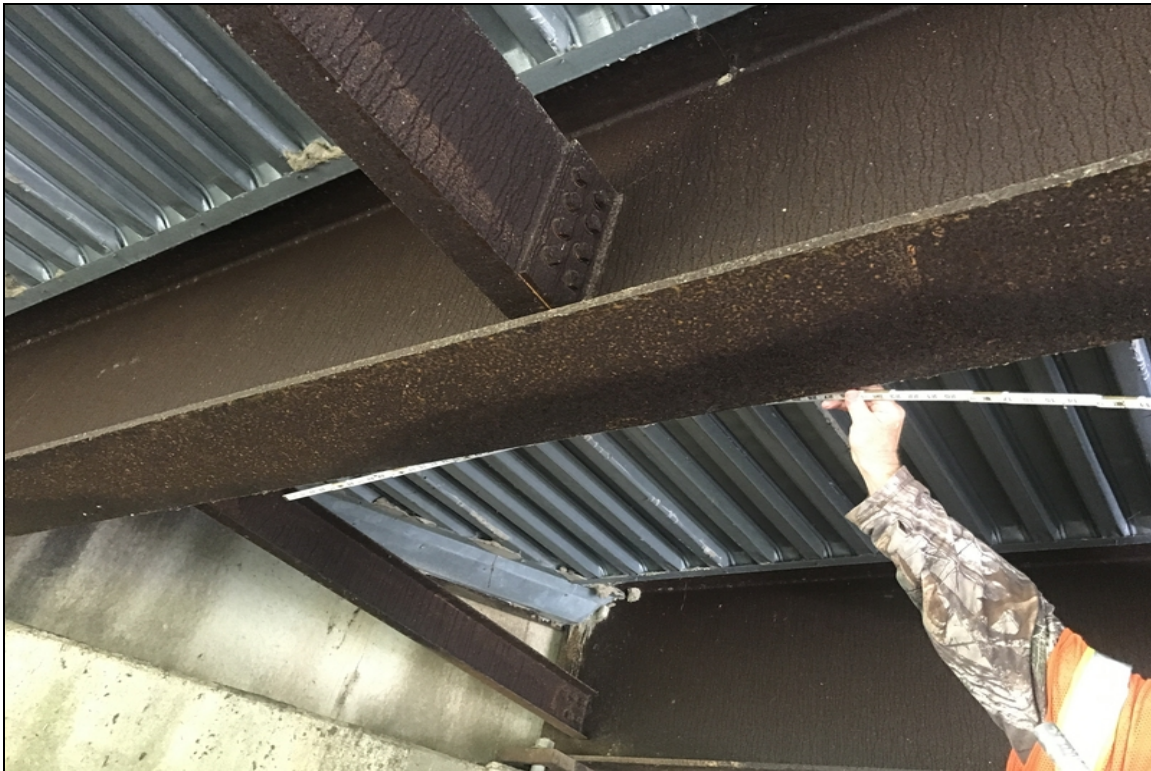
Span 1 beam 3 has flaking rust to bottom flange.
