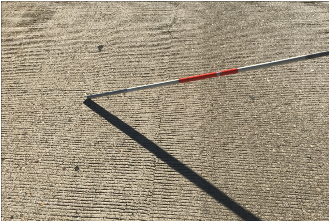
Unsealed longitudinal cracks in decal at span 2.
