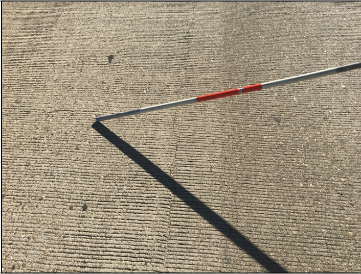
Unsealed longitudinal cracks in decal at span 2.
