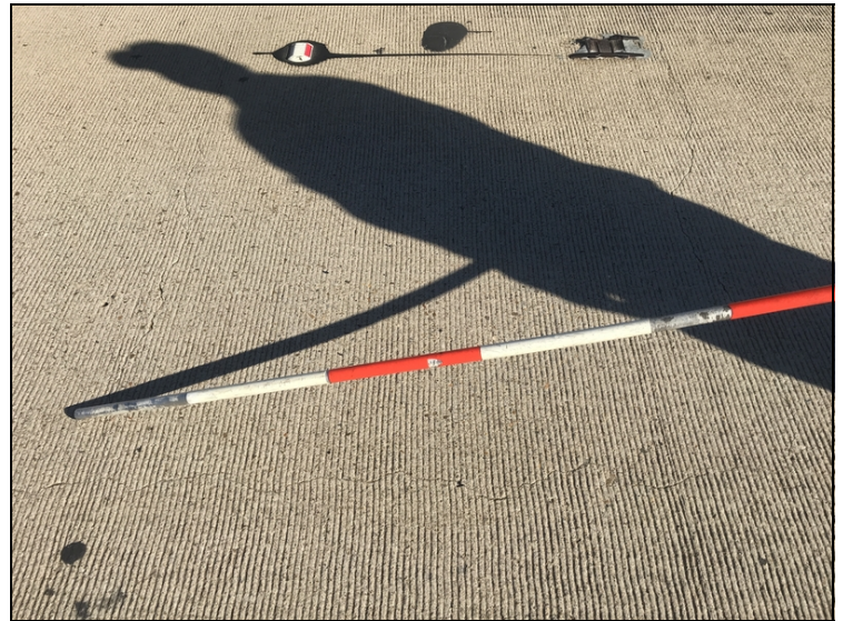
Unsealed transverse cracks in deck at span 5.
