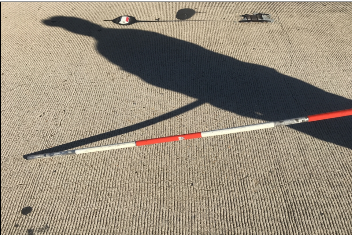
Unsealed transverse cracks in deck at span 5.
