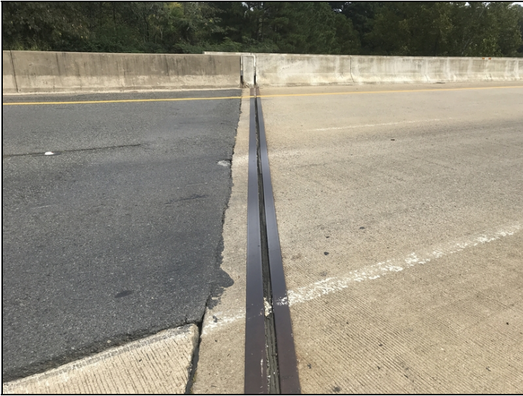
Bent 1 joint has lost adhesion.
