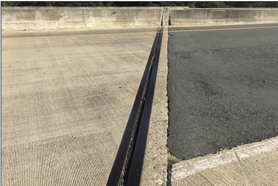
Joint seal at bent 6 has lost bond and is leaking.
