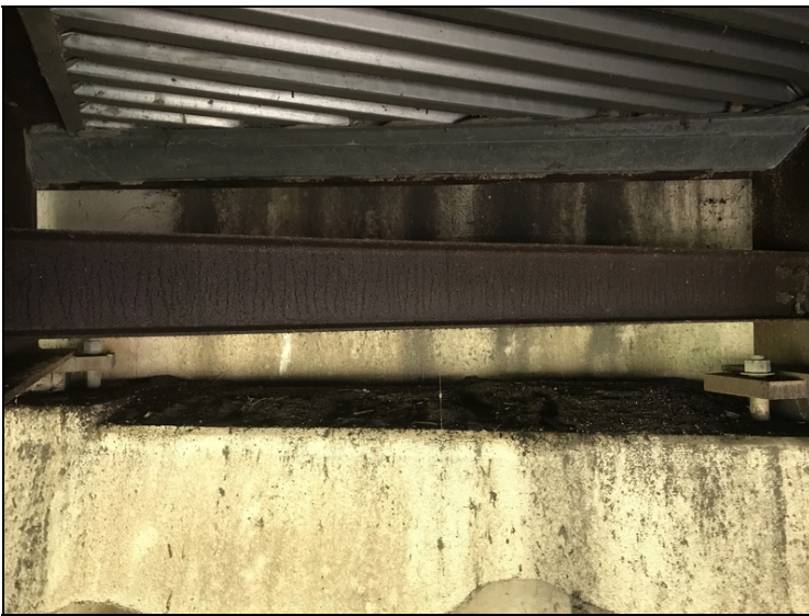
Bent 6 bay 3 debris on top of cap.
