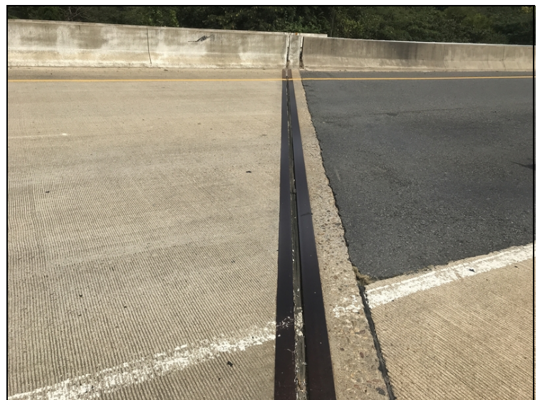
Bent 6 joint has lost adhesion and is leaking.
