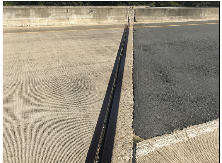
Joint seal at bent 6 has lost bond and is leaking.
