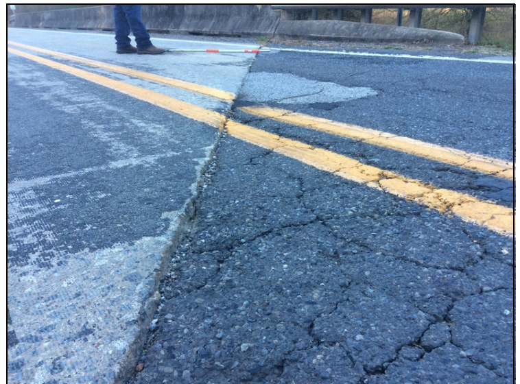
Approach roadway has settled at the west end of the bridge.
