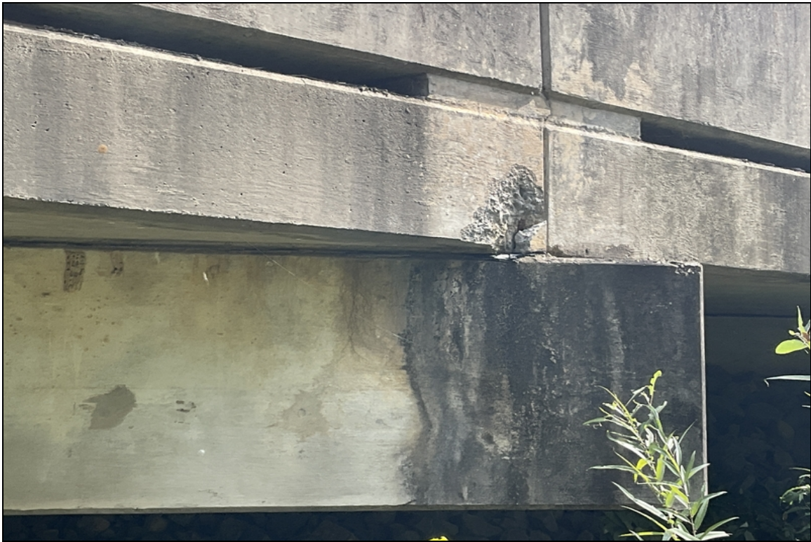
Spall on left side of span 2 at bent 2.
