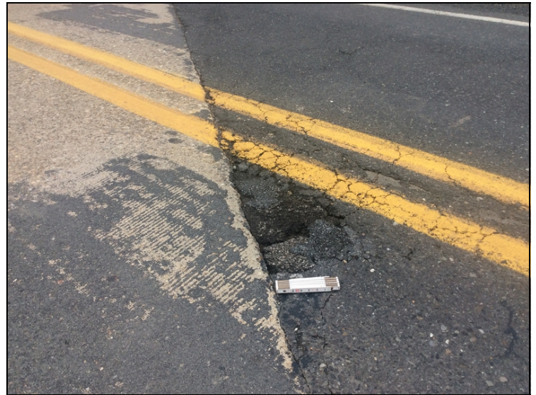
East end, failing patch in approach roadway.
