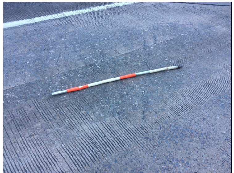
Span 2, unsealed cracks perpendicular to the skew, up to 0.050".
