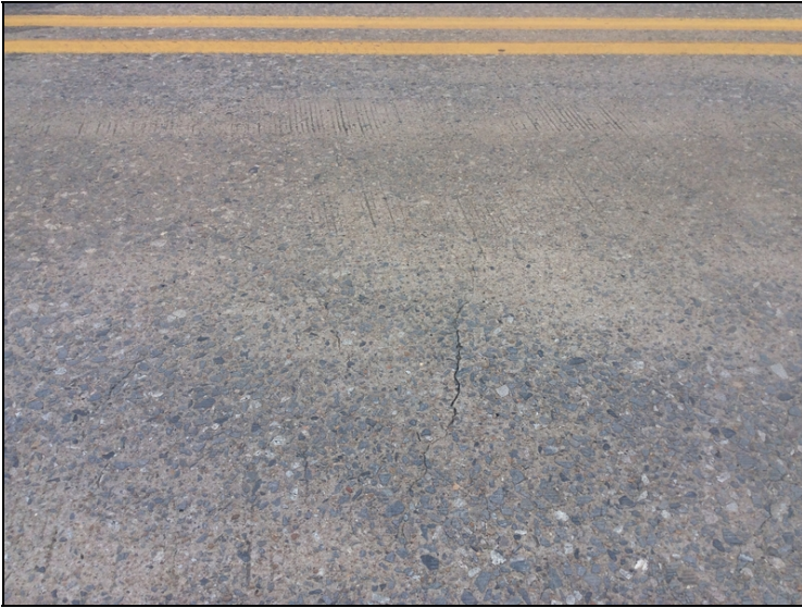
Large transverse crack Span 3.
