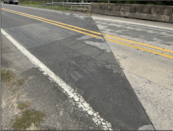
West end of bridge, settled with small potholes.
