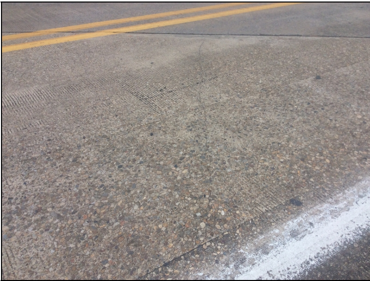
Span 1, large diagonal crack.
