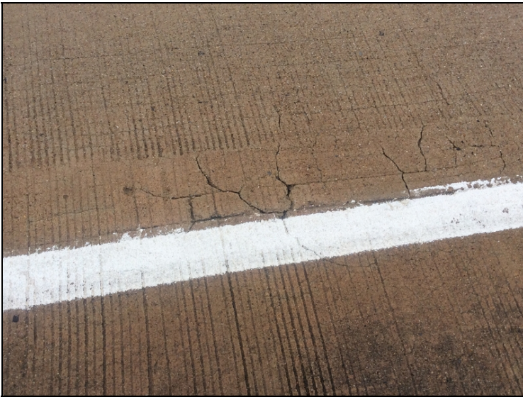
Deck cracks
