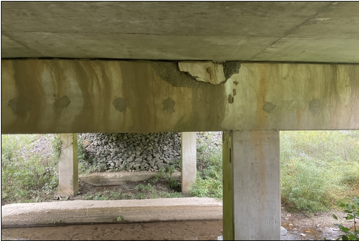
Spall on back side of Bent 2 cap
