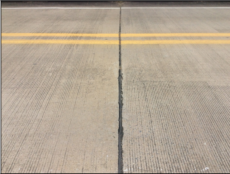
Bent 2 joint leaking due to lost adhesion.
