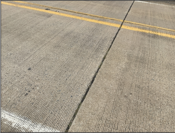
Bent 2 joint seal has lost adhesion
