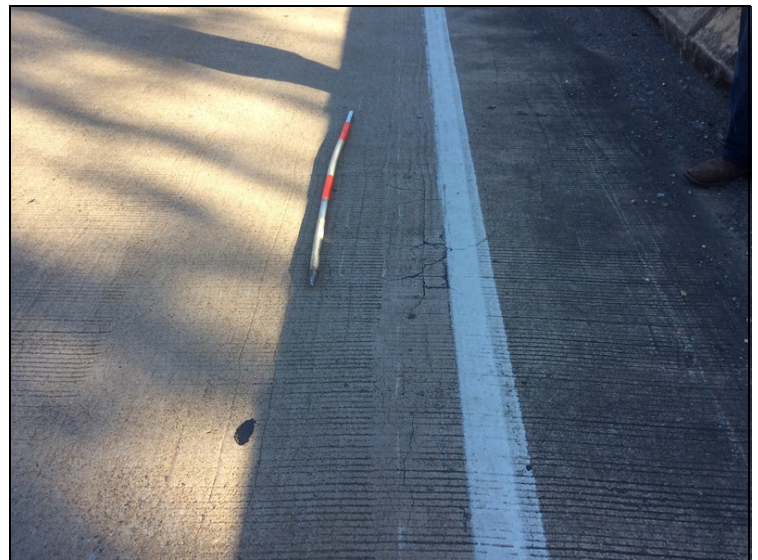
Span 3, unsealed map cracking.
