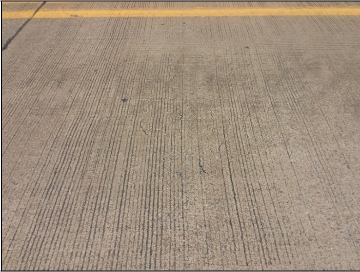
Span 3, large transverse cracks.
