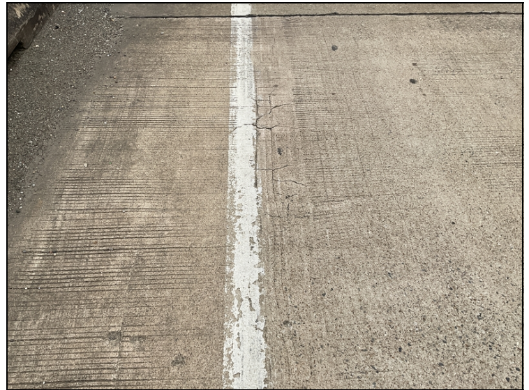
Span 3 right side unsealed map cracking.
