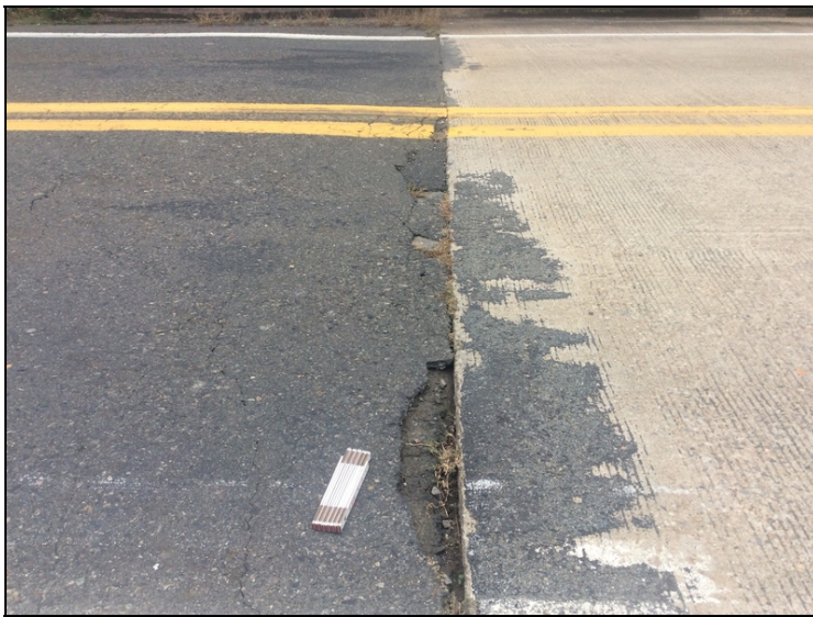
East end of bridge, pothole and patches.
