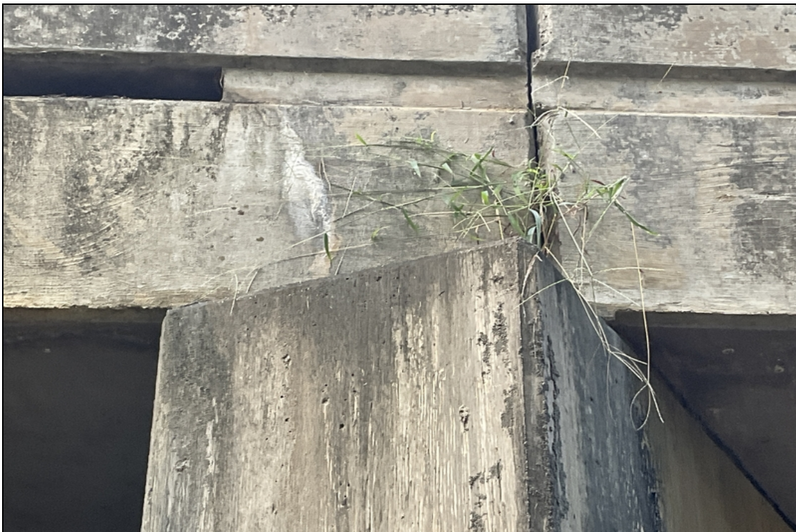
Slab right side at bent 2 vertical crack with light efflorescence.
