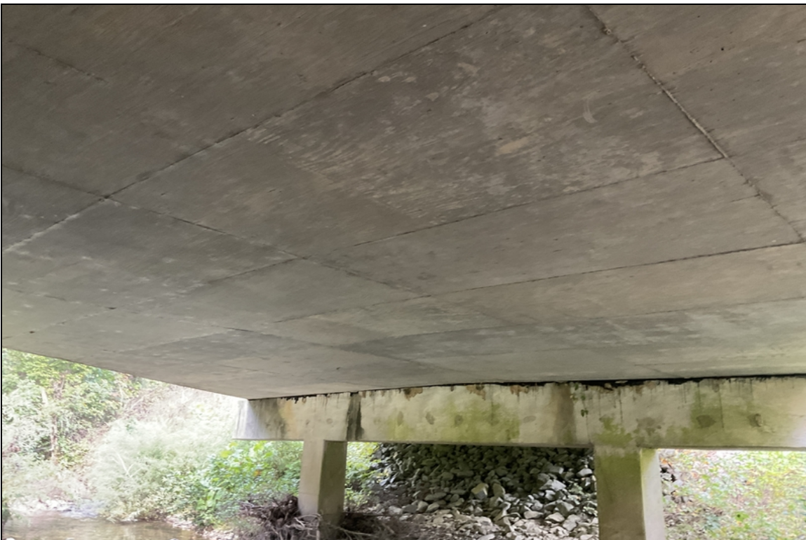
Span 2 soffit no sign of distress. Common all spans.
