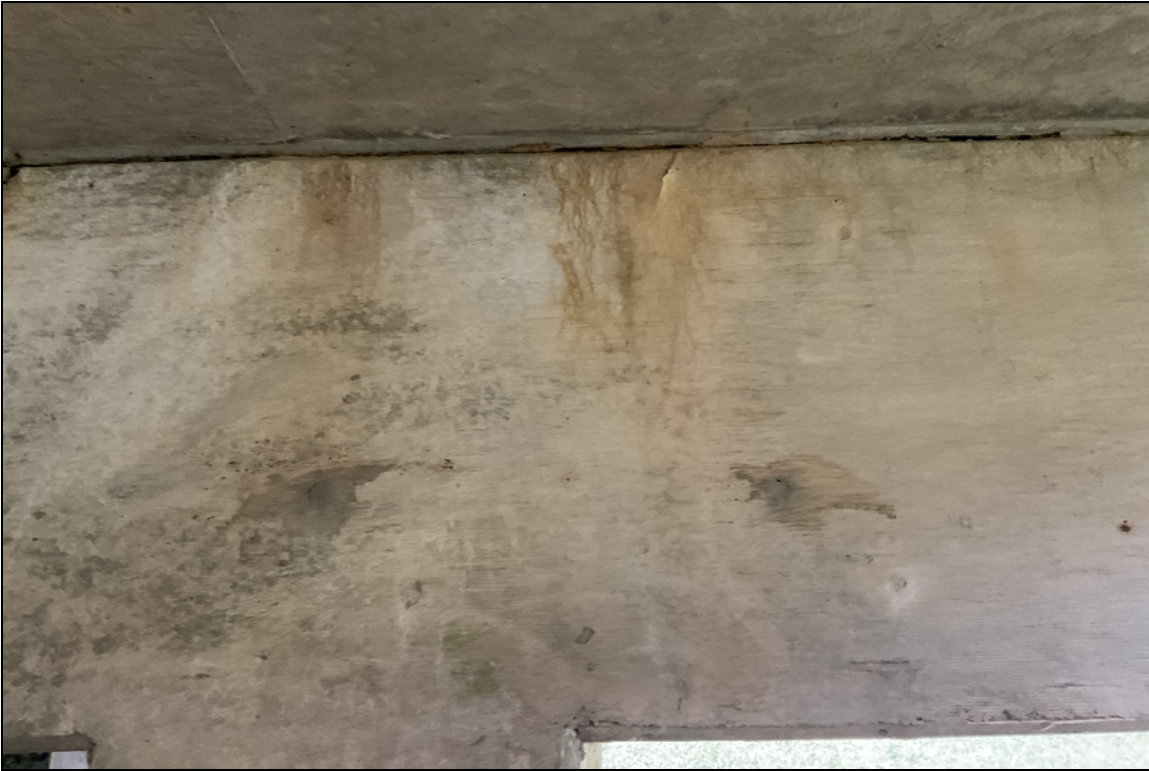
Bent 2 cap ahead crack with minor efflorescence.
