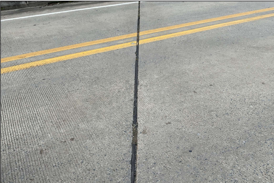
Bent 2 joint seal has lost bond.
