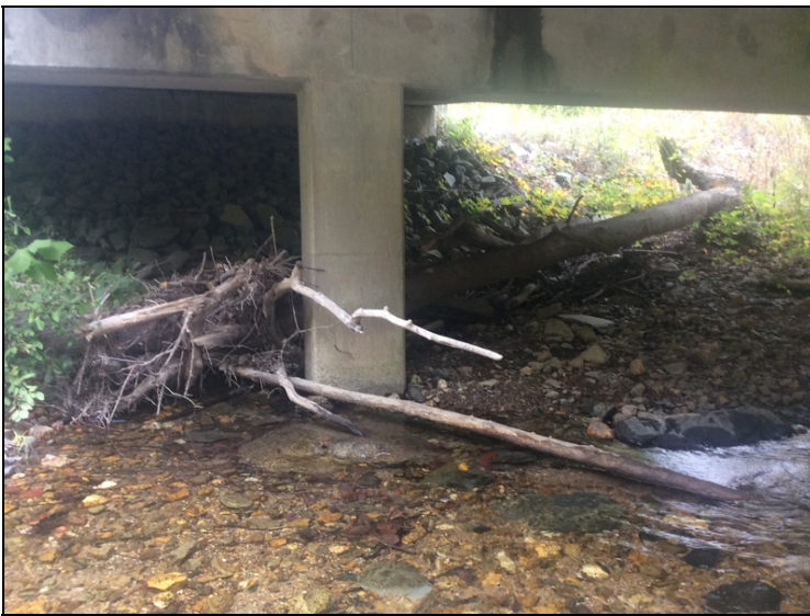
Bent 3, span 3, large tree and debris against column 1.
