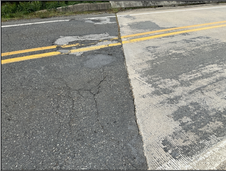
Bent 1, approach roadway has settled.
