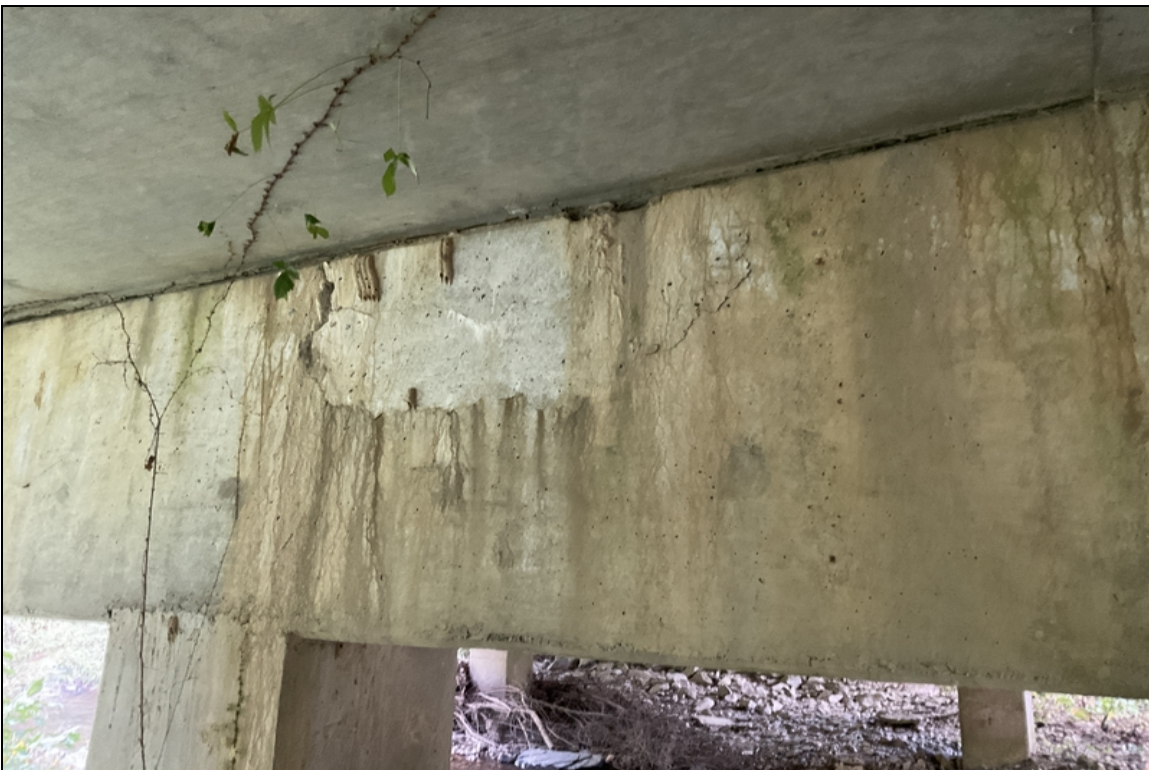
Bent 2 cap back at column 2 delam.
