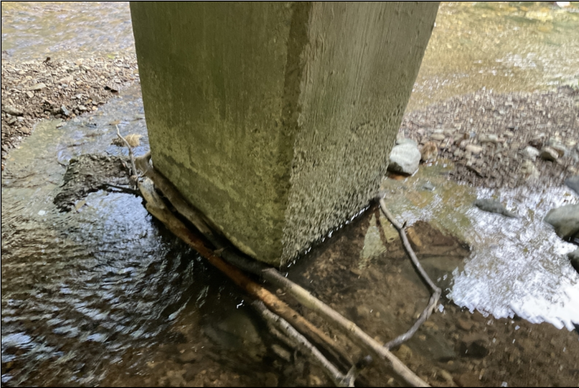
Bent 2 column 1 minor abrasion.
