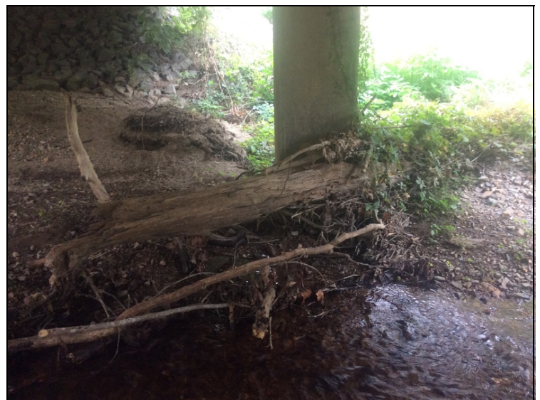
Bent 2, debris laying against column 1.
