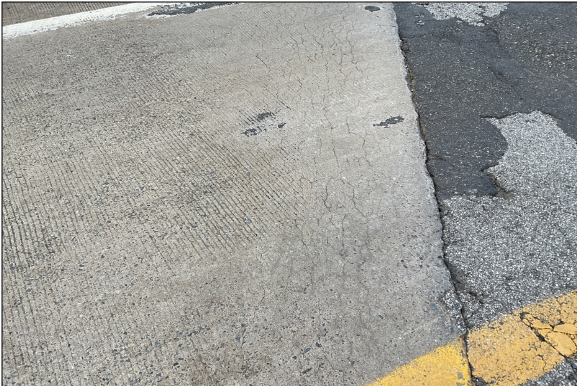
Span 3 deck map cracks. Worst case this bridge.
