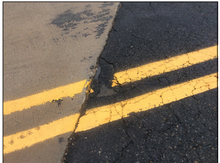
Approach roadway has settled and has small potholes
