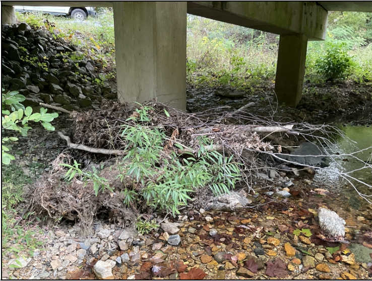
Debris at bent 3 column.
