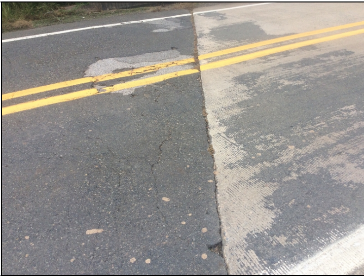
Bent 1, approach roadway has settled.
