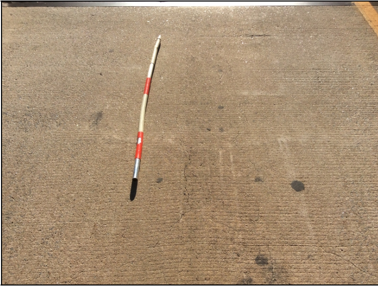
Span 2 unsealed cracks in deck up to 0.020"
