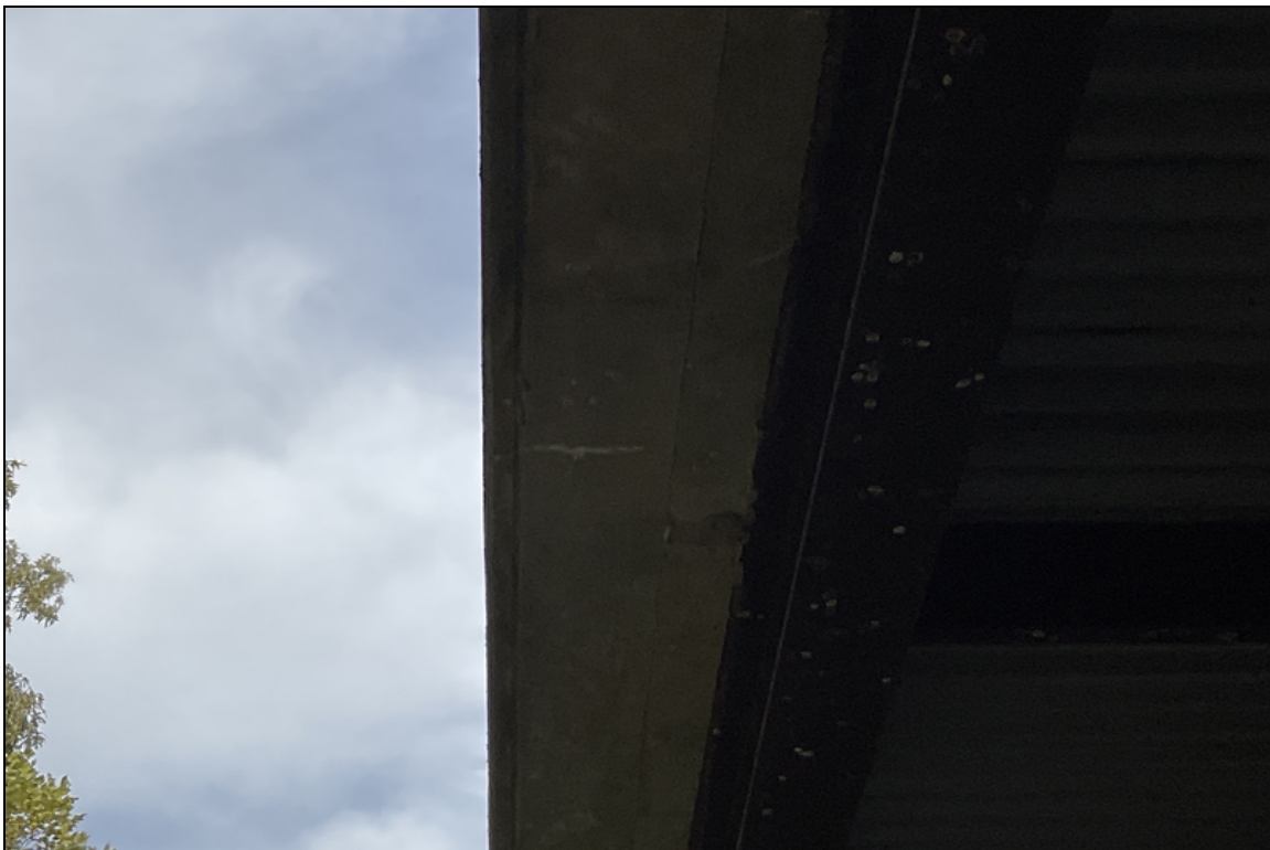
Soffit overhang span 2 left side crack with efflorescence.
