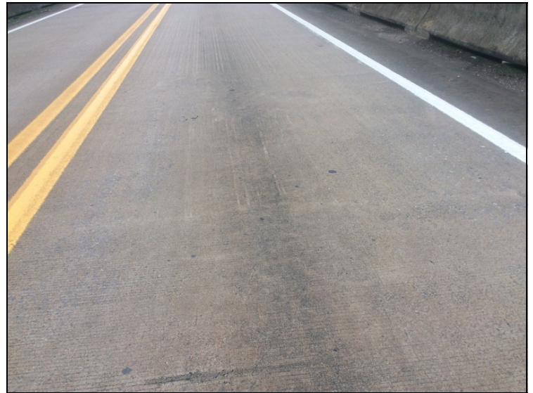
Span 2, longitudinal cracks.
