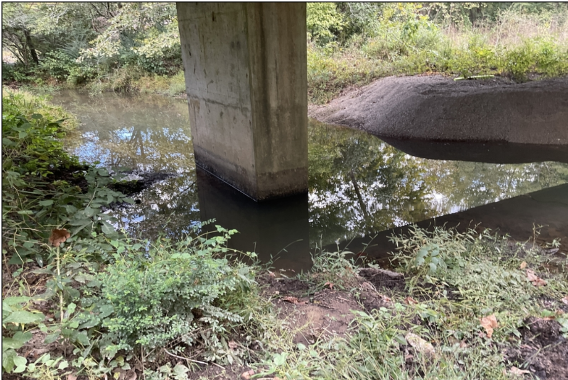
Local scour at bent 4 column.
