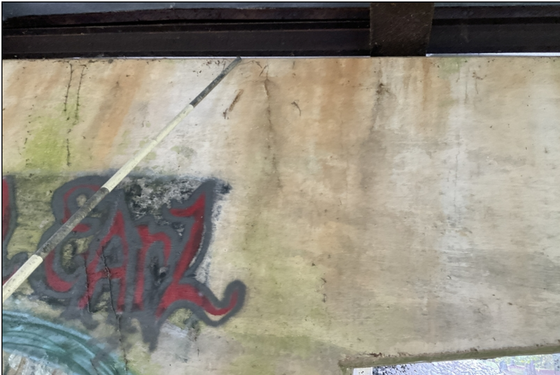
Bent 3 cap ahead face crack and crack with efflorescence.
