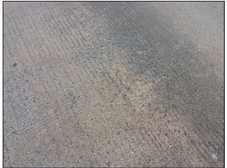
Span 1, map cracking.
