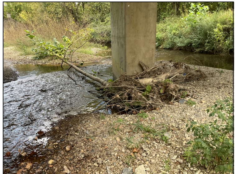
Tree and debris against column at bent 2.
