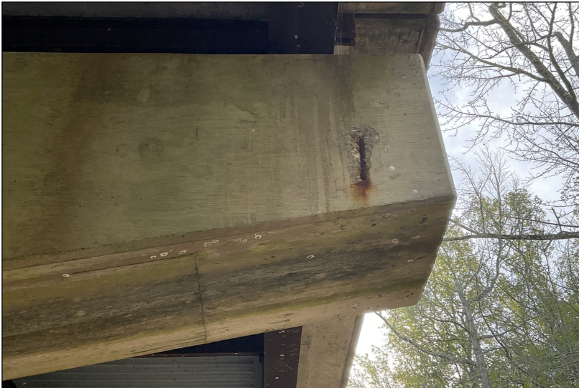
Bent 2 cap left side ahead face spall with exposed rebar.
