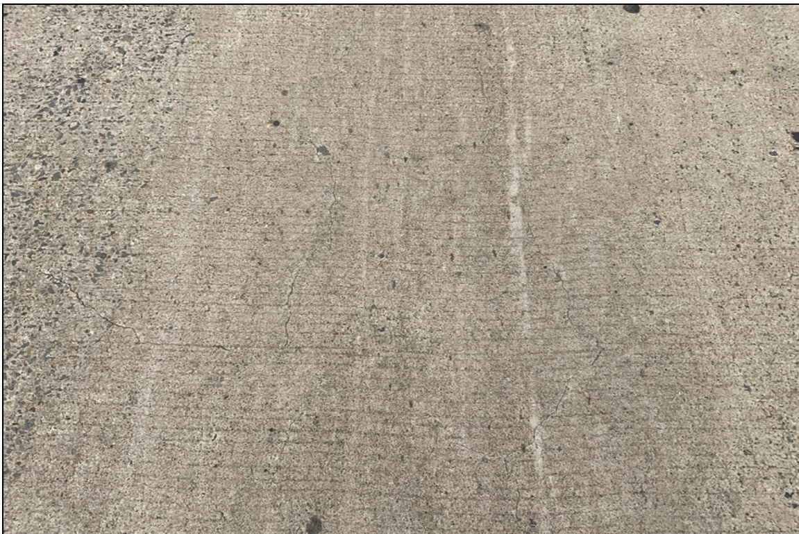
Span 2 longitudinal cracks.
