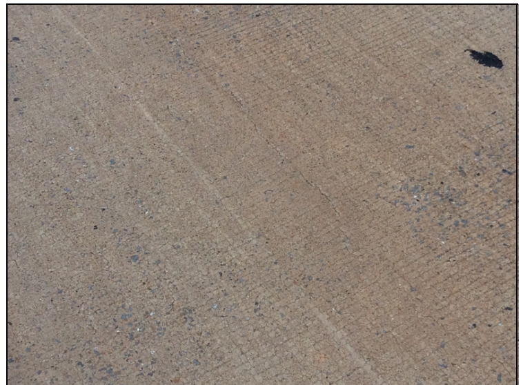
Deck cracks
