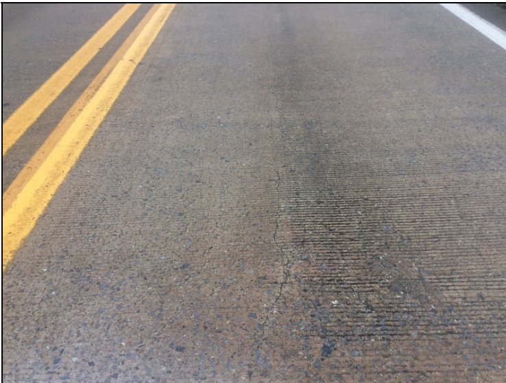
Span 1, longitudinal cracks.
