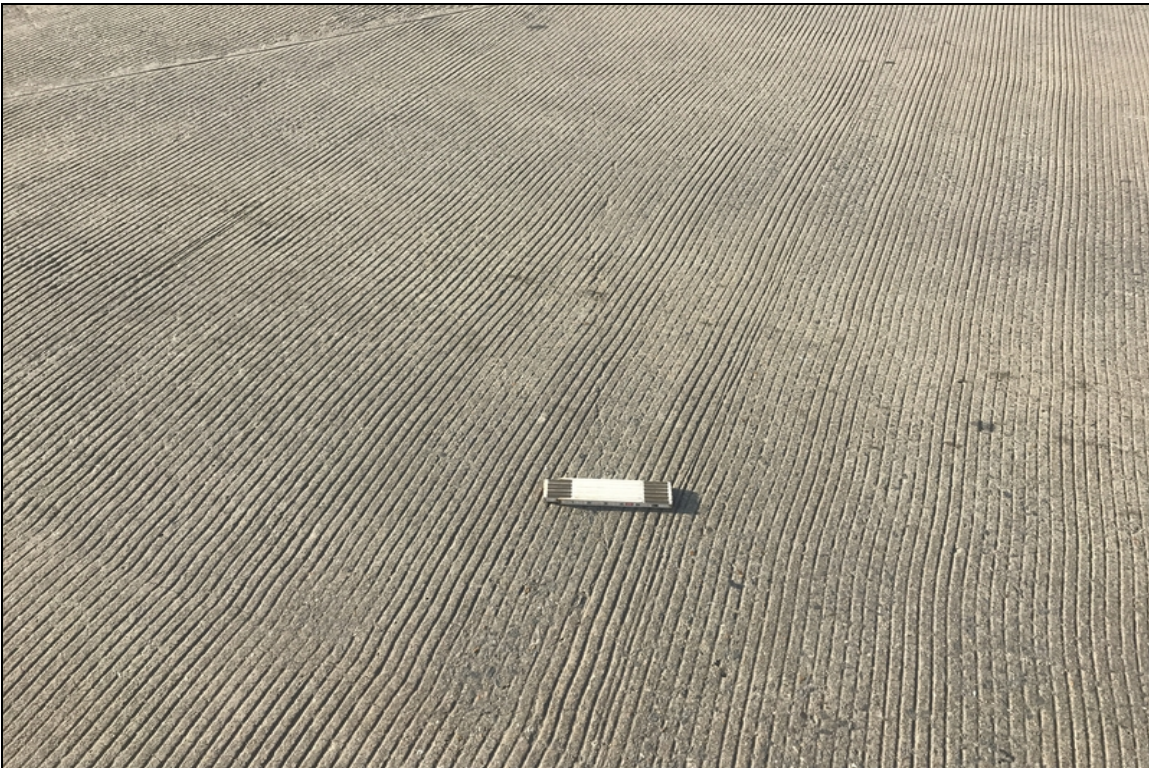
Transverse deck crack, 0.015".
