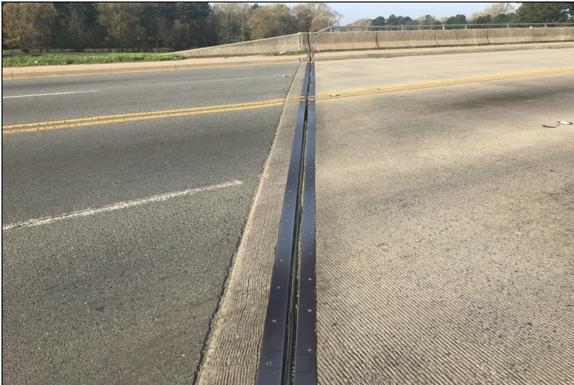
Joint seal at bent 6 debris impaction & loss of adhesion.
