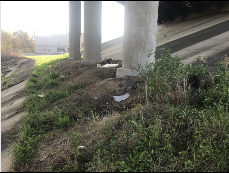
Erosion around columns 2,3 and 4 at bent 5.
