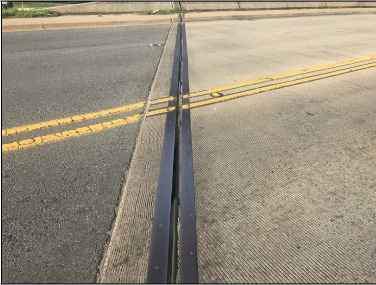
Bent 6 joint seal has lost adhesion & has debris impaction.
